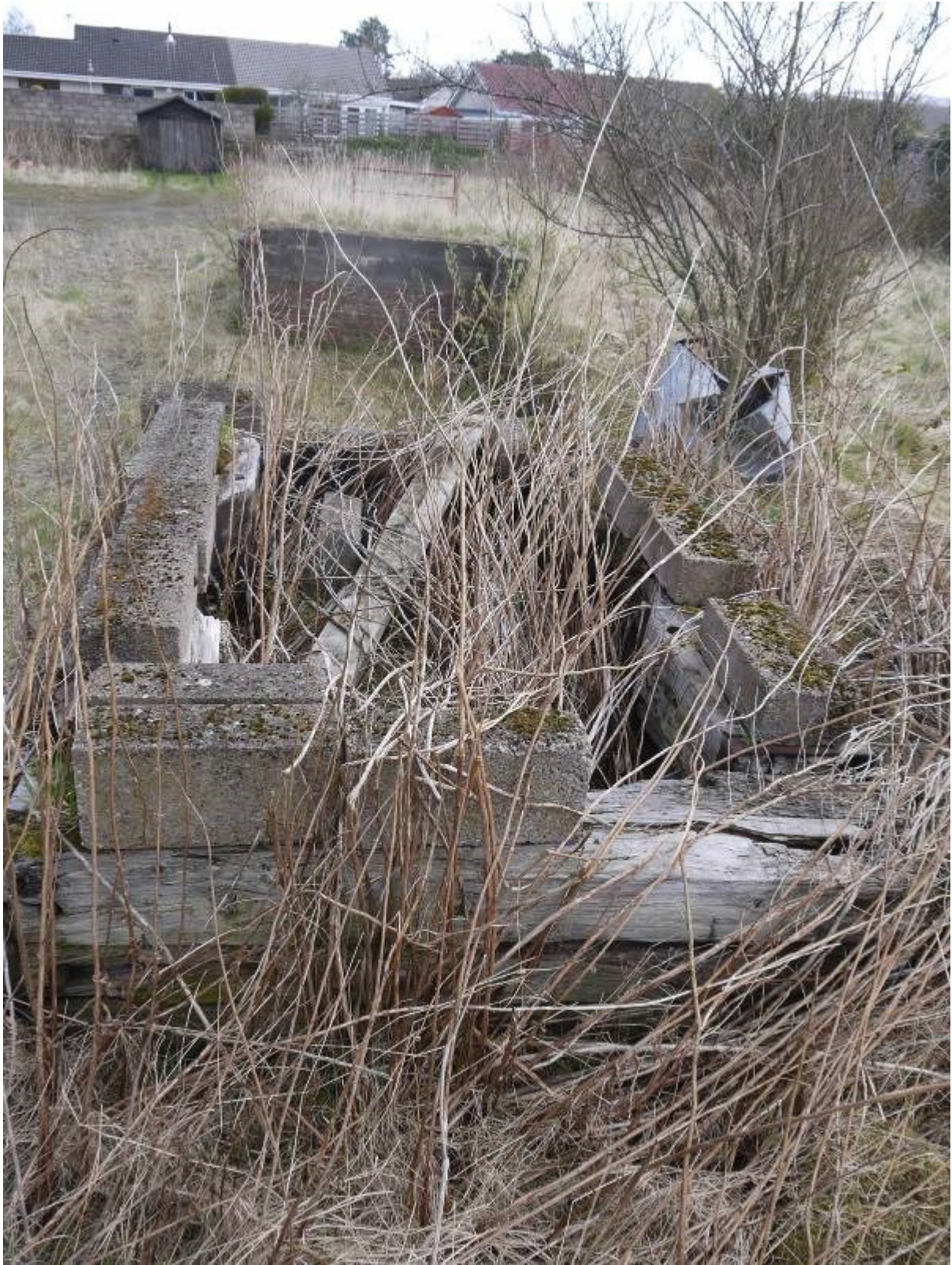
Illustration 29 Detail of structure on top of loading bay (Building C) built of sleepers and loose bricks looking east
