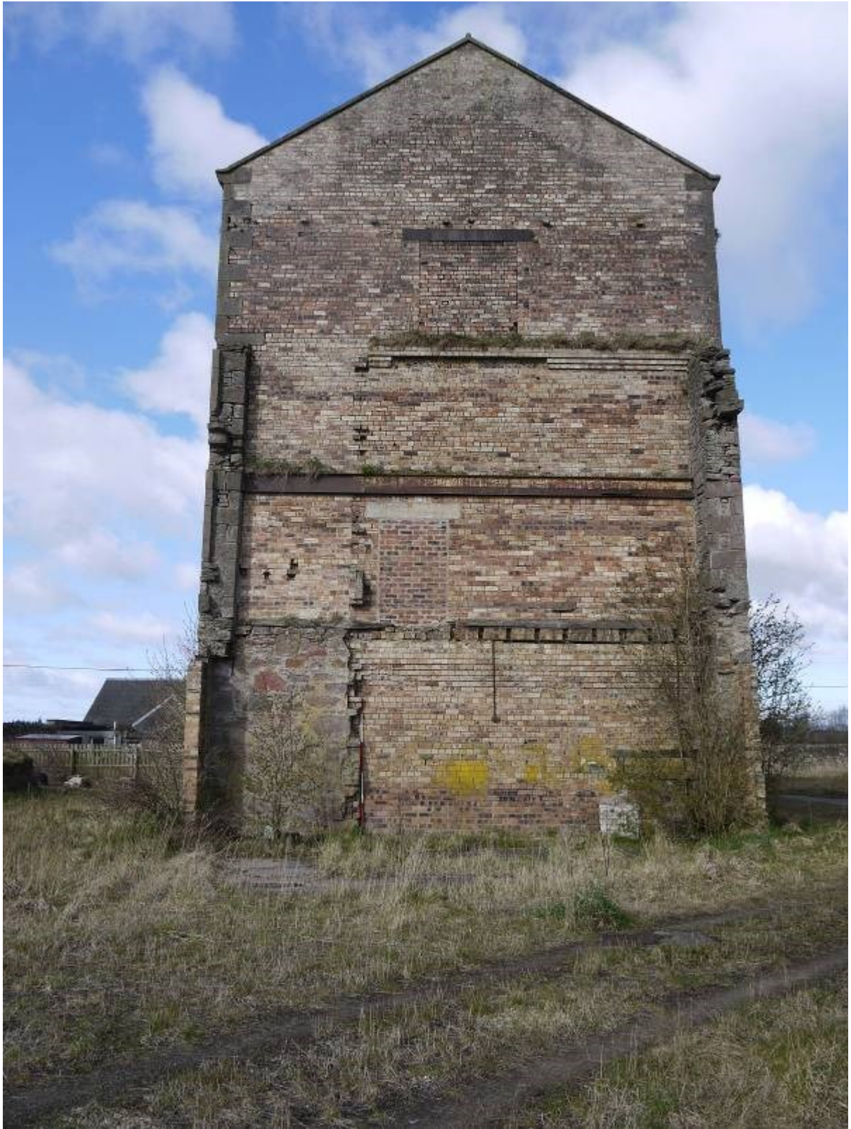
Illustration 10 eastern elevation of Building A
