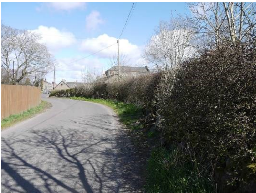
Pleasance Road Tannery buildings from the south
