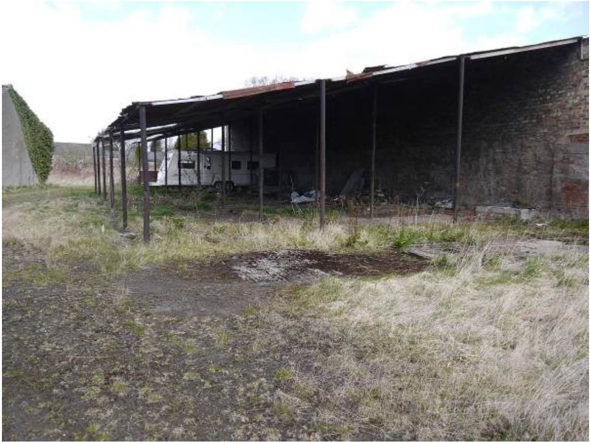
Illustration 30 Building D looking north
