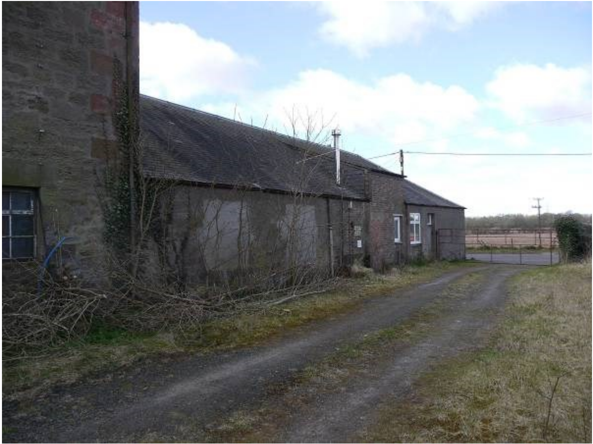
Illustration 24 north facing elevation of Building B looking west
