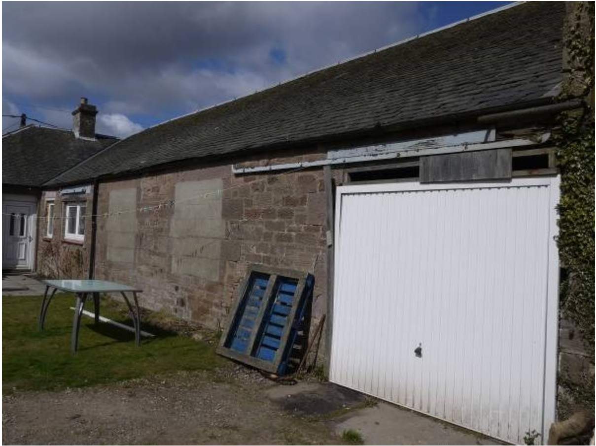
Illustration 25 south facing elevation of Building B looking north west
