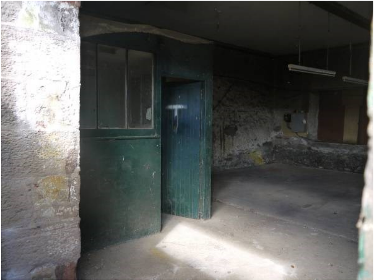
Illustration 16 Ground floor of Building A accessible from south showing office building
