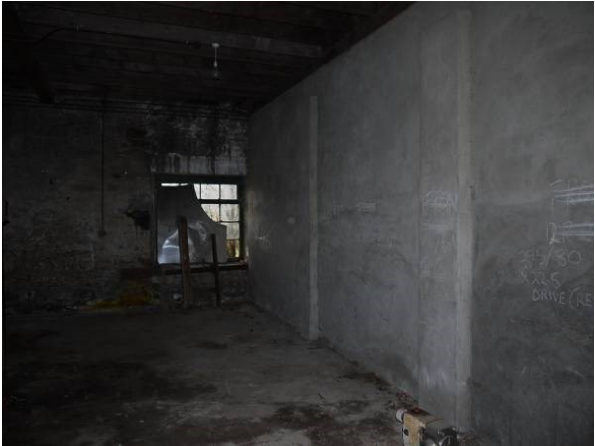
Illustration 14 western side of ground floor of Building A accessible from north
