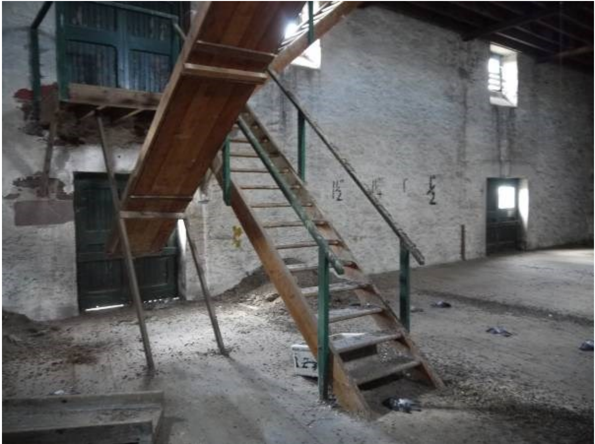
Illustration 18 steps to top floor level on first floor of Building A, chute from top floor also visible
