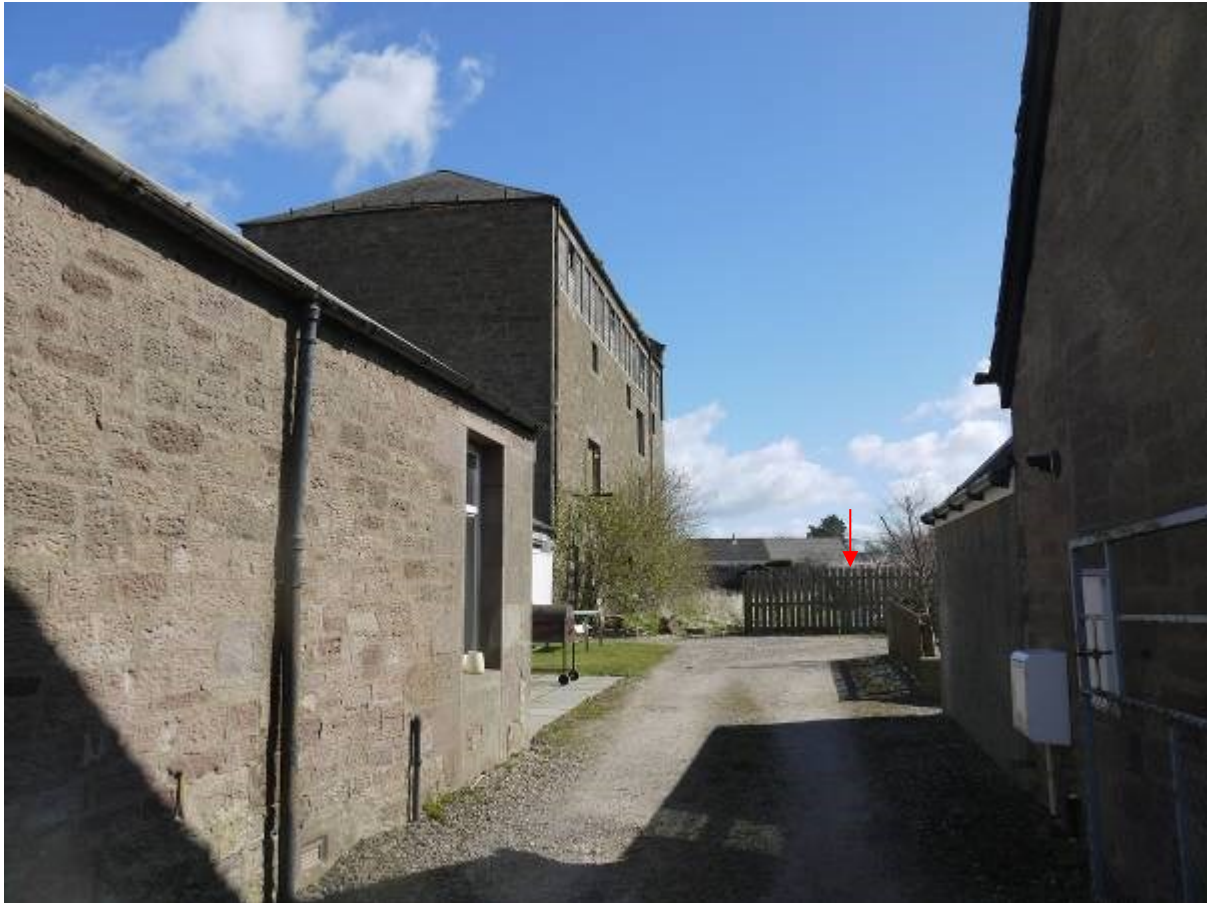
Illustration 6 General view of southern sides of Buildings B and A and location of Building C (at red arrow) looking east
