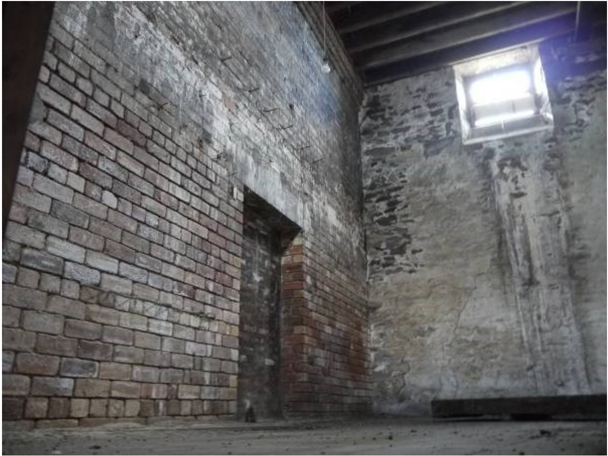
Illustration 17 eastern end of first floor level of Building A
