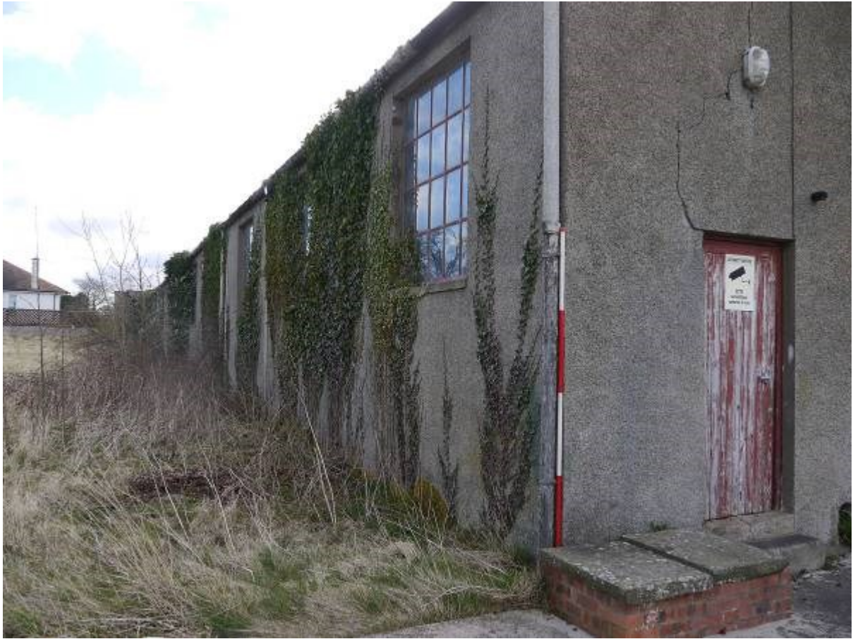
Illustration 33 northern elevation of Building E looking east
