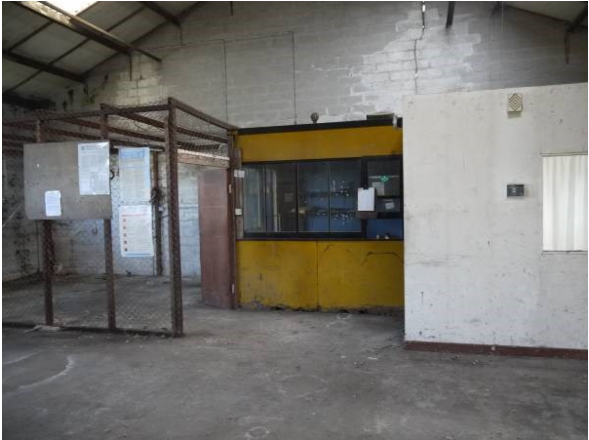
Illustration 35 Former office buildings at eastern end of Building E
