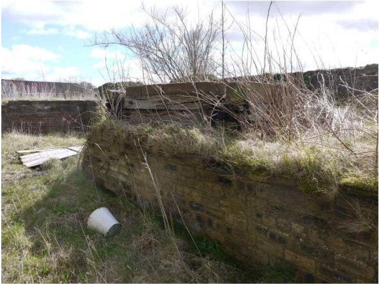
Illustration 28 View of sleeper built structure in Building C looking south east
