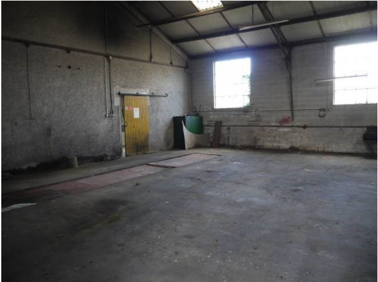
Illustration 36 interior of eastern end of Building E looking north
