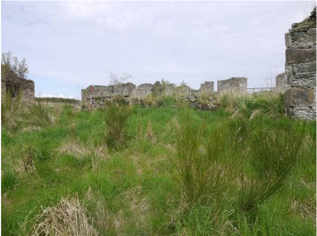
Illustration 28 Southern elevation of Building D looking north
