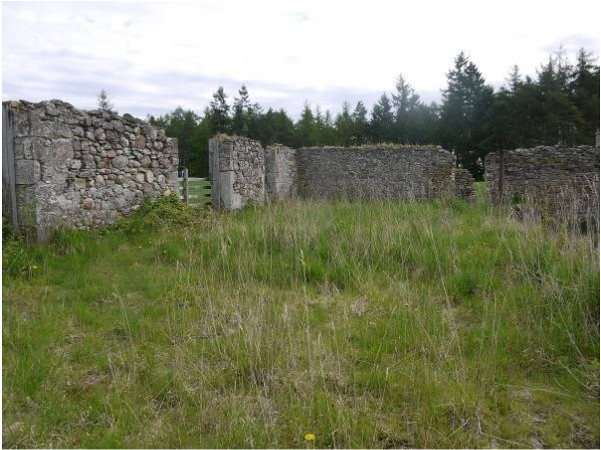
Illustration 24 Interior of Building C looking east
