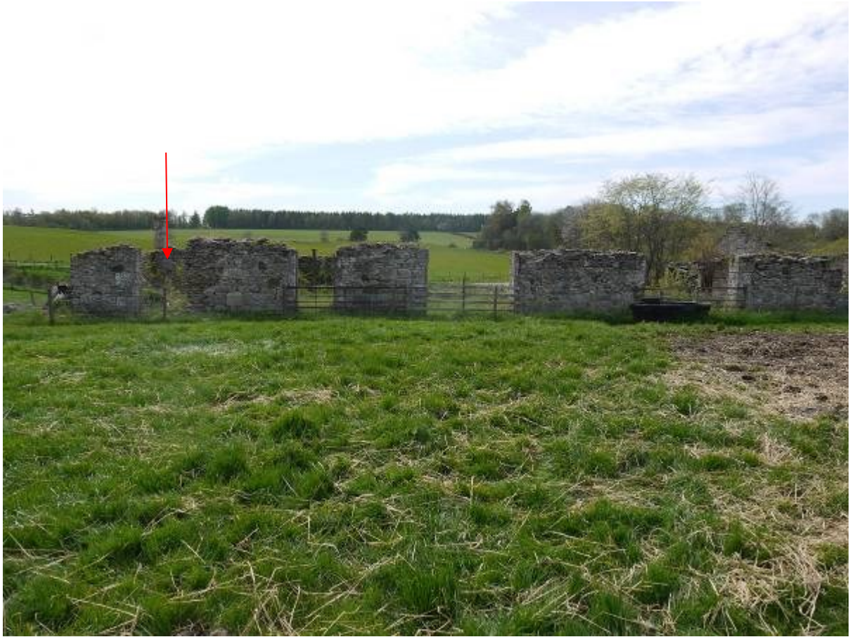
Illustration 32 Northern elevations of Buildings C and E (marked with red arrow)
