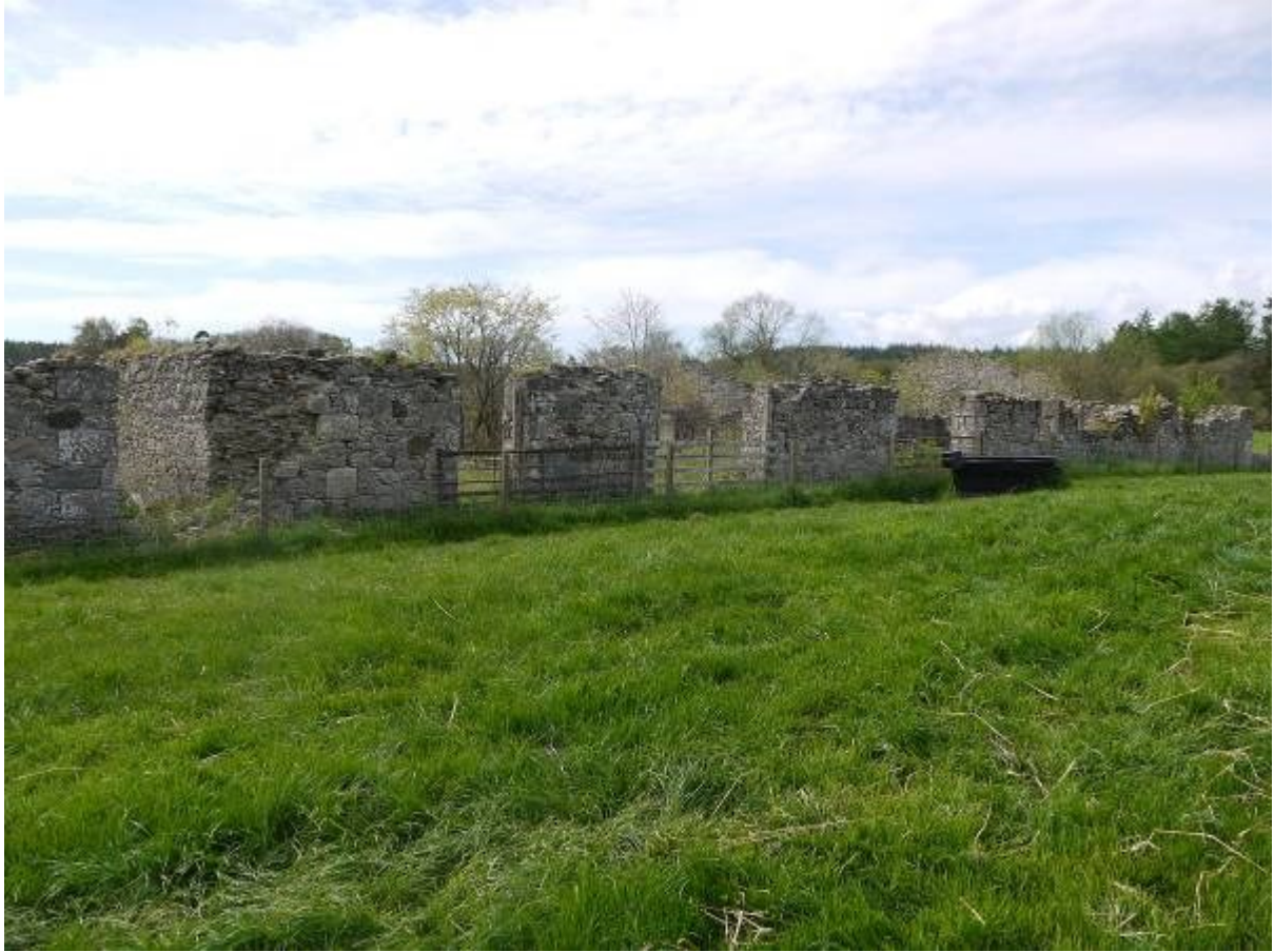
Illustration 25 Northern elevation of Building C looking south west
