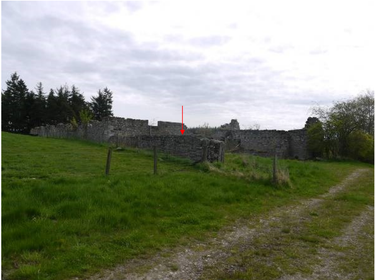
Illustration 20 Building complex looking south east, red arrow indicates wall line described in text
