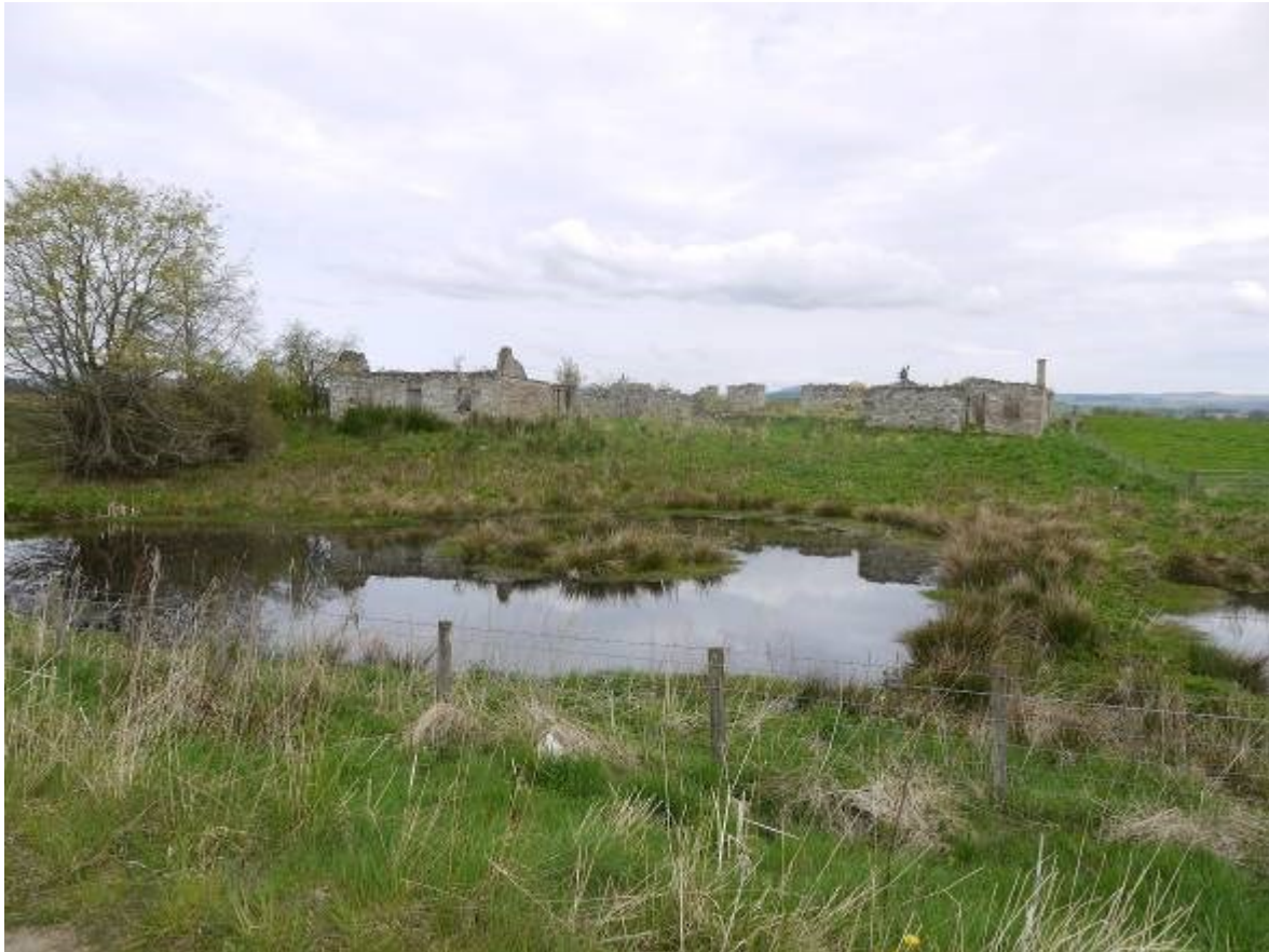
Group of derelict buildings at Old England from the south
