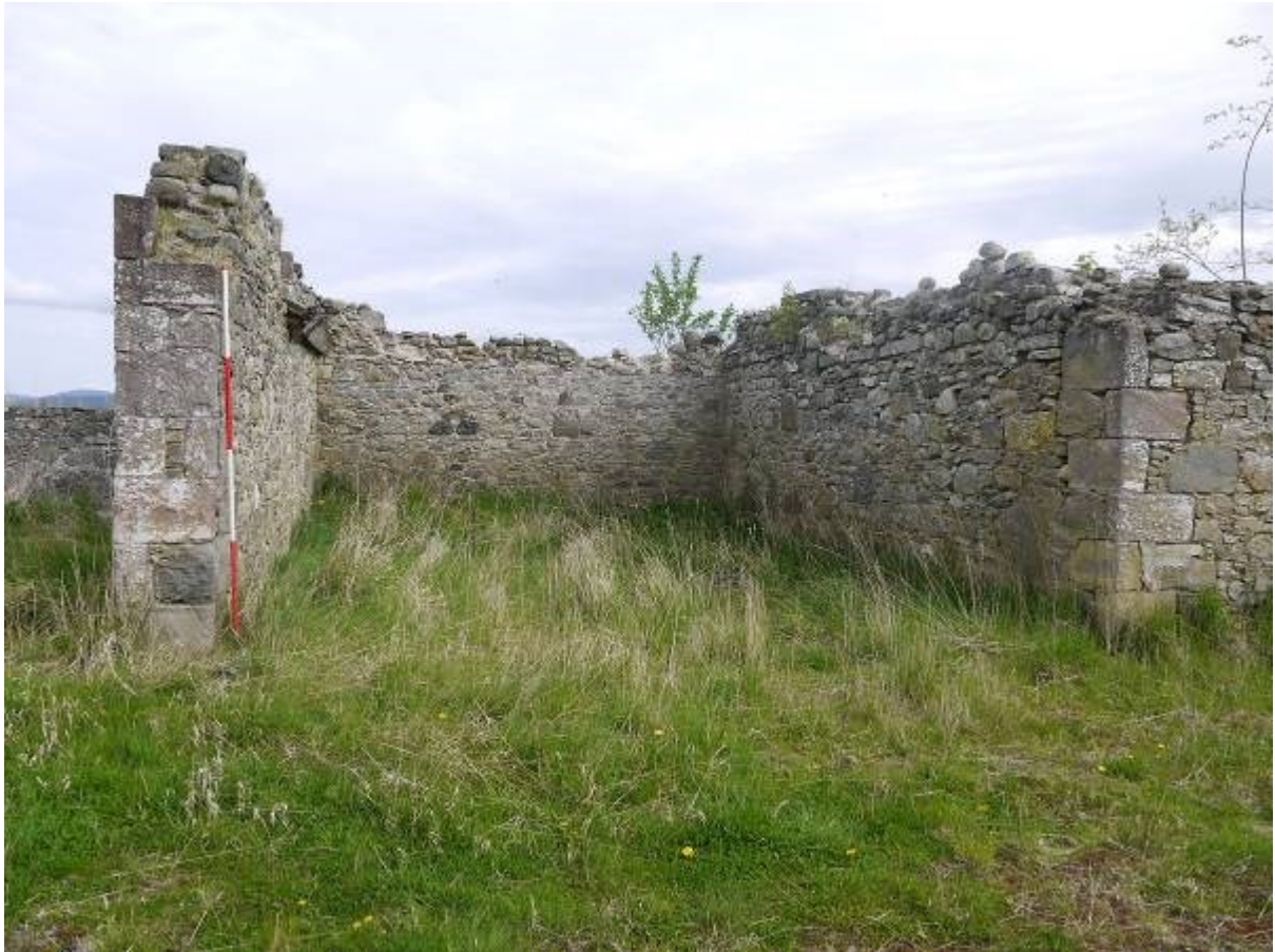
Illustration 21 Building B looking north
