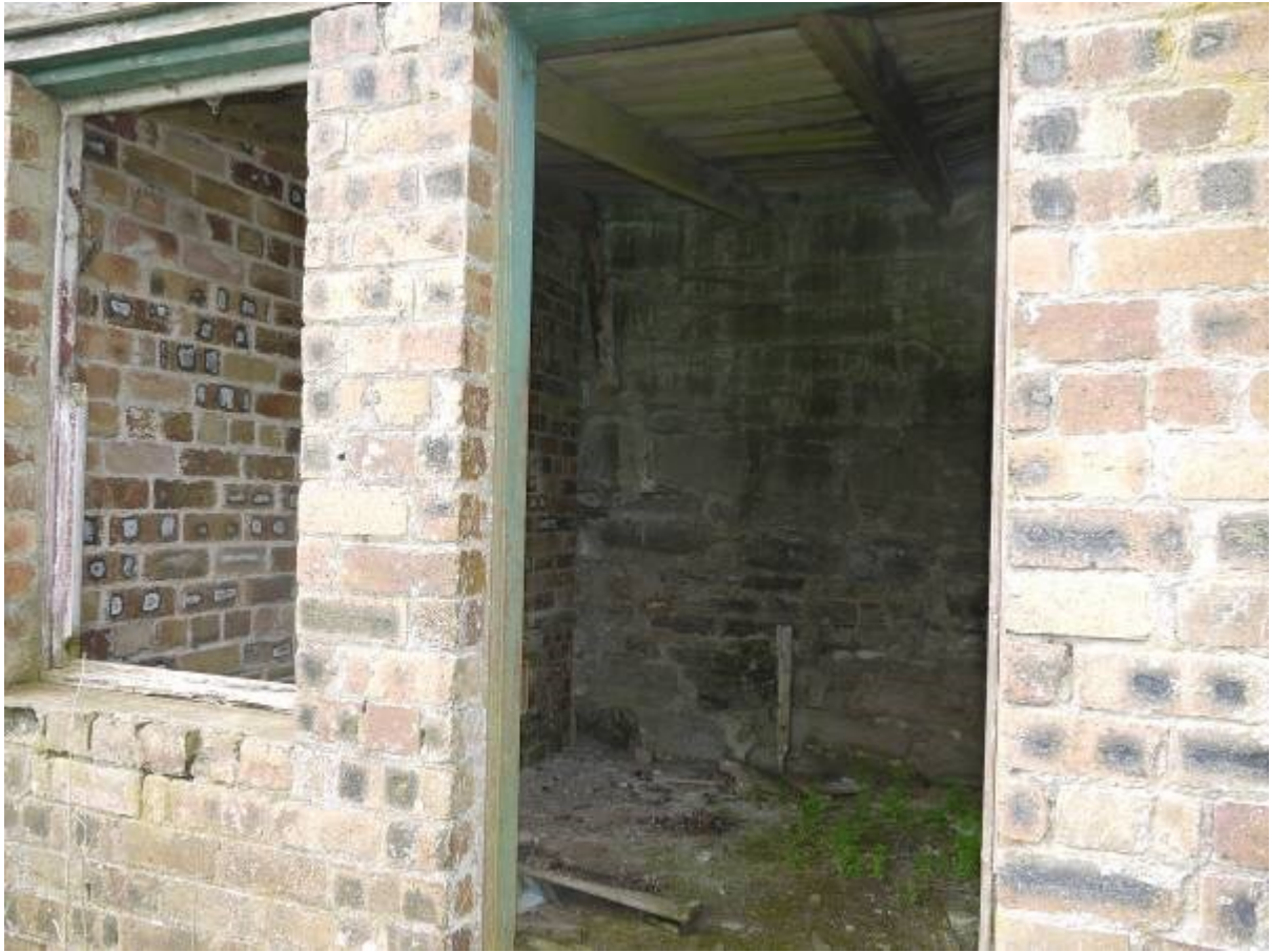
Illustration 17 Interior of room at southern end of brick extension
