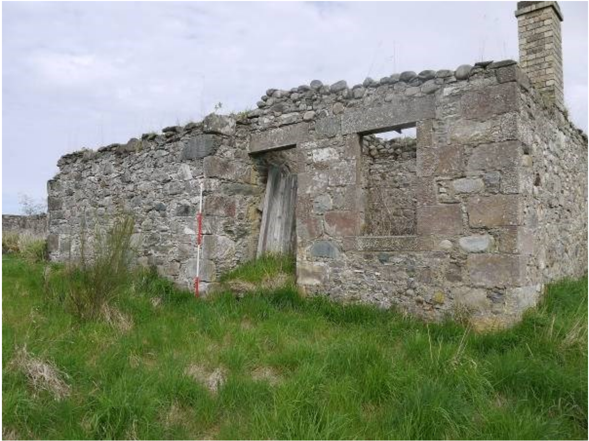
Illustration 30 Southern elevation of buildings D and E looking north
