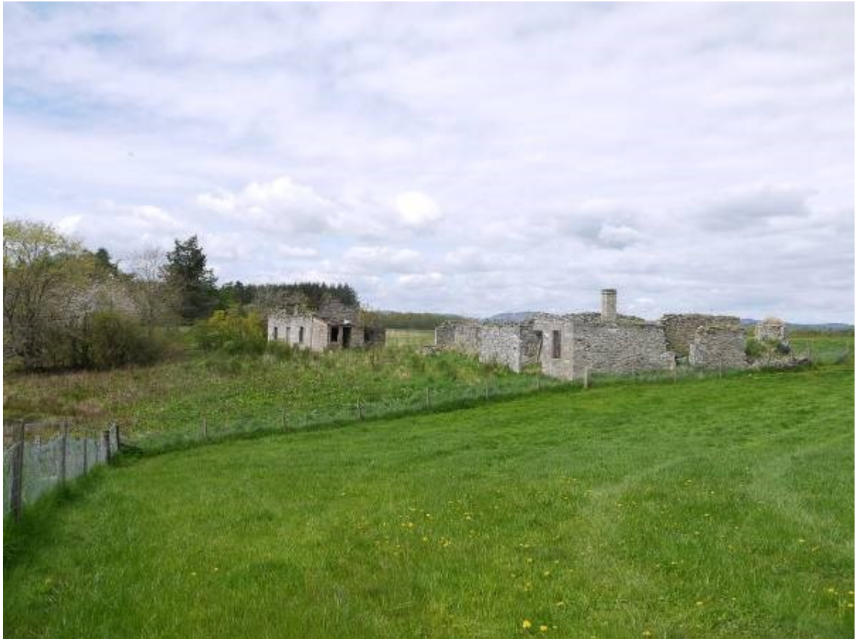
Illustration 5 Derelict buildings at Old England looking North West
