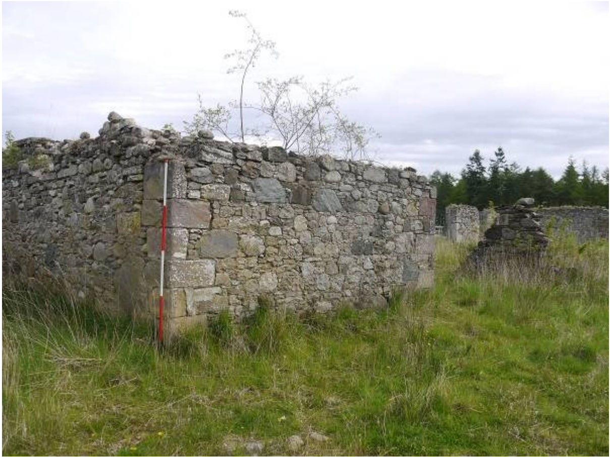
Illustration 22 Southern elevation of Building C looking north east
