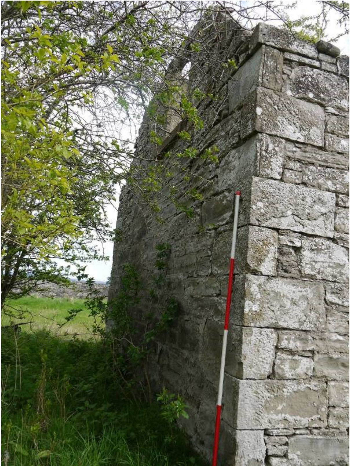
Illustration 9 Western elevation of Building A looking north
