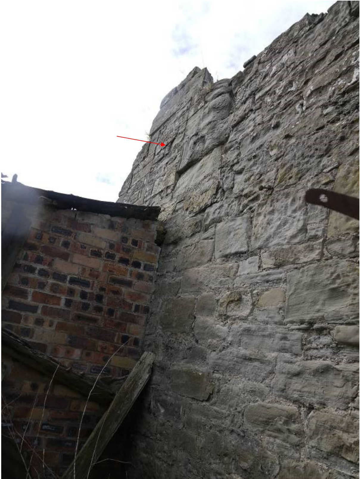
Illustration 19 View of interior of brick extension showing junction with eastern wall of farmhouse and blocked window (red arrow)
