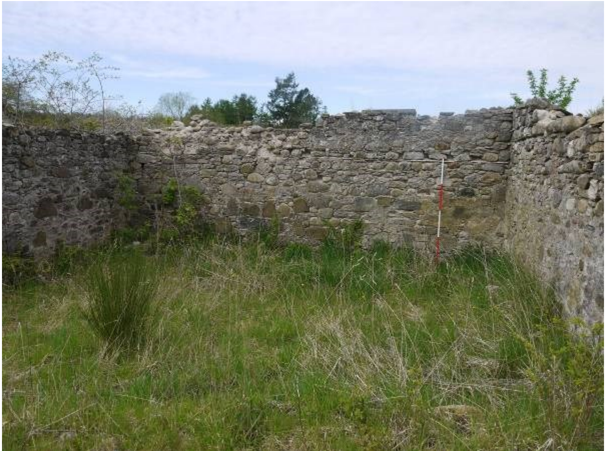
Illustration 23 Interior of western end of Building C looking west
