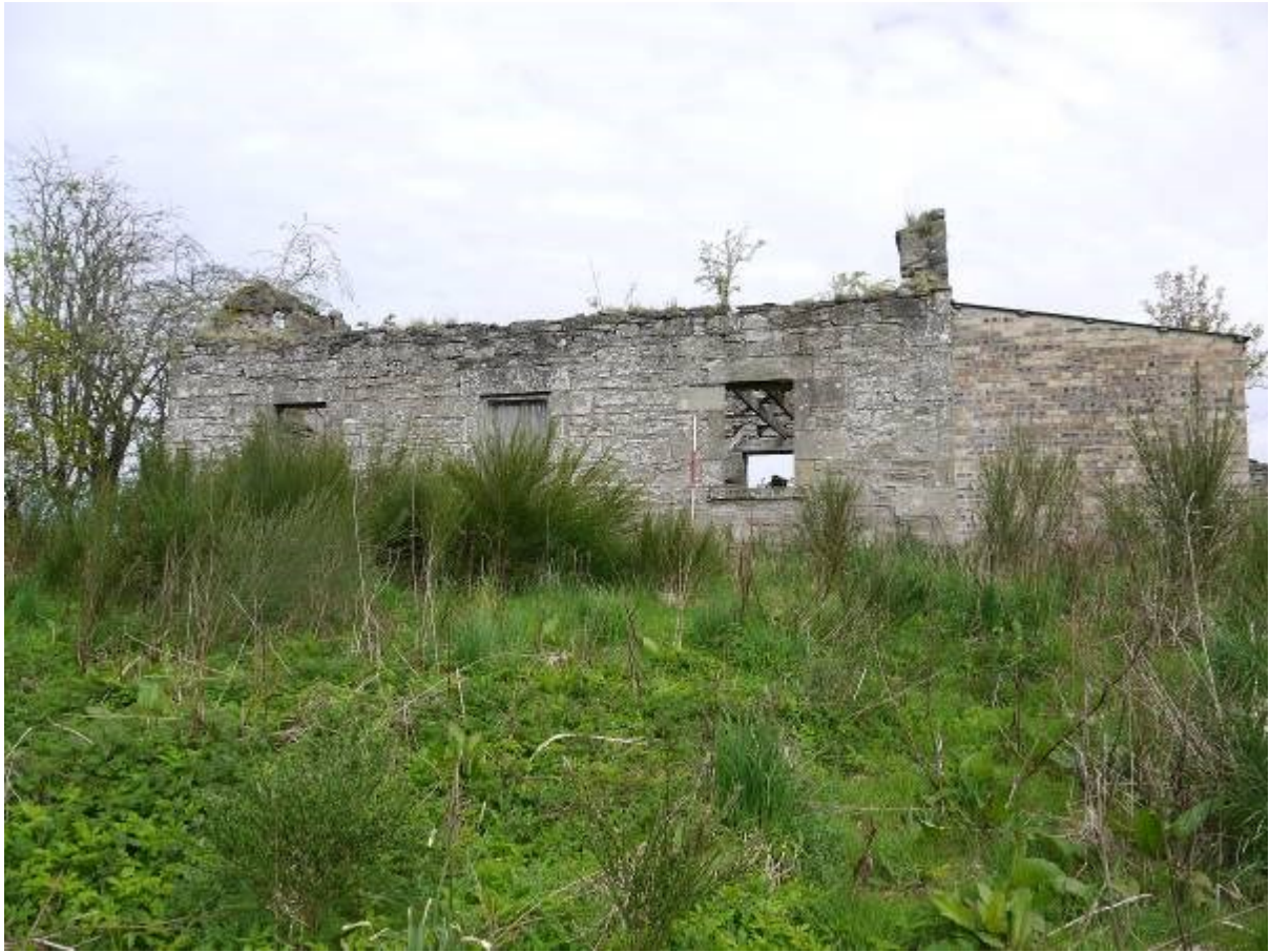
Illustration 10 Southern elevation of Building A looking north
