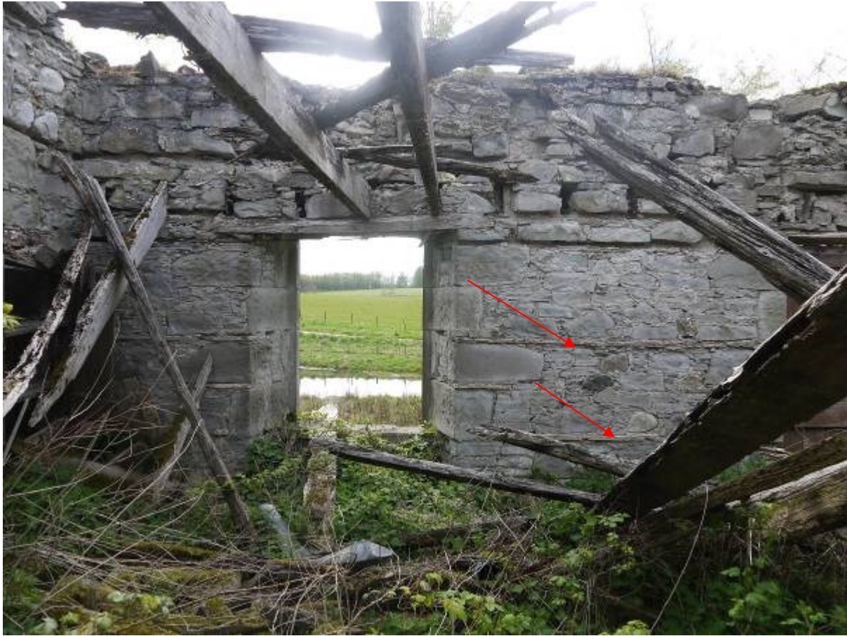
Illustration 13 Internal northern elevation (eastern end) looking south, red arrows indicate planks built into wall face
