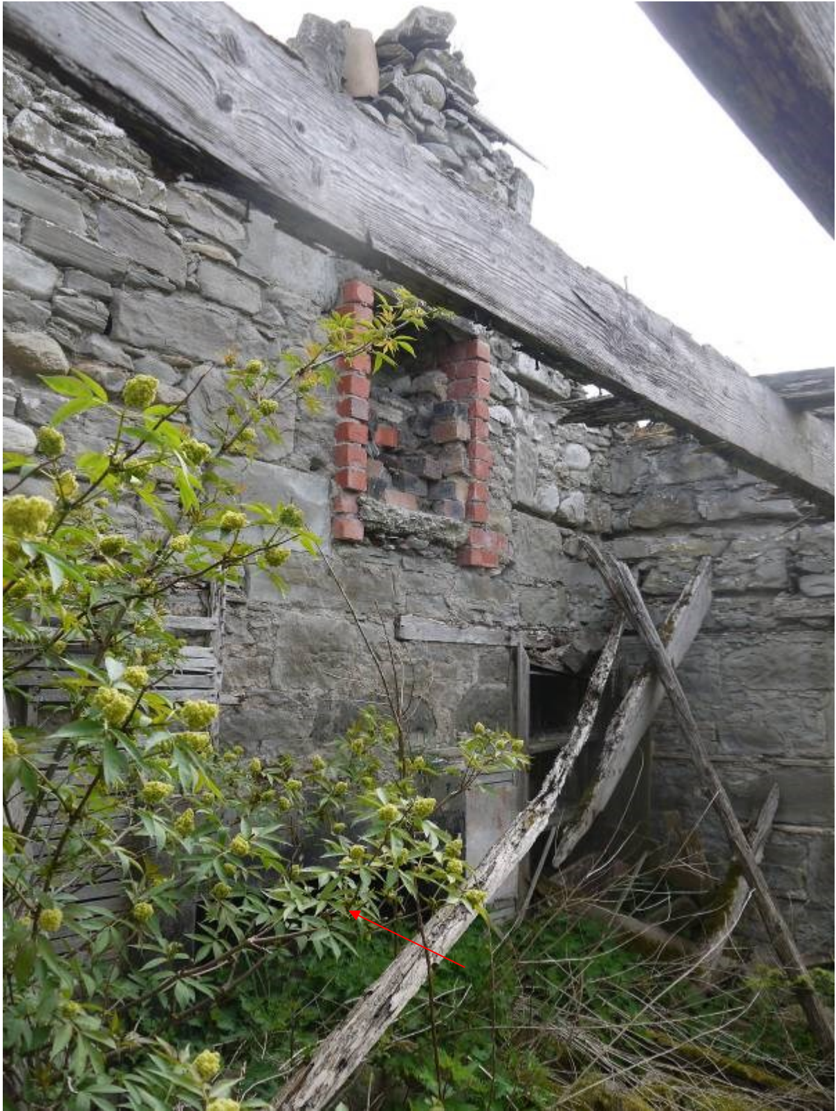
Illustration 12 Internal western elevation of Building A showing surviving wooden wall panelling, fireplace at first floor level and cupboard and fireplace at ground floor level (marked with red arrow)
