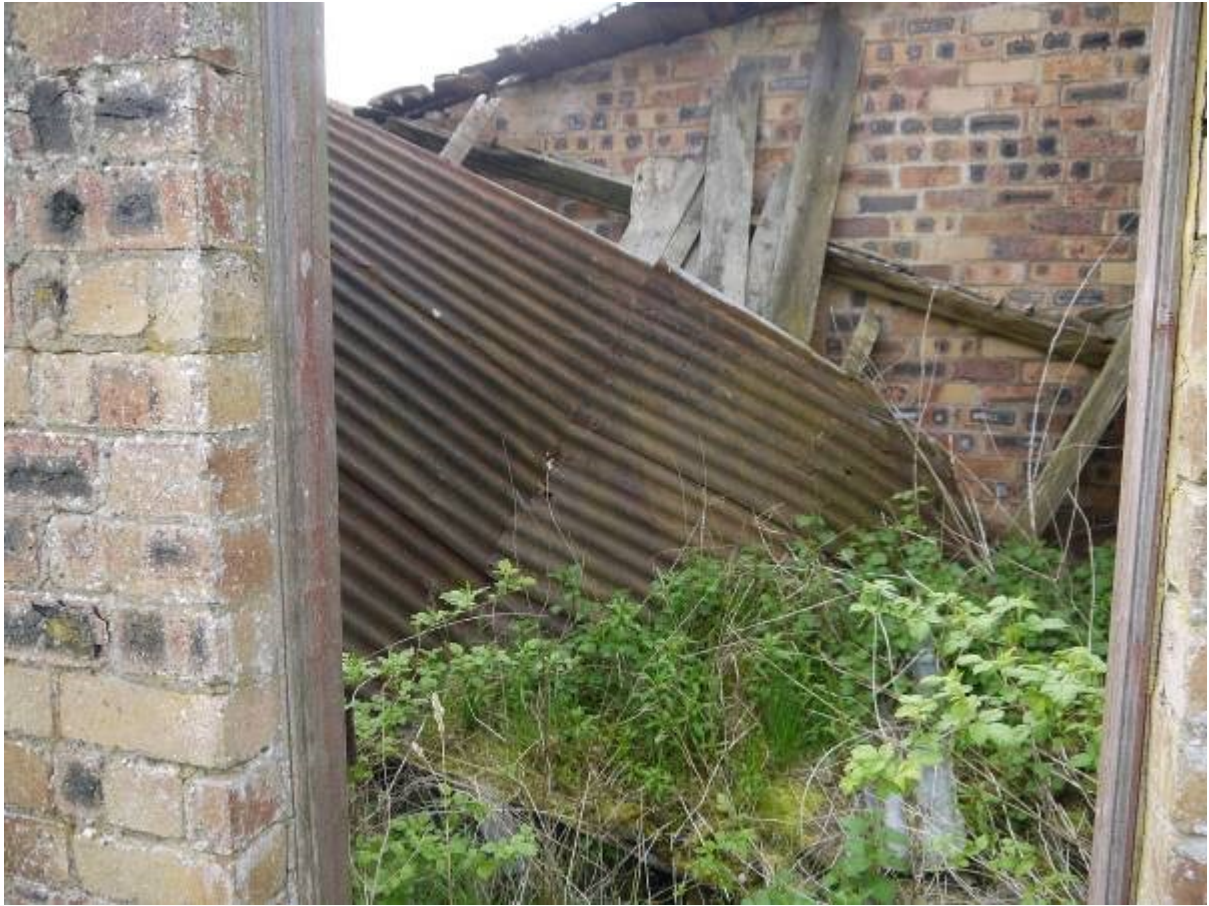
Illustration 18 Interior of northern room in brick extension
