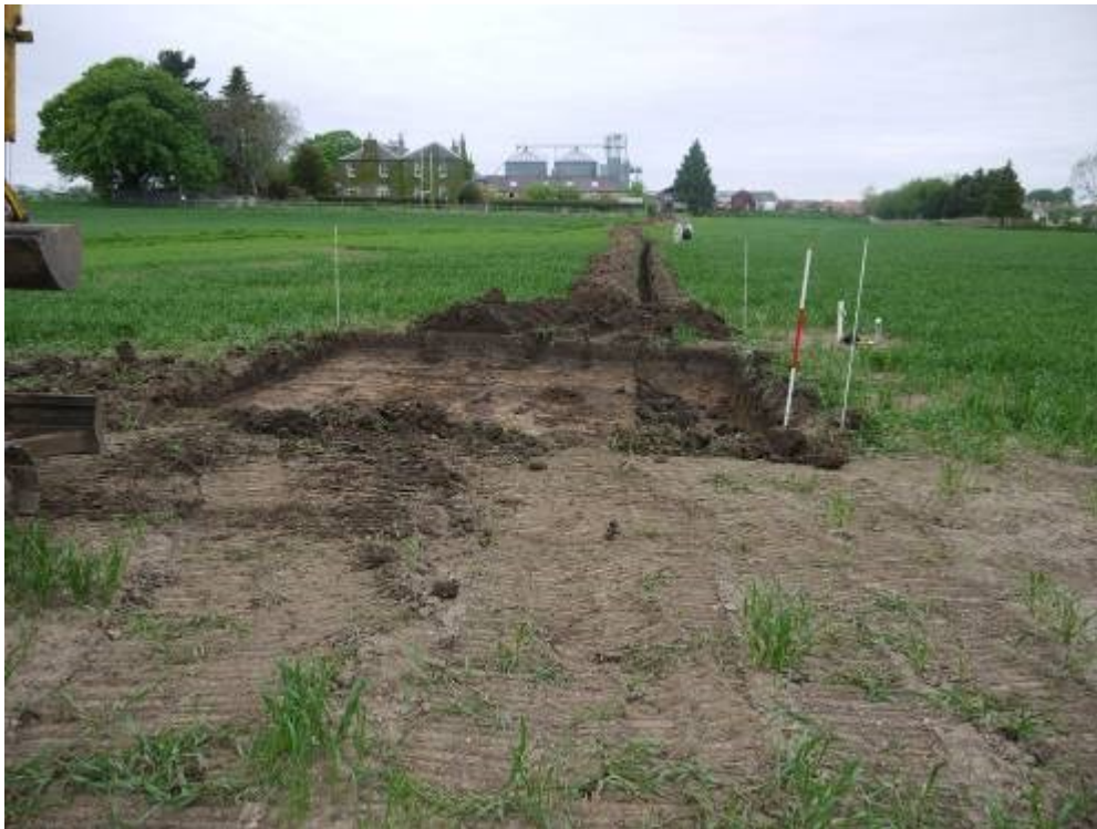
Excavated wind turbine plinth and cable trench looking North (South Elphinstone Farm in background)
