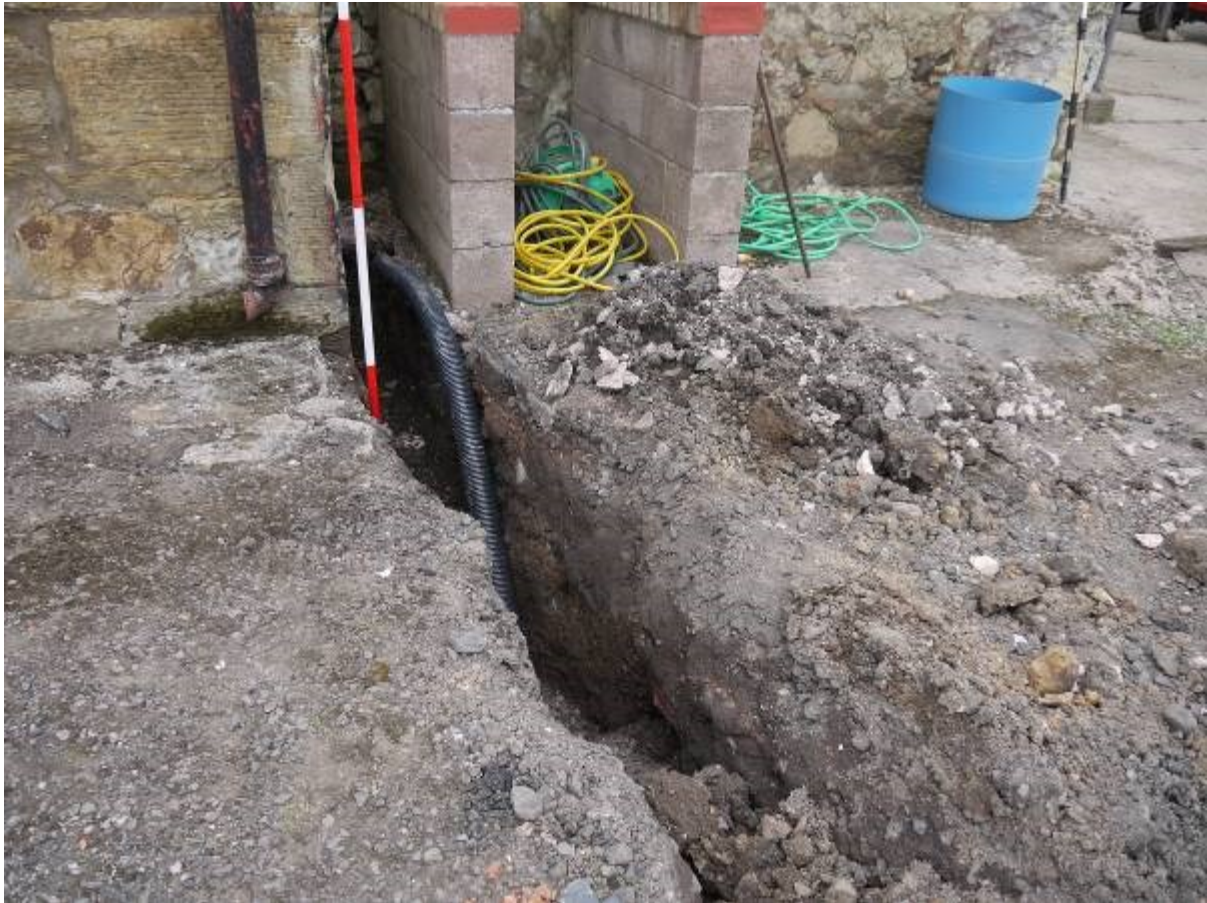
Illustration 4 Cable trench adjacent to farm steadings looking north east
