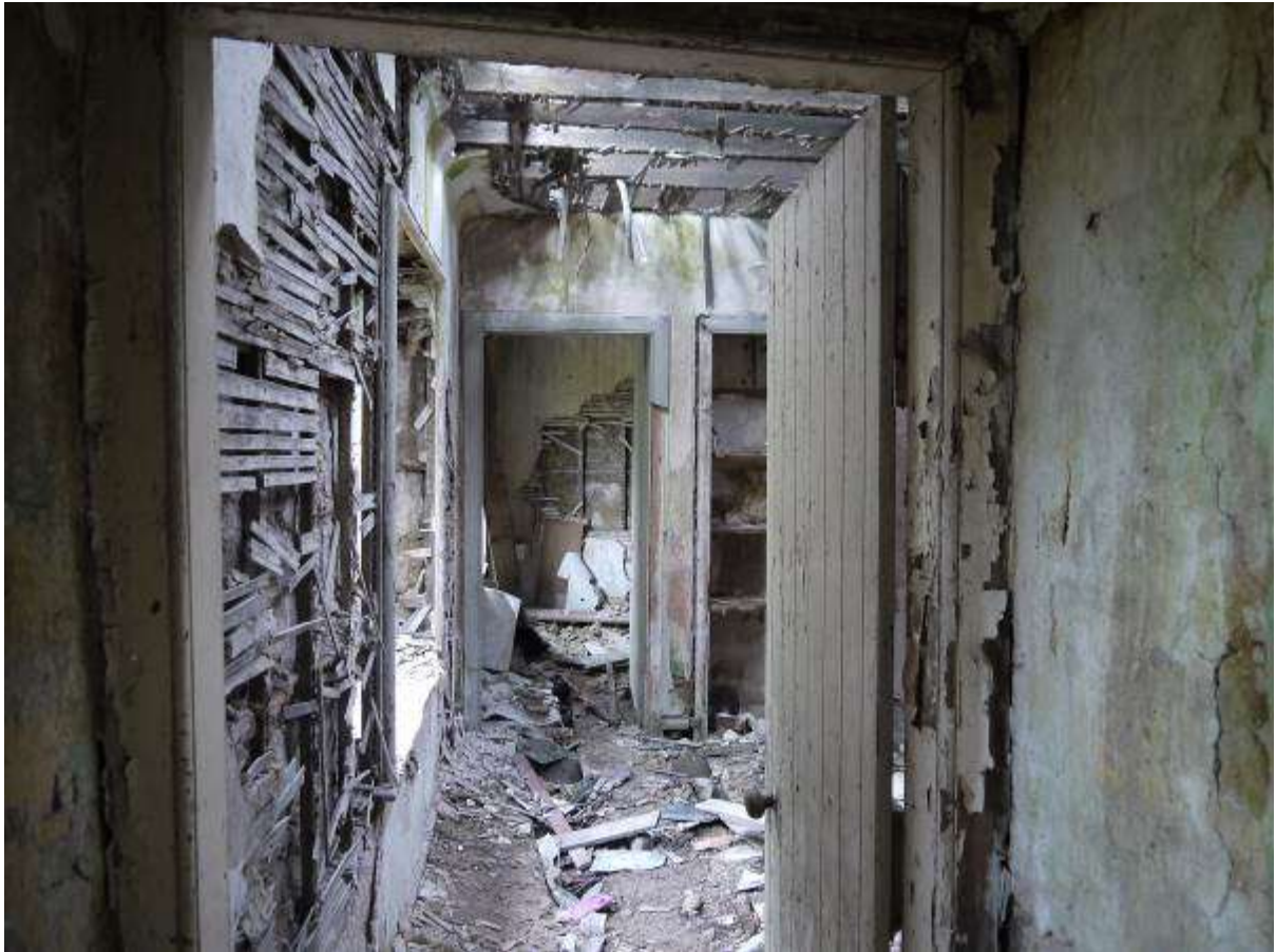
Illustration 19 Interior of Building 1 looking South West
