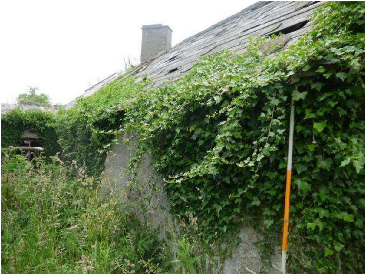
Illustration 15 North western elevation of Building 1 looking north east
