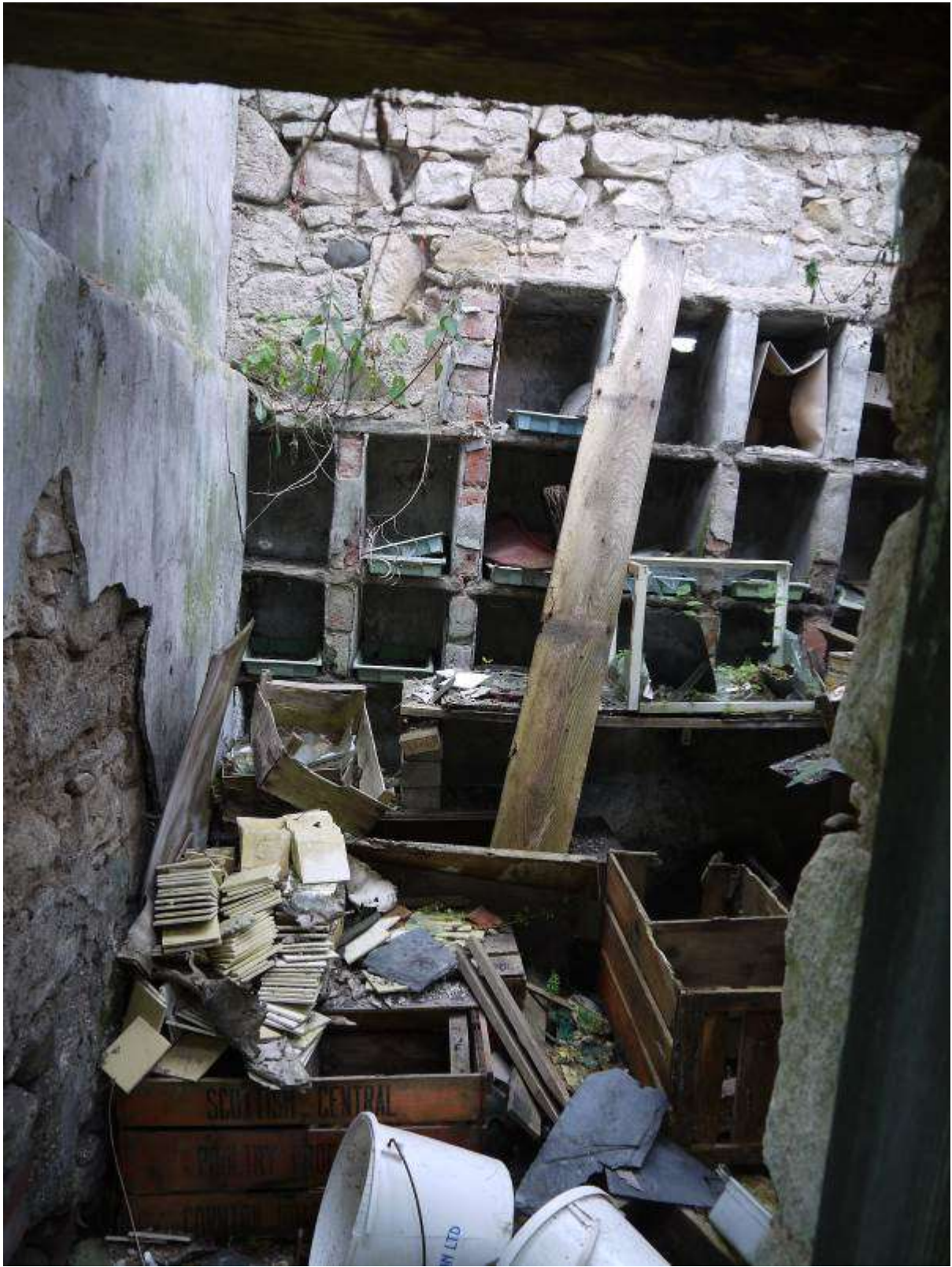
Illustration 23 Internal view of Room B in Building 3 showing stone built boxes in face of wall
