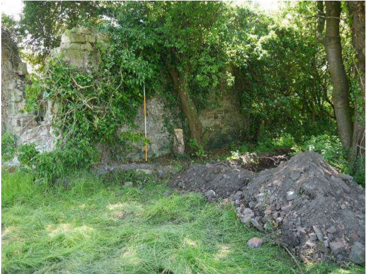
Illustration 29 External North West facing elevation of Wall J looking South East
