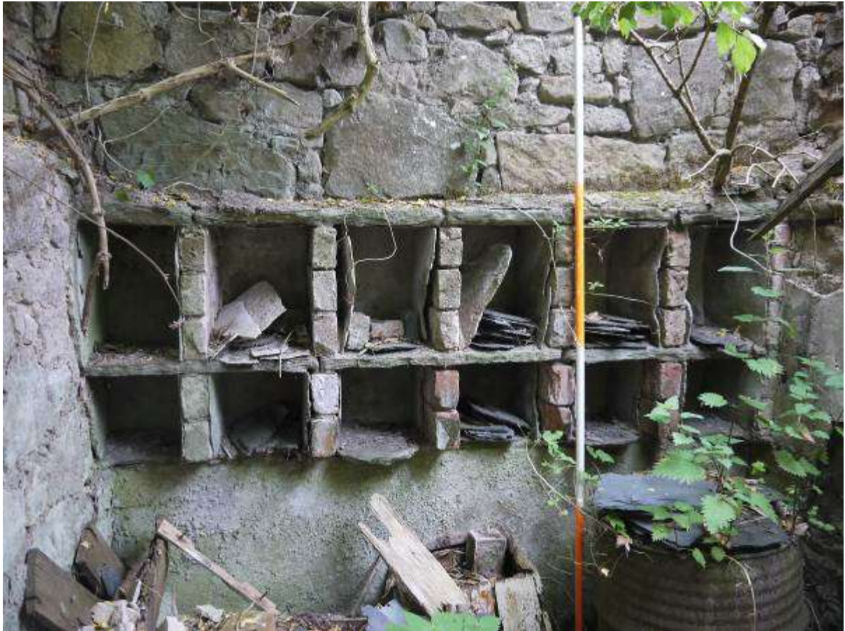
Illustration 26 Internal view of Room E in Building 3 showing stone and brick built boxes in wall face
