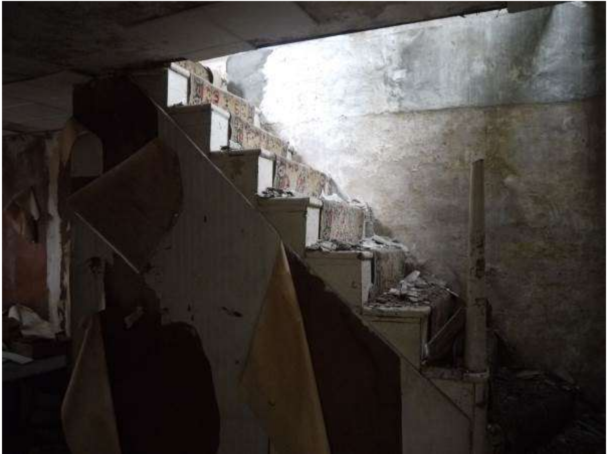
Illustration 20 staircase to attic floor level inside Building 1
