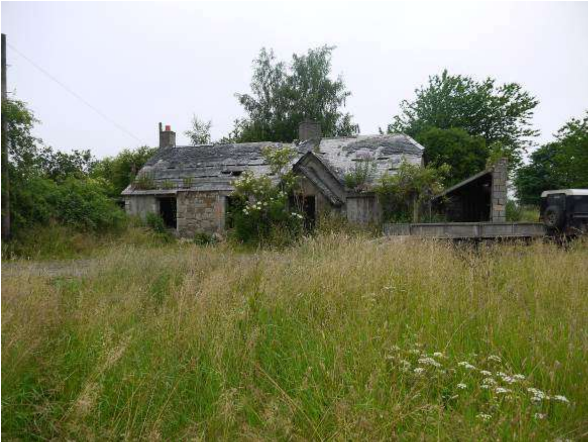
Derelict cottage, The Kennels, Lower Polmaise looking North West
