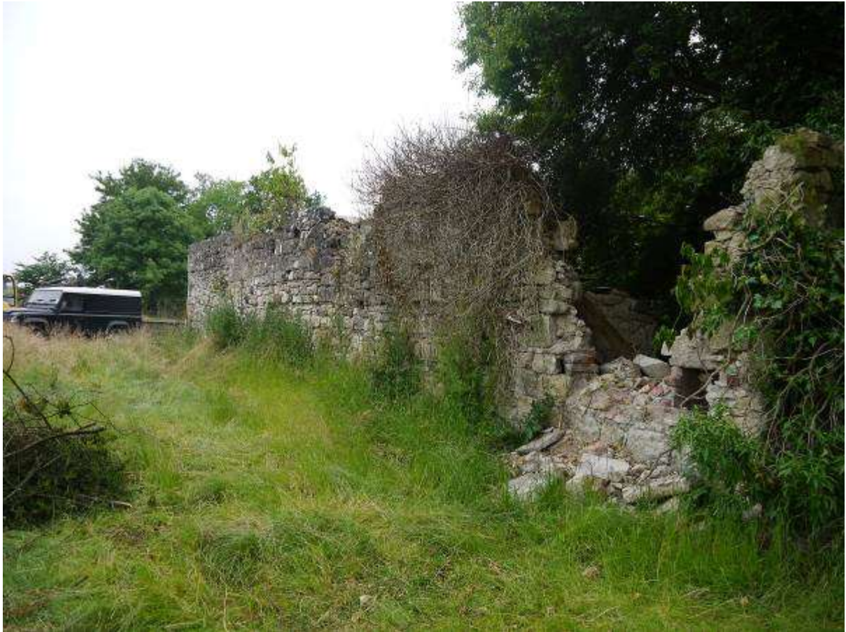
Illustration 28 North West facing external elevation of Wall H looking South East
