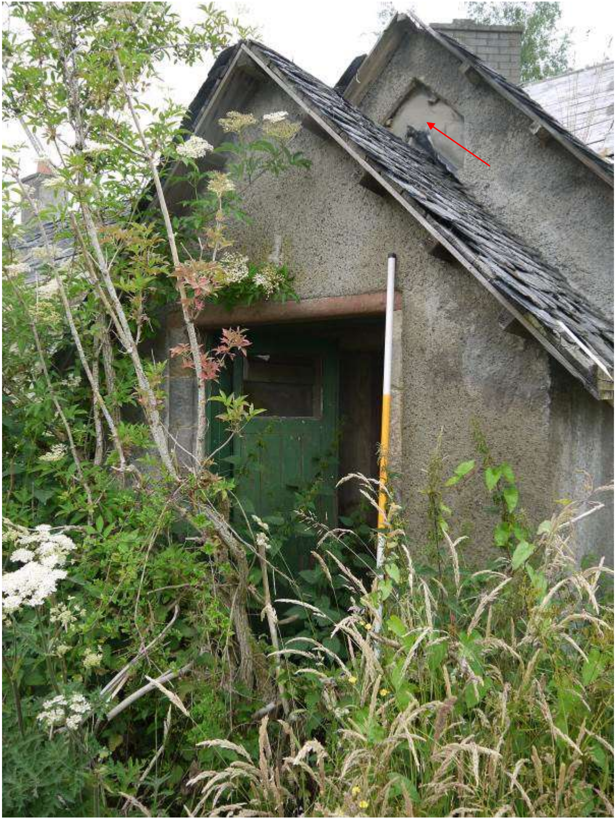
Illustration 13 Porched entrance to Building 1 with reused roll moulded doorway, possible location of date stone marked with red arrow
