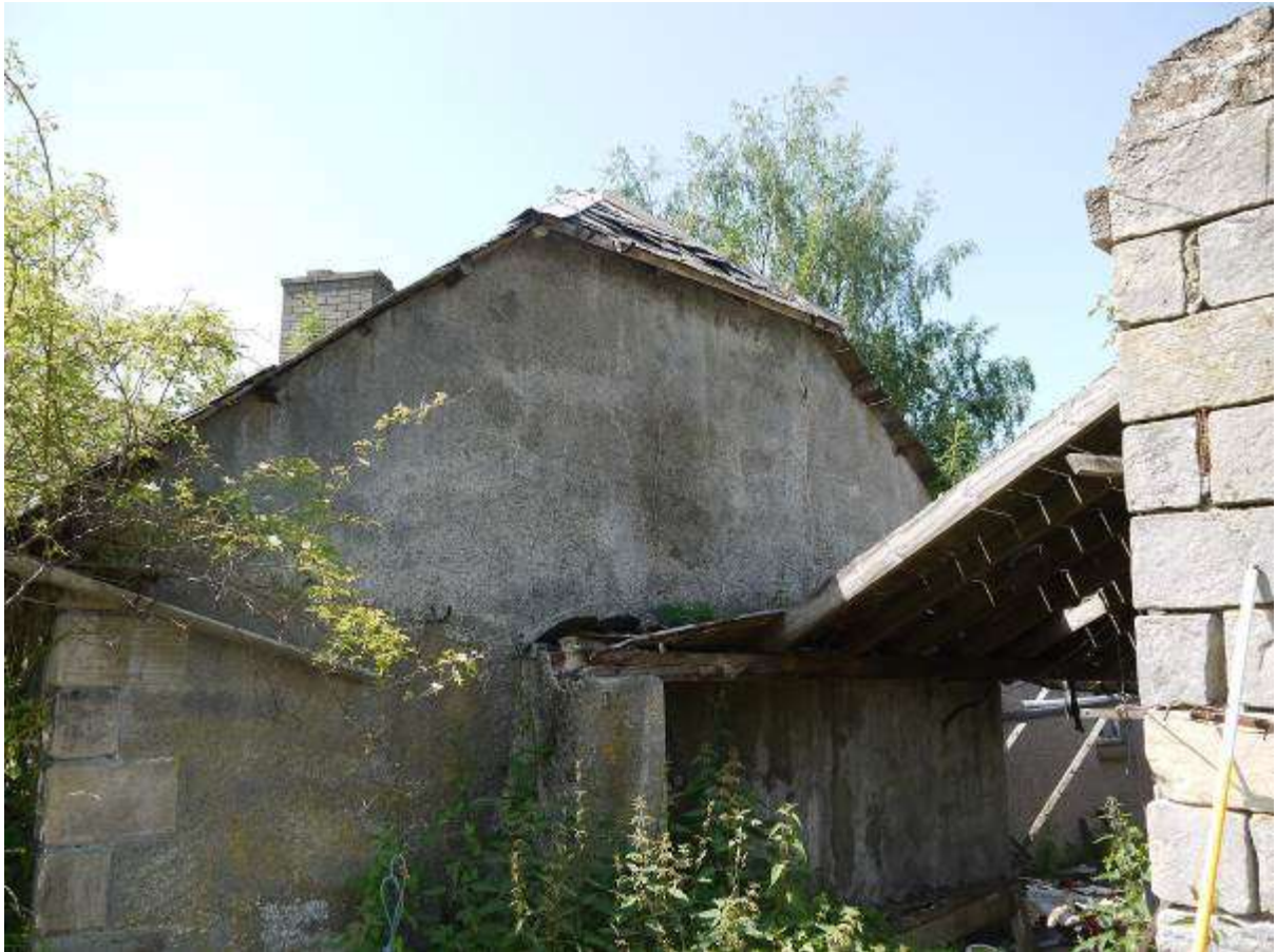
Illustration 17 North Eastern elevation of Building 1 showing angled top to gable looking south west, shaped quoins at end of Wall H visible behind scale to right of photograph
