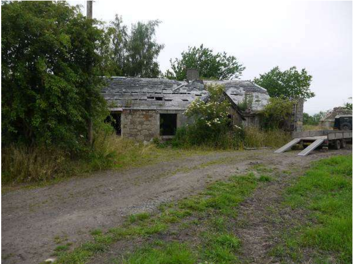
Illustration 6 General view of group of buildings looking North West
