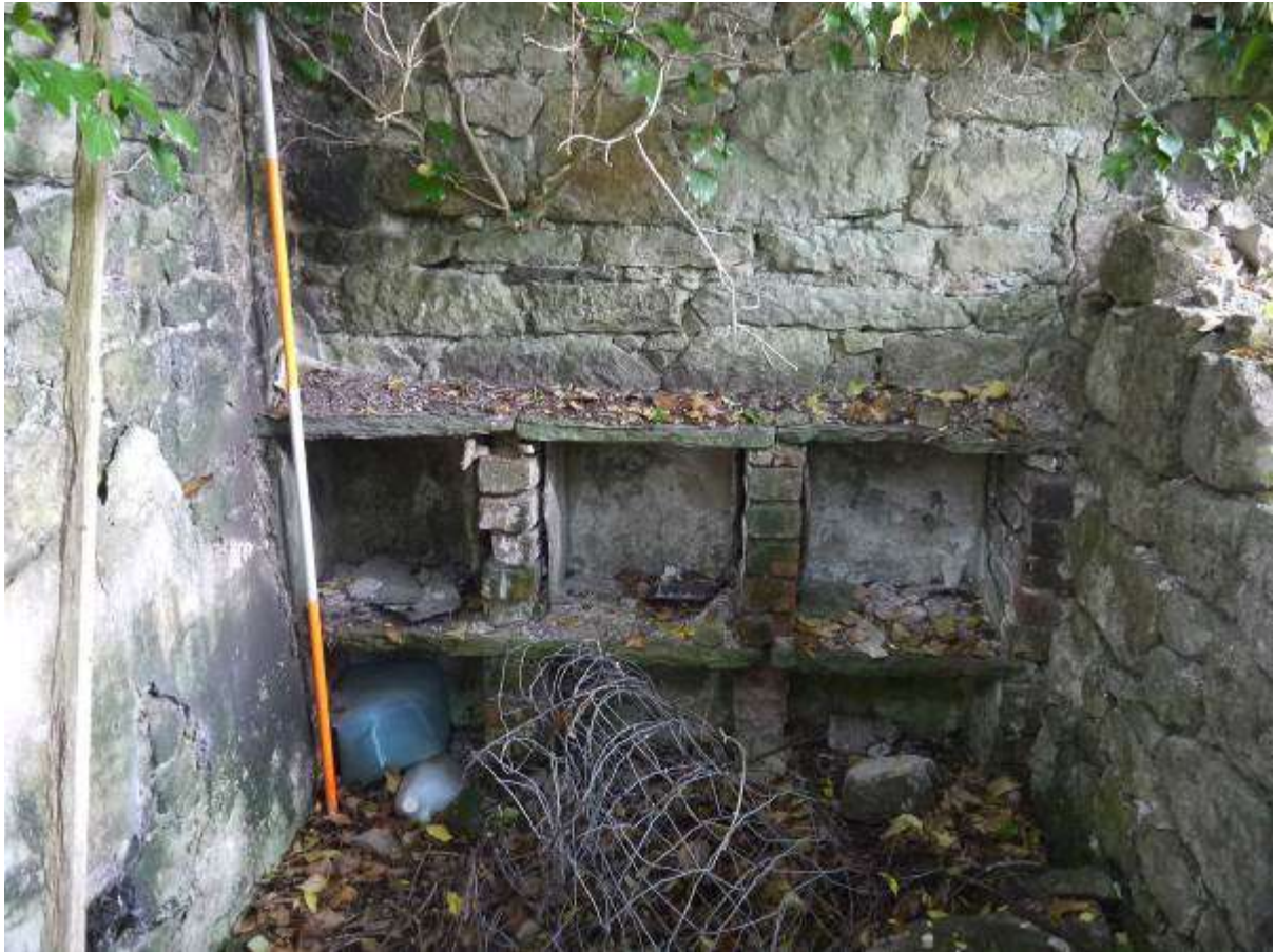
Illustration 27 Internal view of Room F showing stone and brick built boxes in wall face
