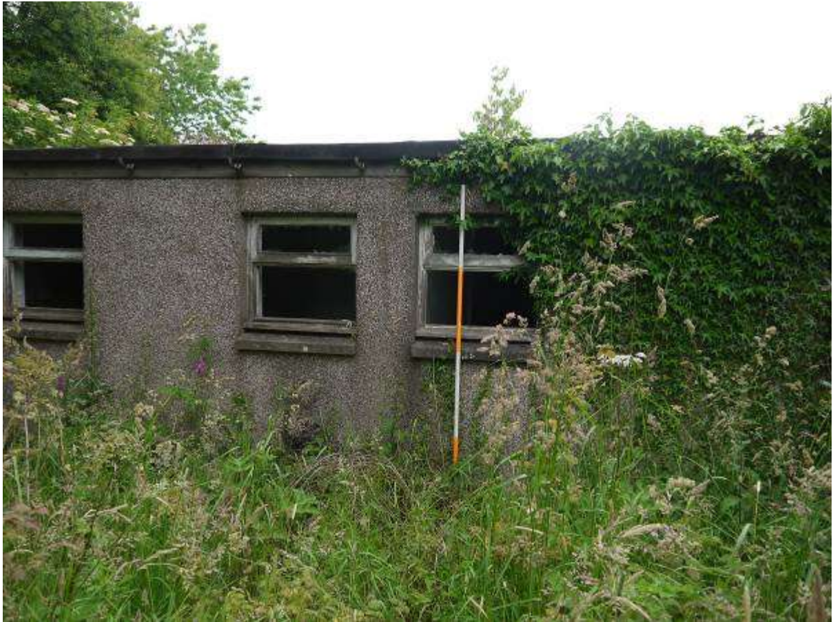
Illustration 21 South western elevation of Building 2 looking North East
