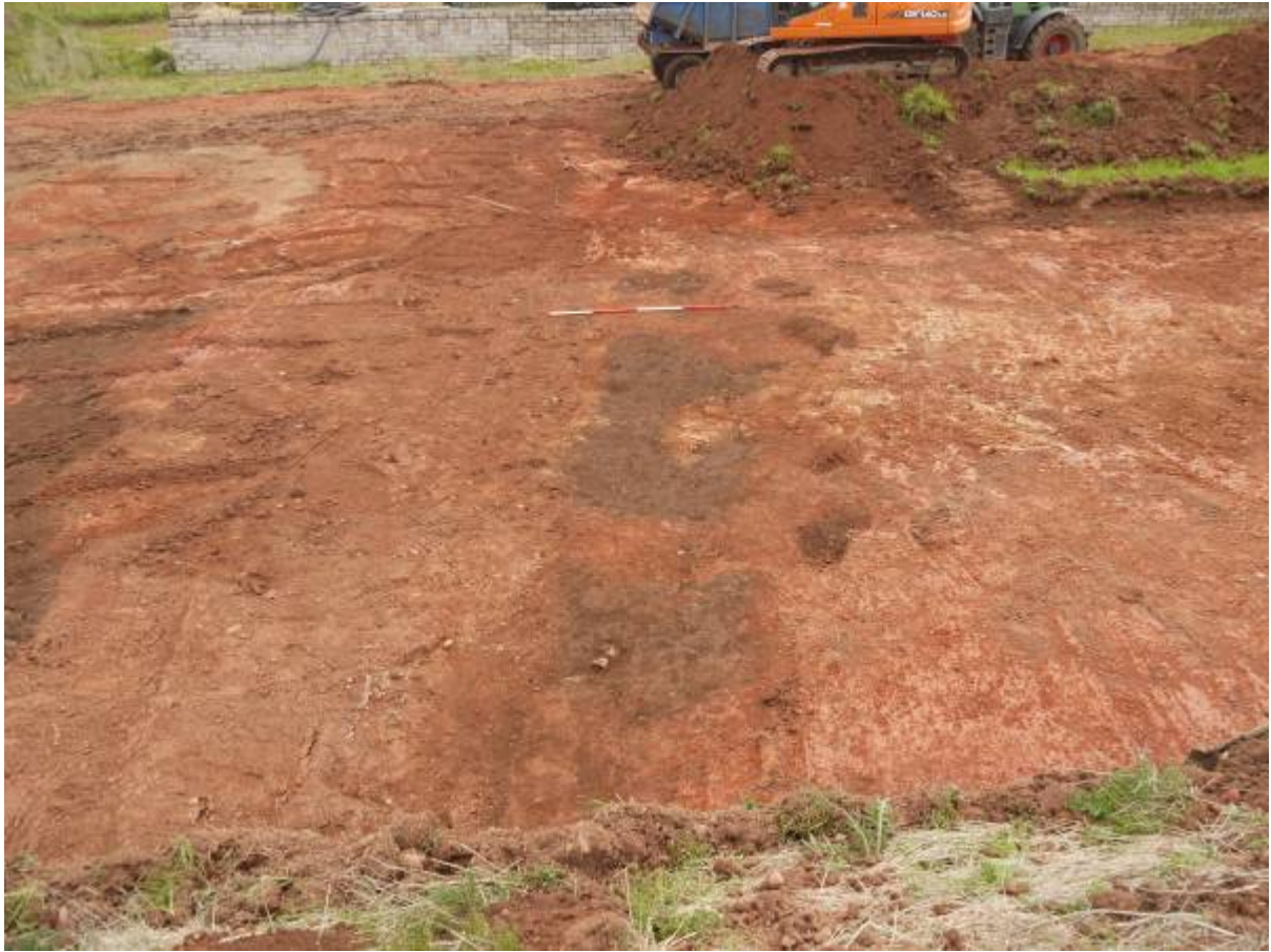
Illustration 8 Cut Feature Group 2 looking South East
