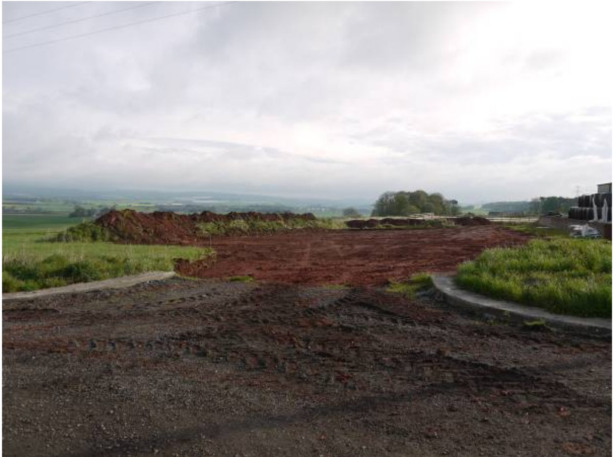
Illustration 3 Site A completely stripped of ploughsoil looking North East
