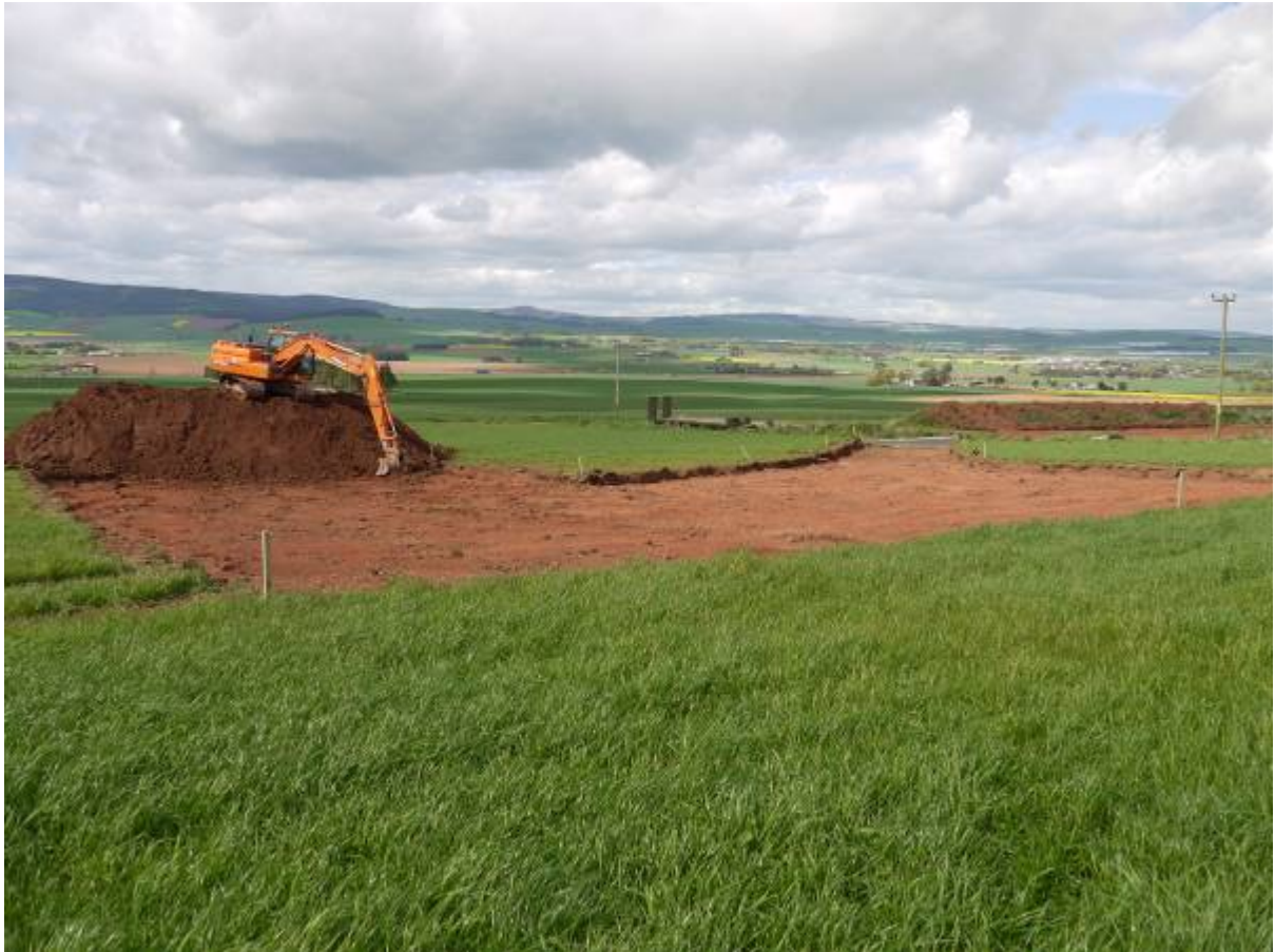
Illustration 14 Site B (house and access road) completely stripped of ploughsoil looking North
