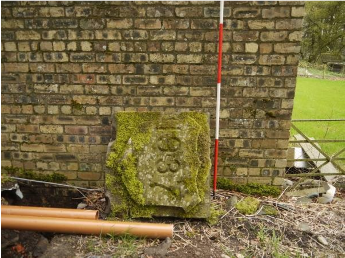
Illustration 8 Date stone propped against eastern wall of boiler house
