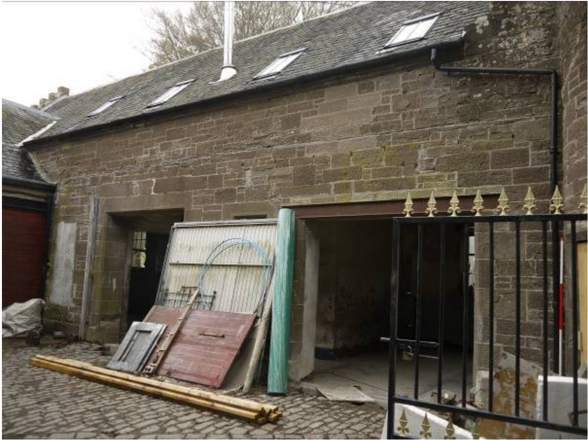
Illustration 10 Western elevation of former stables
