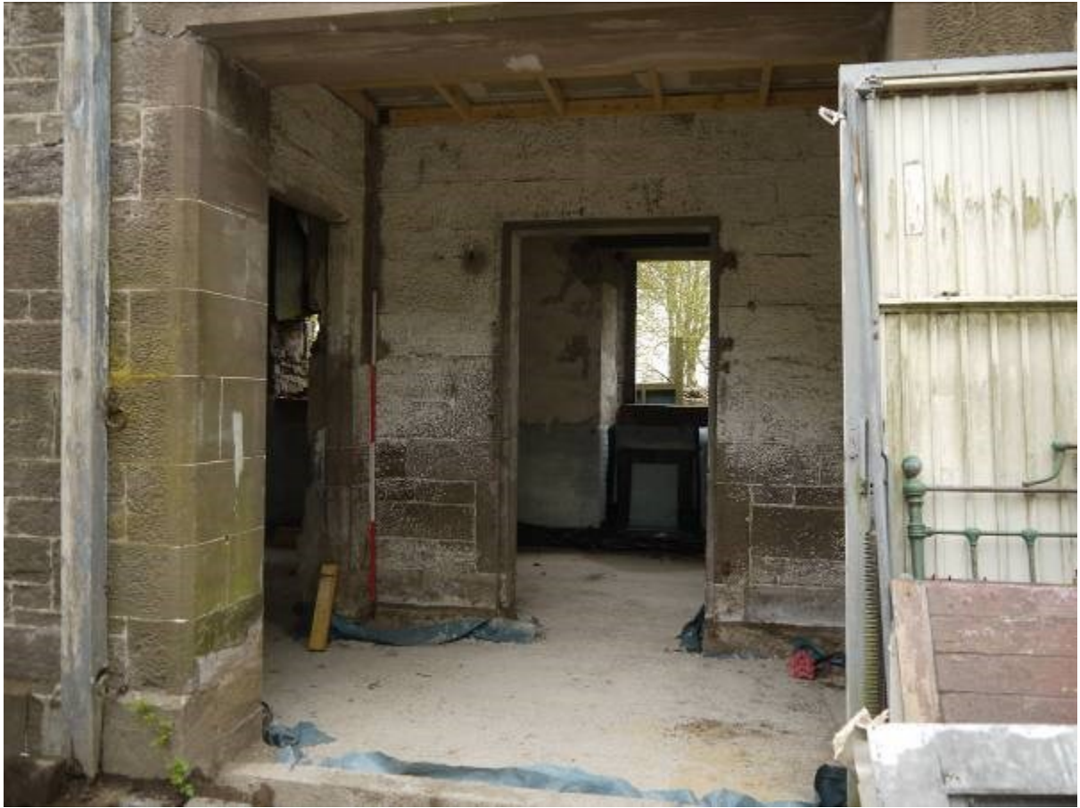
Illustration 16 Room D looking East
