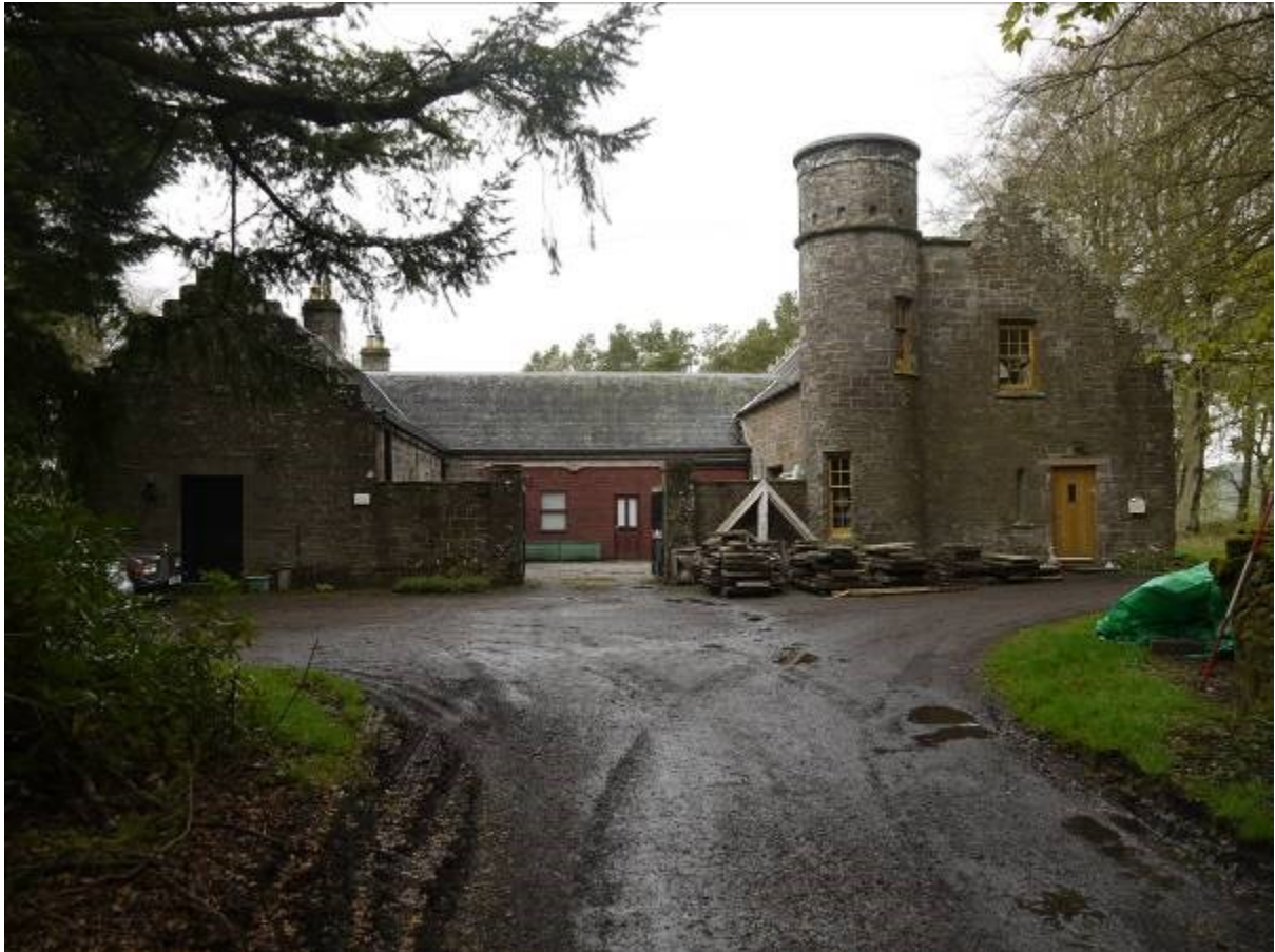
Illustration 4 Complex of buildings at South Lochton including former stables (to right with stair tower) looking North
