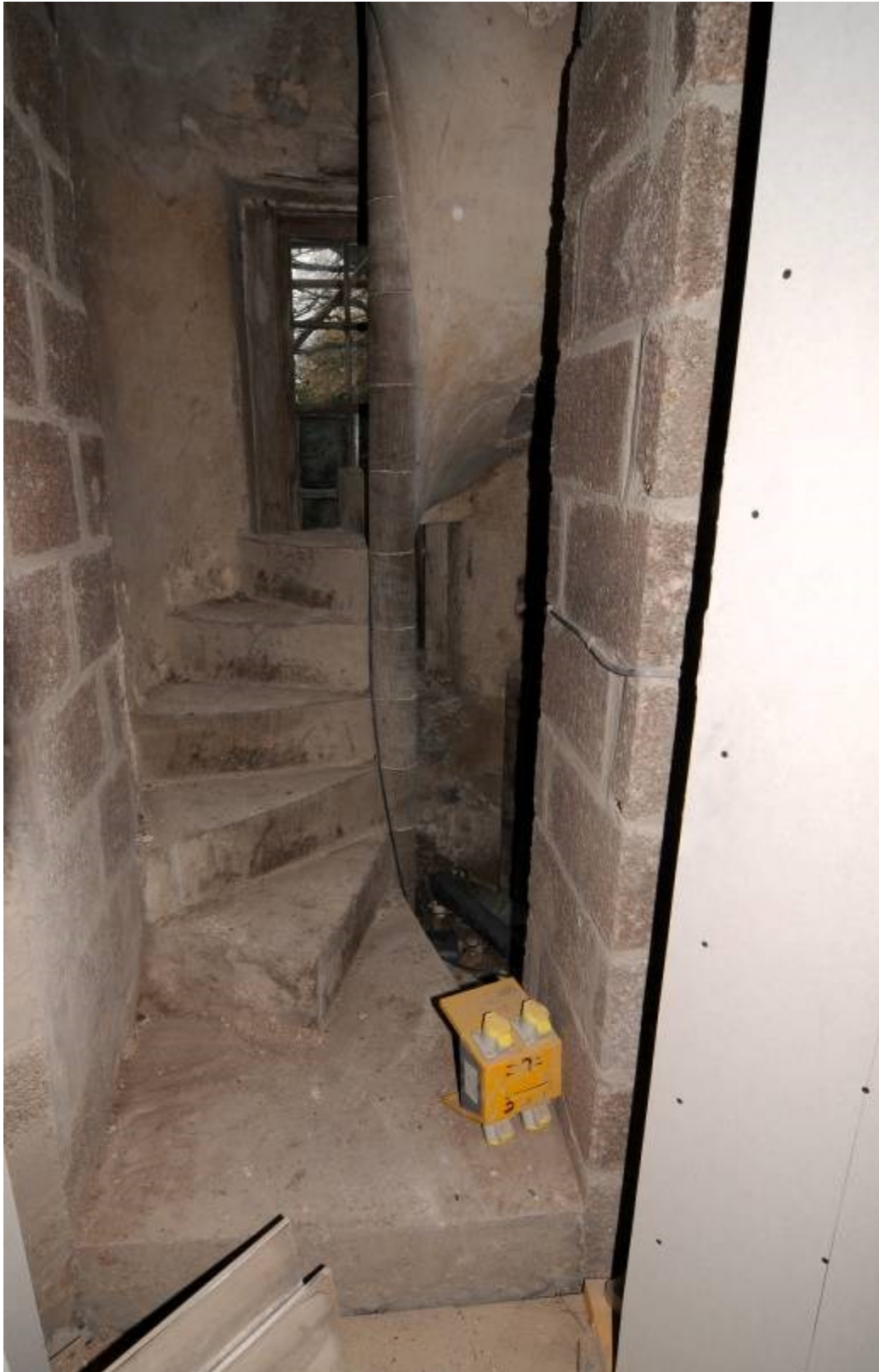
Illustration 17 Interior of Room E showing access to stair tower
