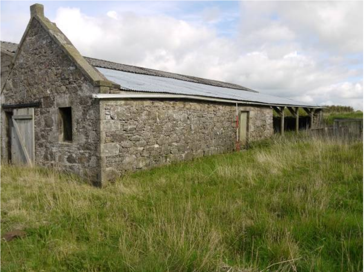
Illustration 14 Southern end of East facing elevation showing Structure 2 in foreground
