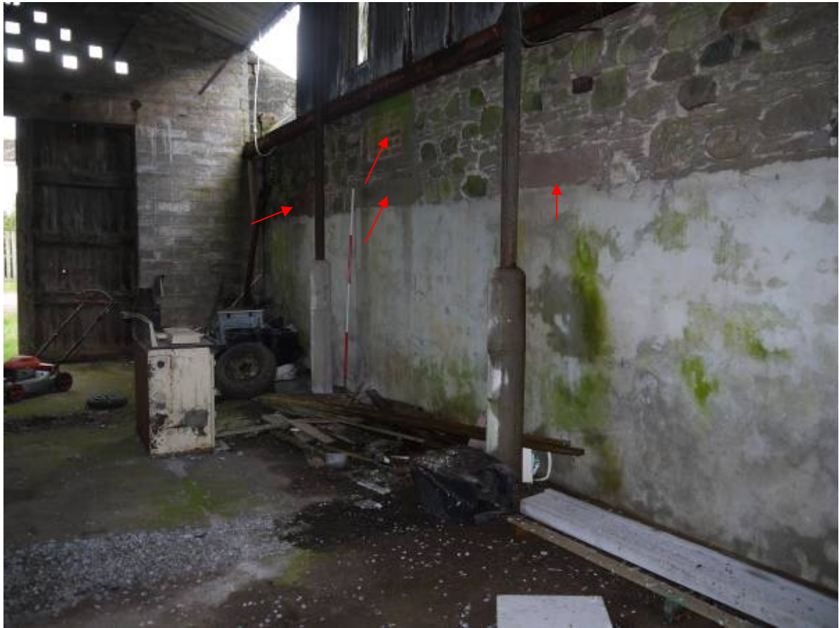
Illustration 22 Western elevation of Structure 1 (now inside amalgamated structure) showing blocked windows and doorway (red arrows)
