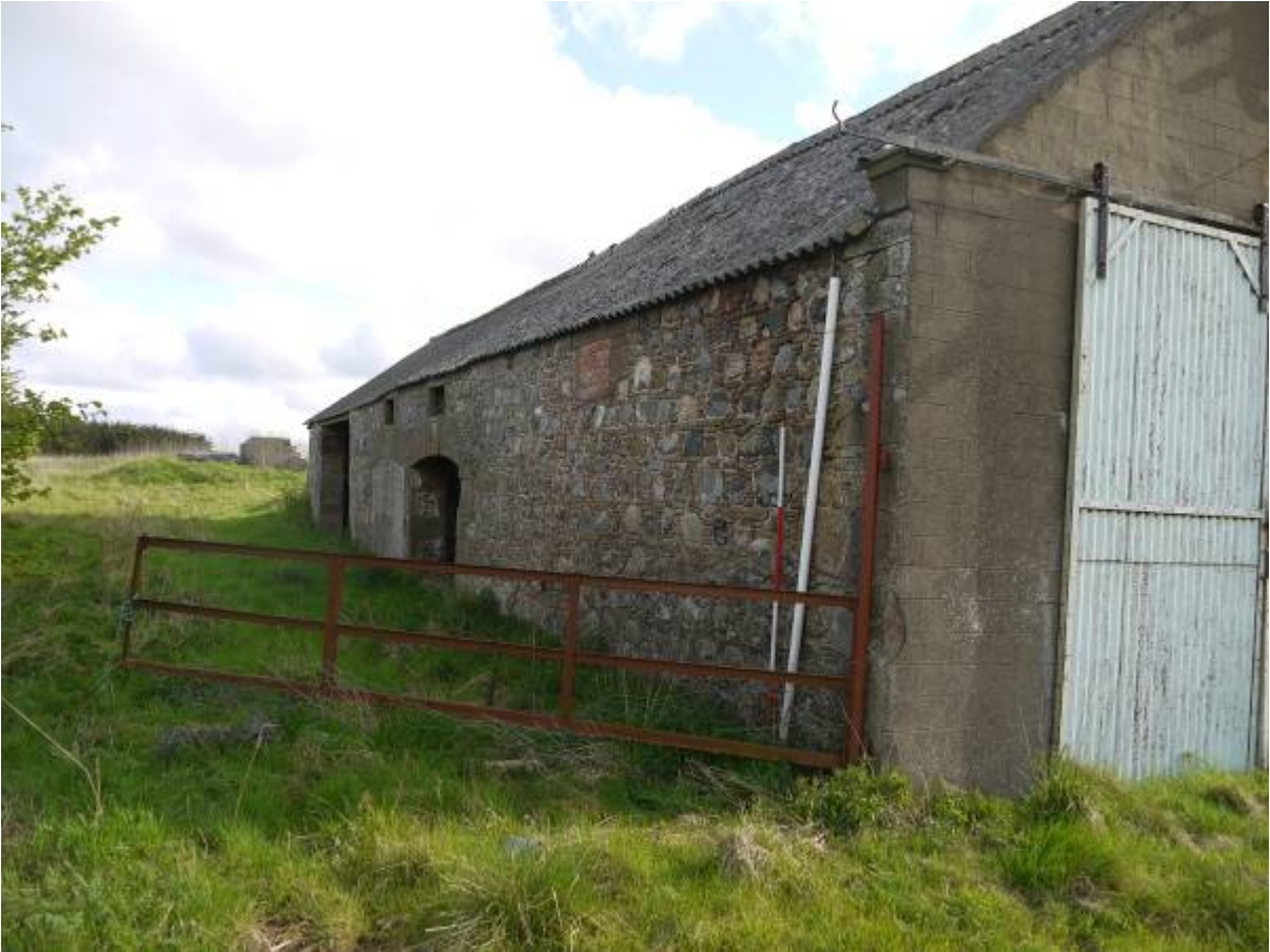
Illustration 5 West facing elevation of Structure 1 looking NE
