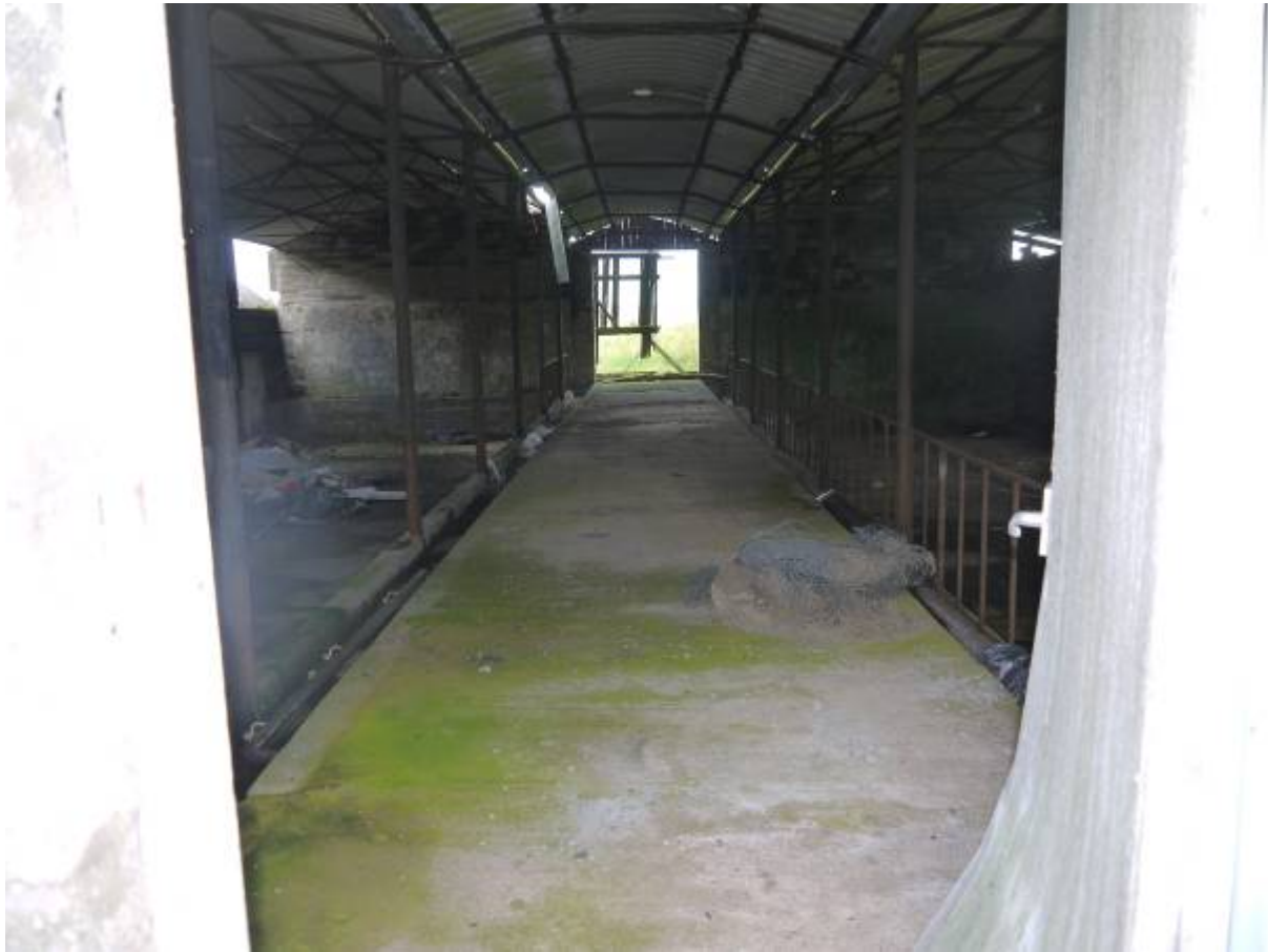
Illustration 16 Internal elevated walkway in Structure 3 looking north
