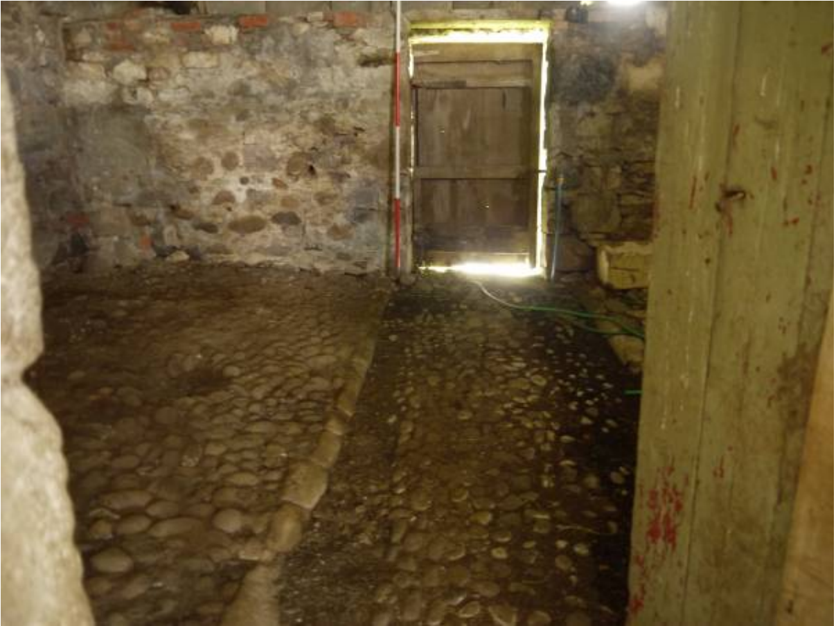
Illustration 24 Cobbled floor inside Structure 2 showing defined walkway to doorway
