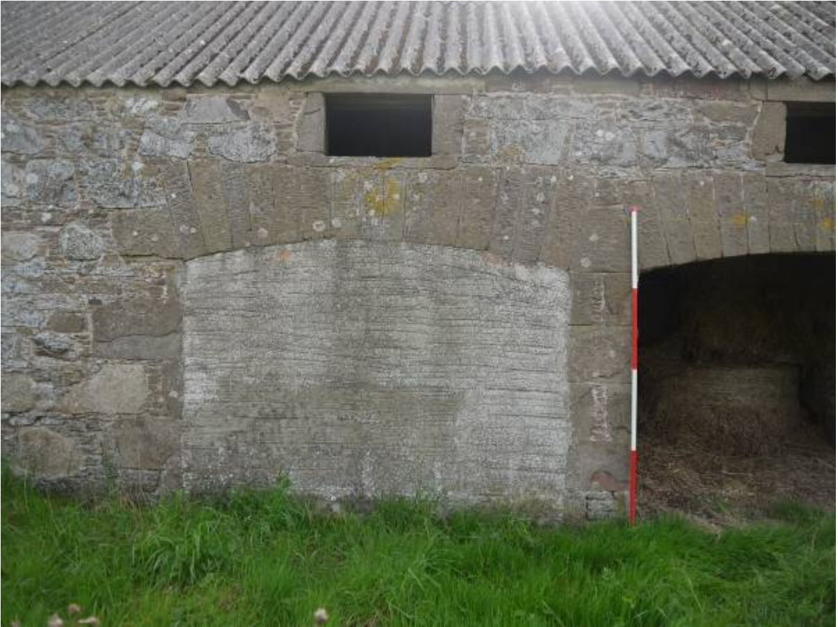
Illustration 8 Blocked arched entrance in West facing elevation of Structure 1
