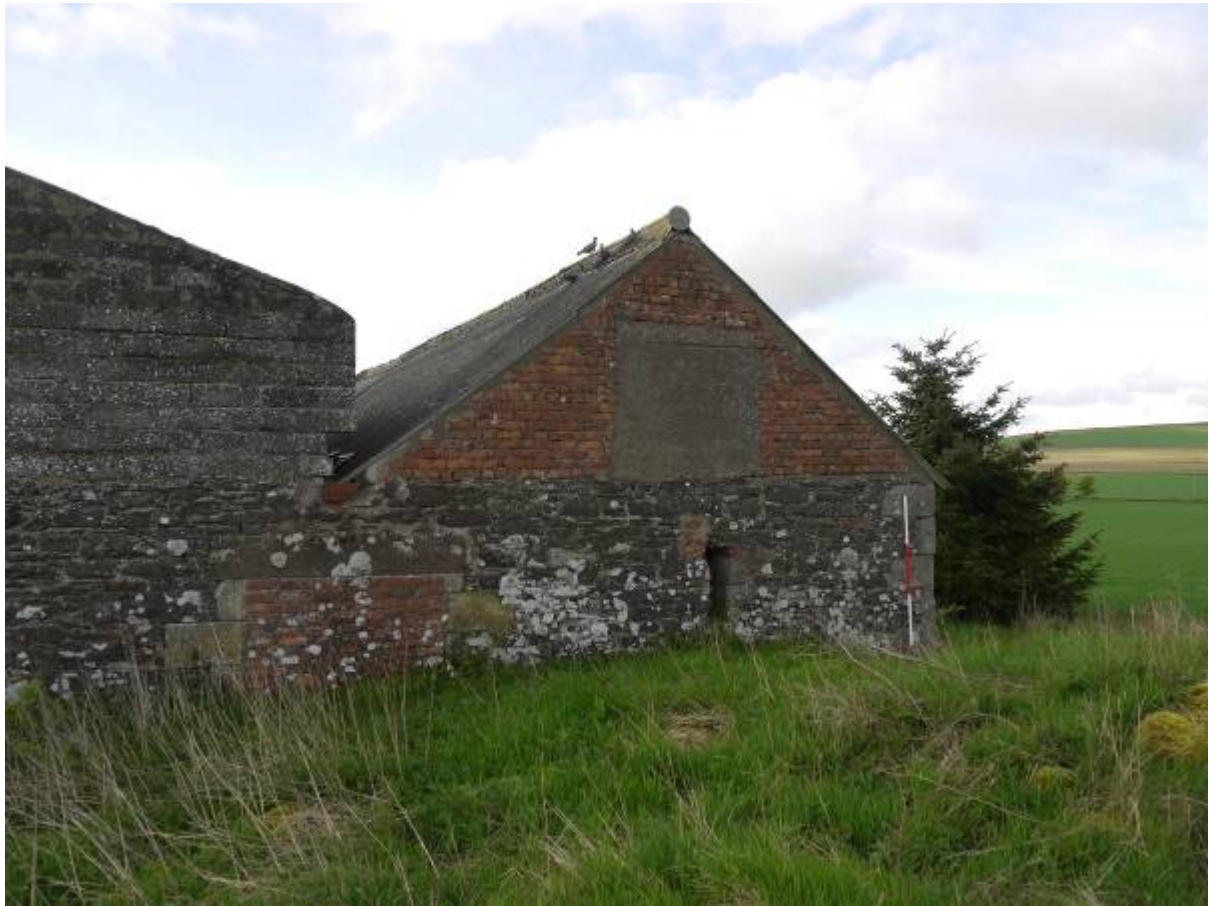
Illustration 11 Detail of Western end of North facing elevation showing blocked window and doorway
