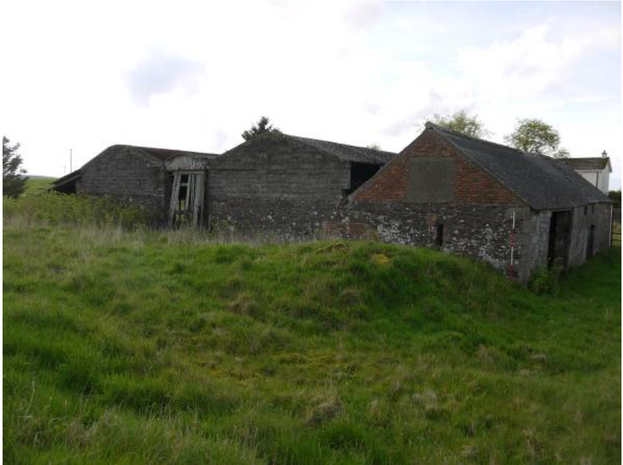
Illustration 10 North facing elevation looking SE Structure 1 to right
