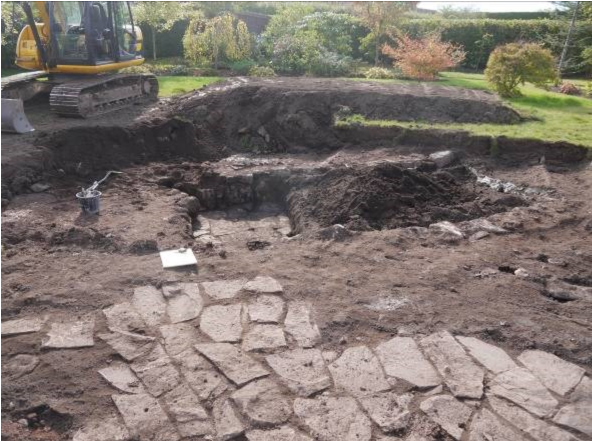
Paving and sunken garden looking west
