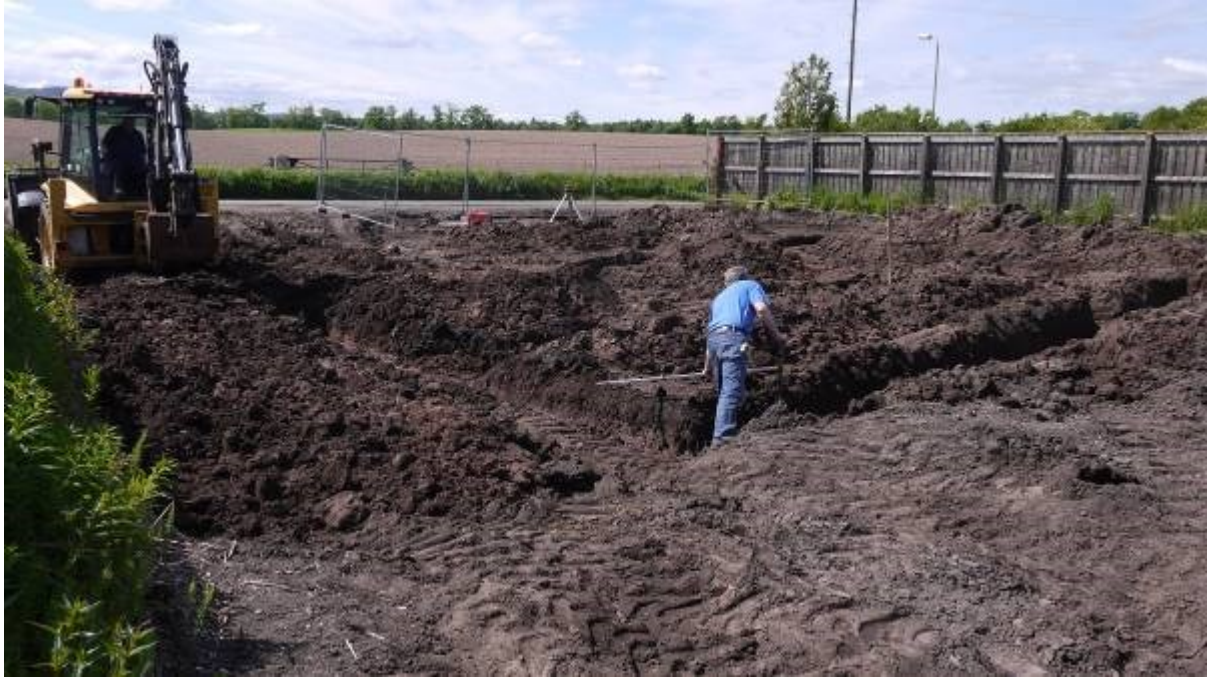
Illustration 8 Excavated foundation trenches at Eastern end of site
