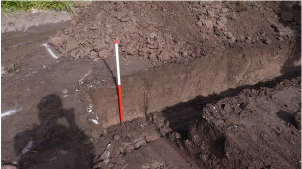
Illustration 7 Excavated trench section showing subsoil sitting above natural grey sandy silt at Western end of site
