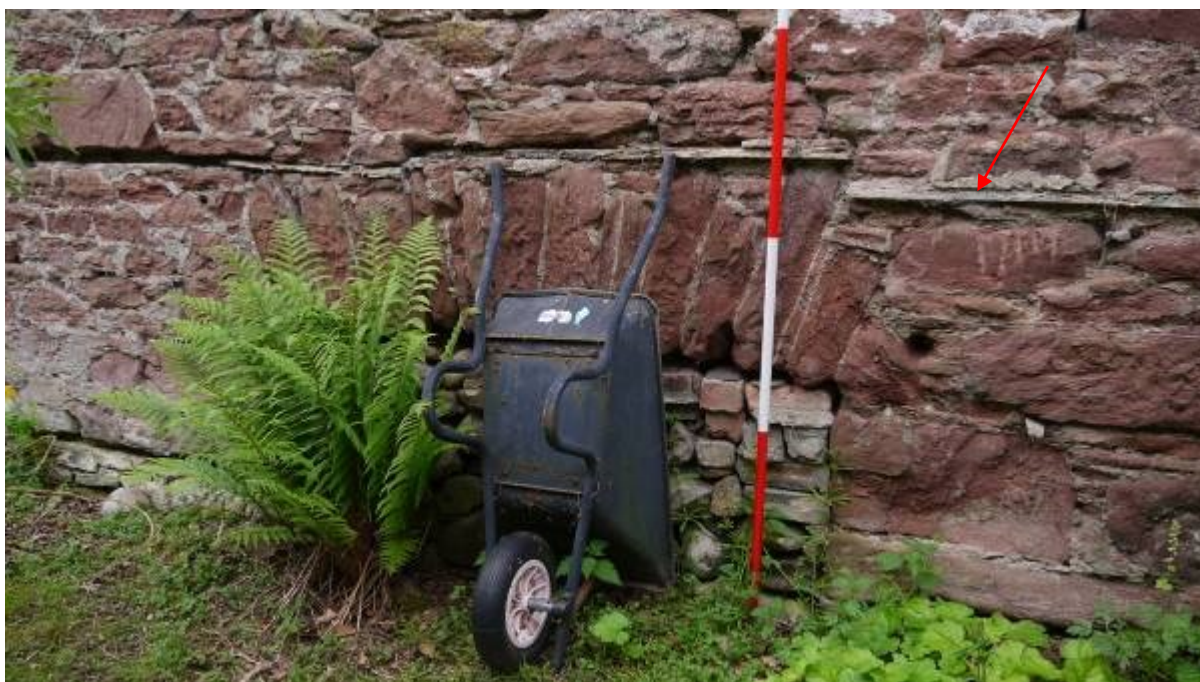
Illustration 19 Relieving arch in internal Southern elevation of Building A, panelling recess is visible (red arrow)
