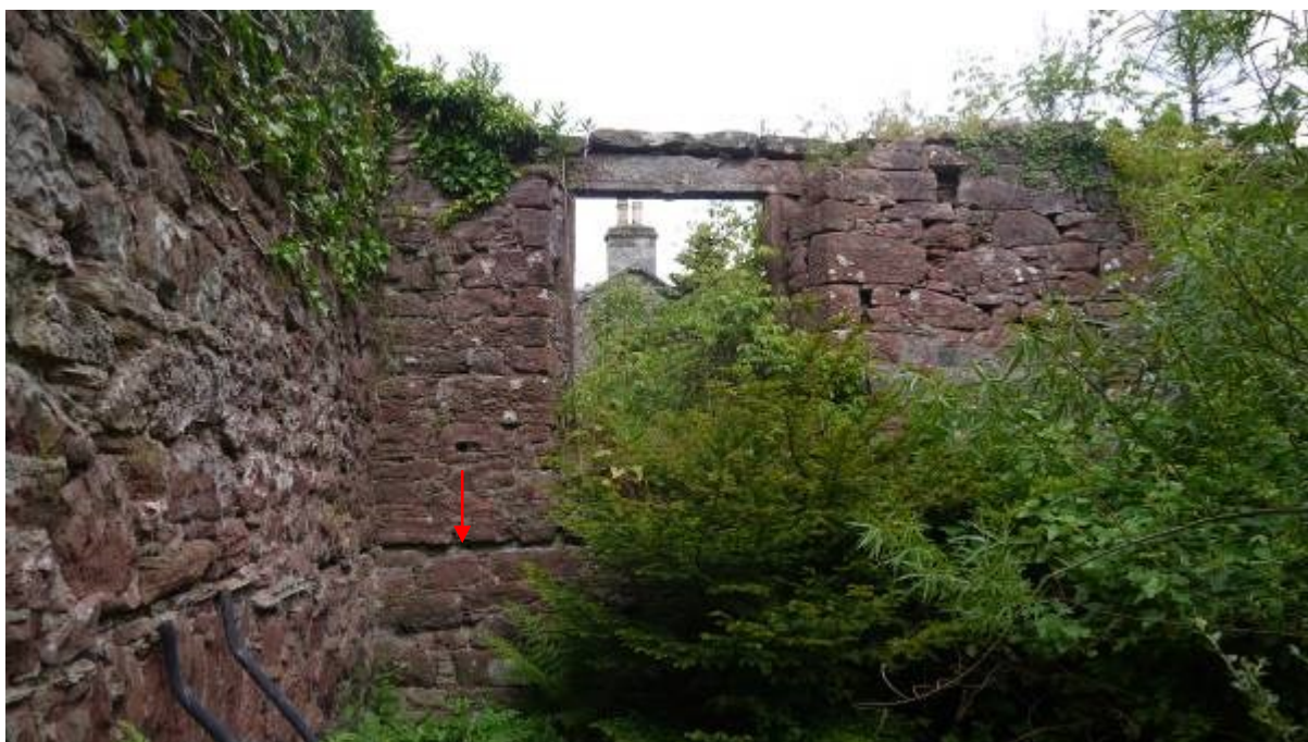
Illustration 20 Internal Western elevation of Building A (recessed groove for panelling support visible at red arrow)
