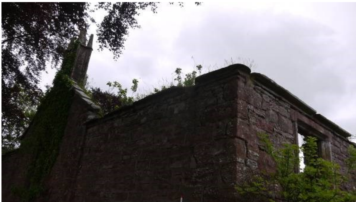
Illustration 9 Detail view of coping stones on wall head of Northern elevation of Building A at its North Western corner and on gable wall head looking East.
