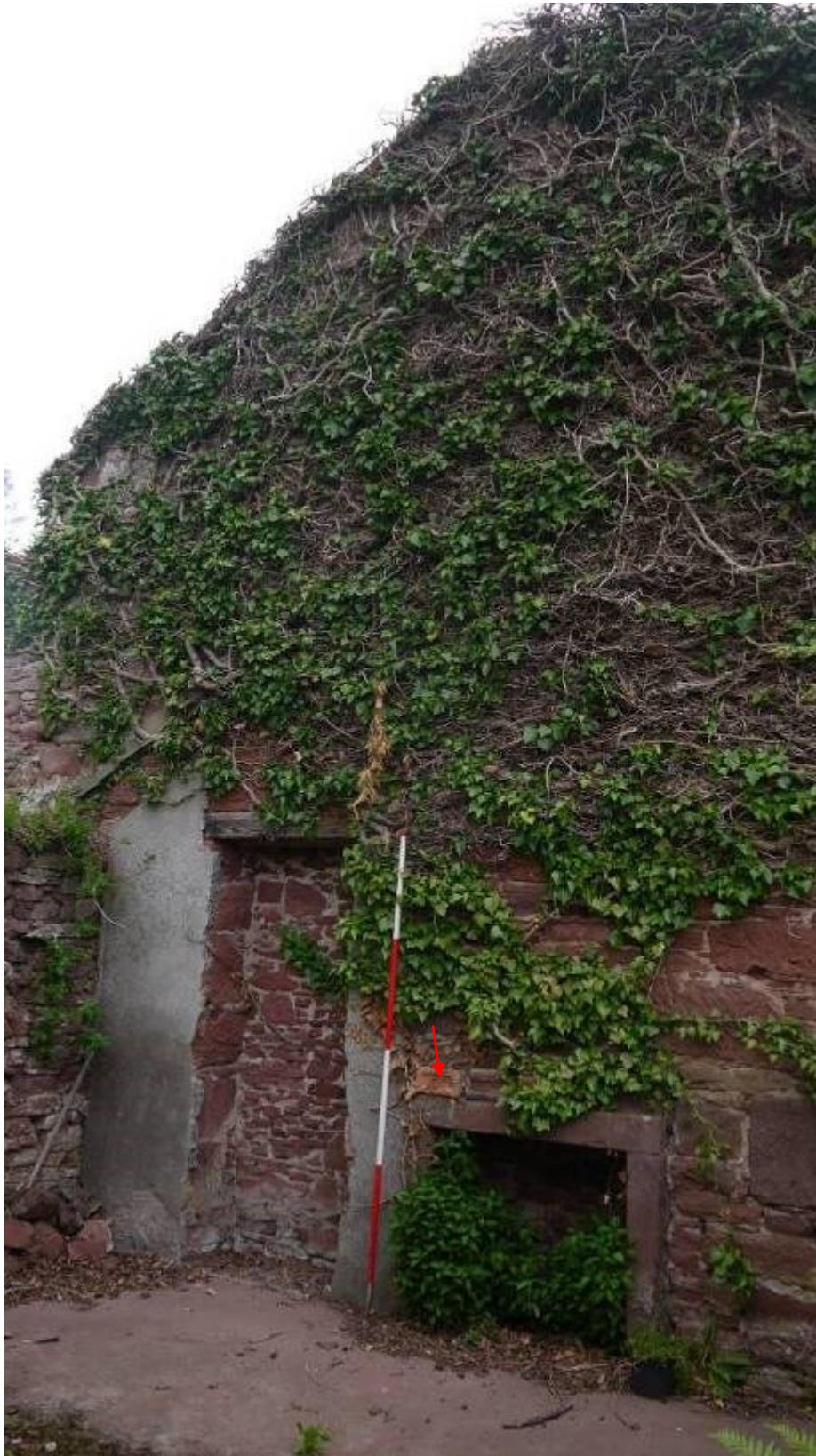
Illustration 24 Internal Northern elevation of Building B (Bricks on fireplace mantle visible at red arrow)
