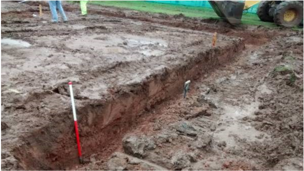
Illustration 7 Excavated eastern foundation trench looking North West
