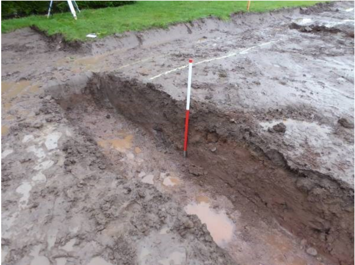
Illustration 8 Southern end of excavated eastern foundation trench for house
