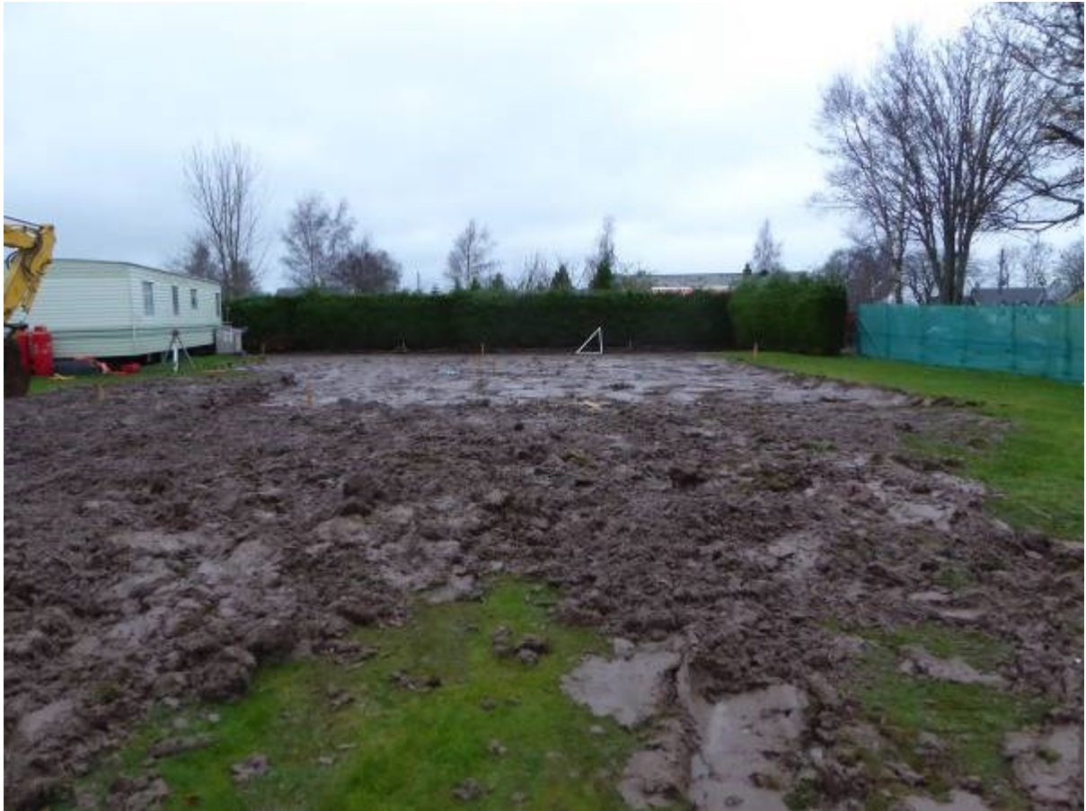
Illustration 5 General view of house plot looking West.
