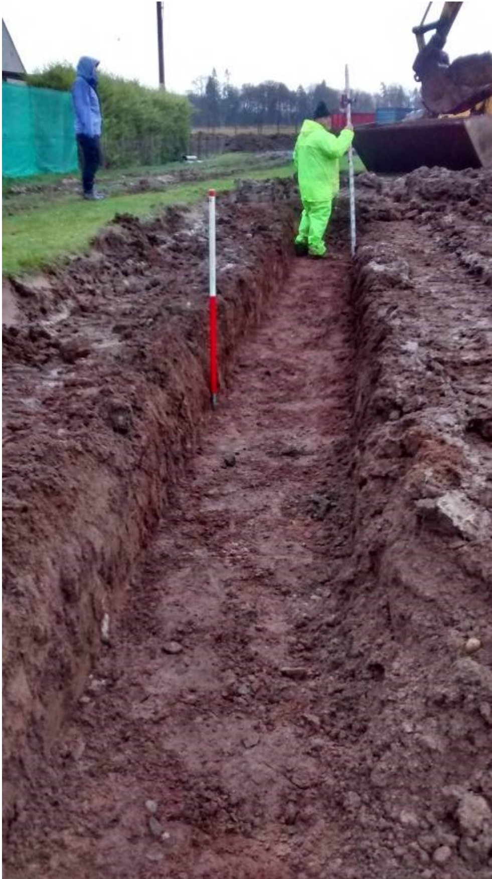
Illustration 6 Excavated northern foundation trench looking East
