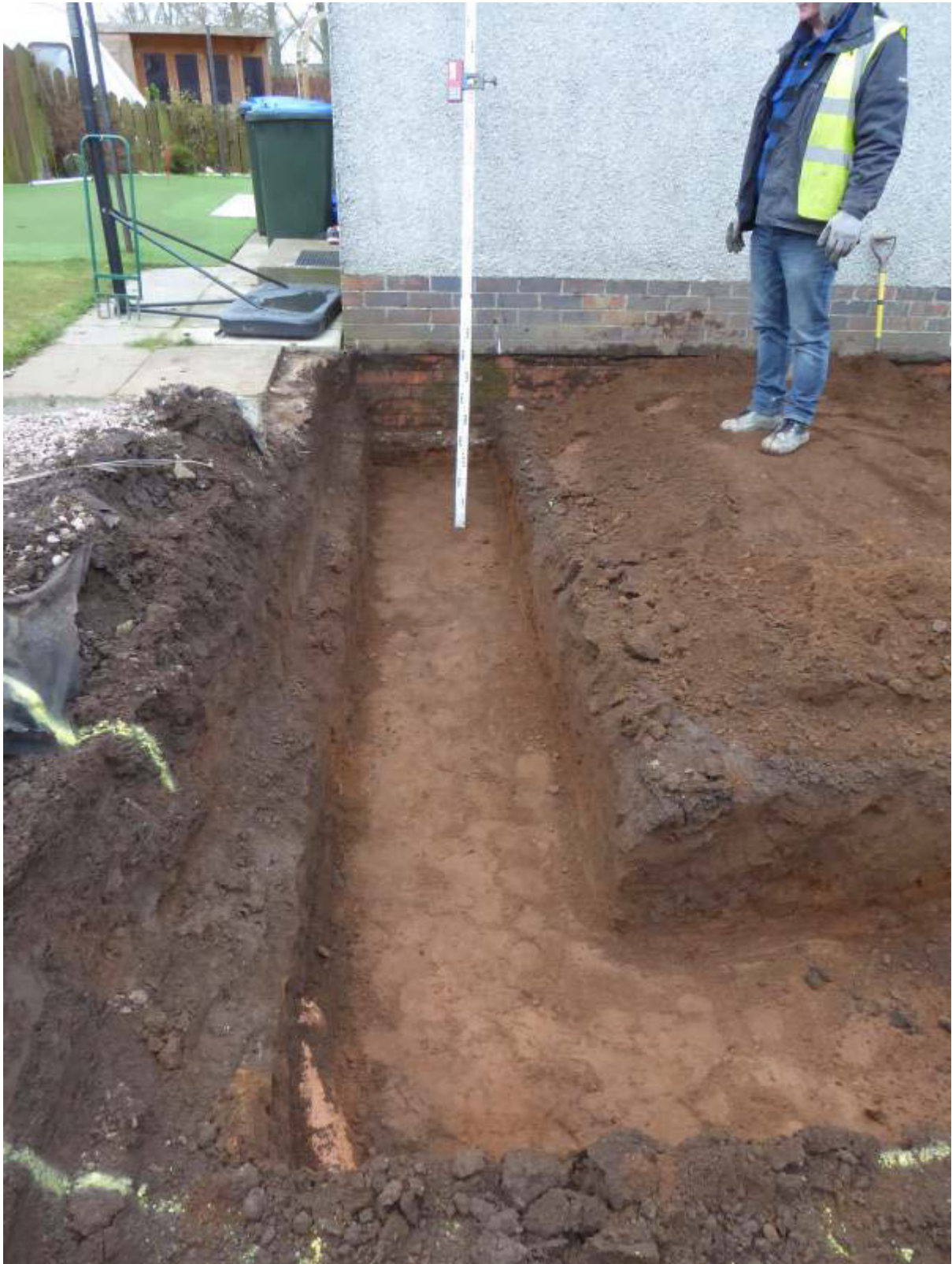
Illustration 6 Excavated trench for Eastern wall line (A) looking South
