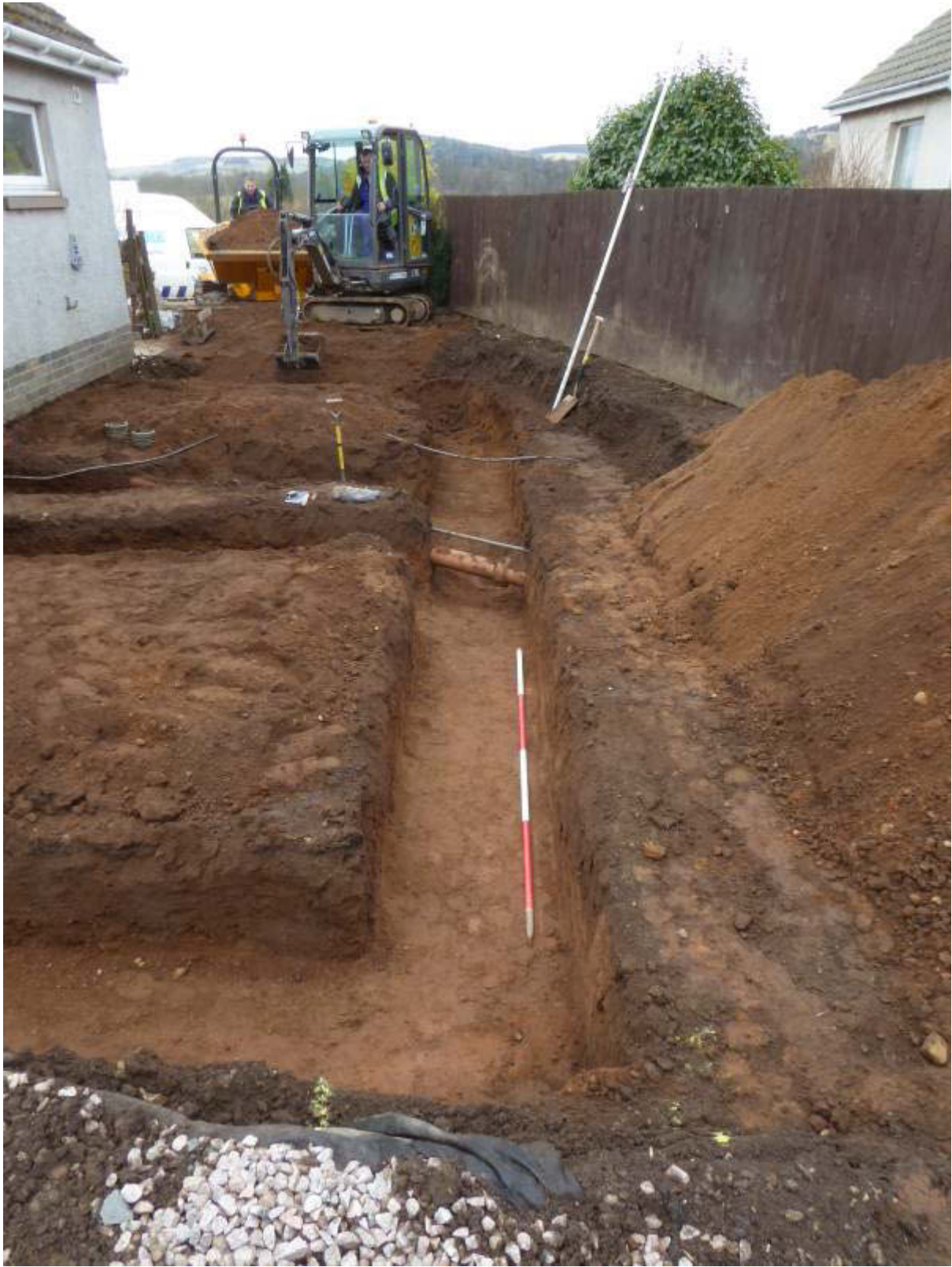
Illustration 10 Excavated line of northern wall trench (D) looking West.
