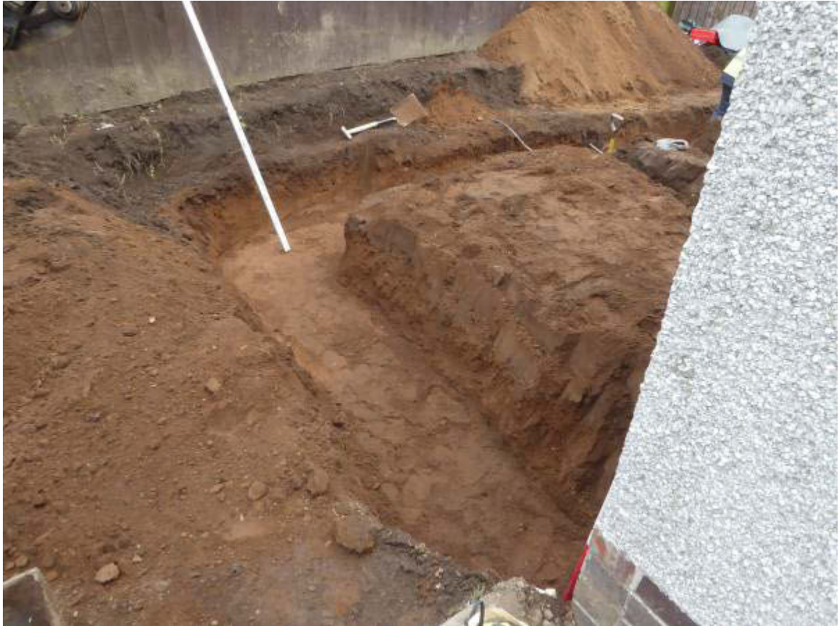
Illustration 11 Excavated line of western wall line (E) looking North East.
