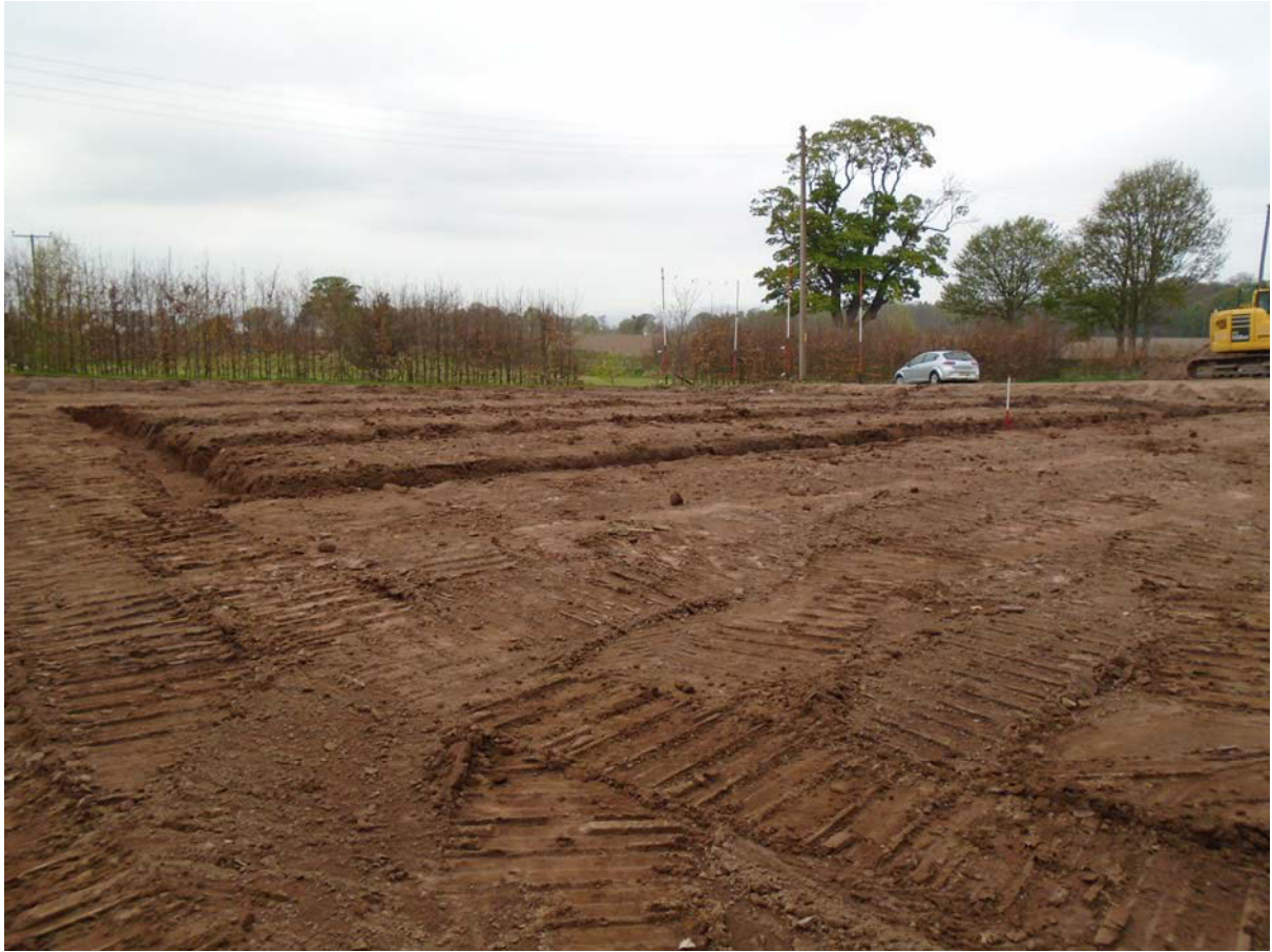
Illustration 6 General view of excavated foundation trenches looking North West
