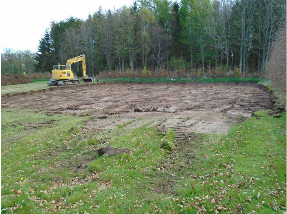
Illustration 5 Plot stripped of topsoil looking East
