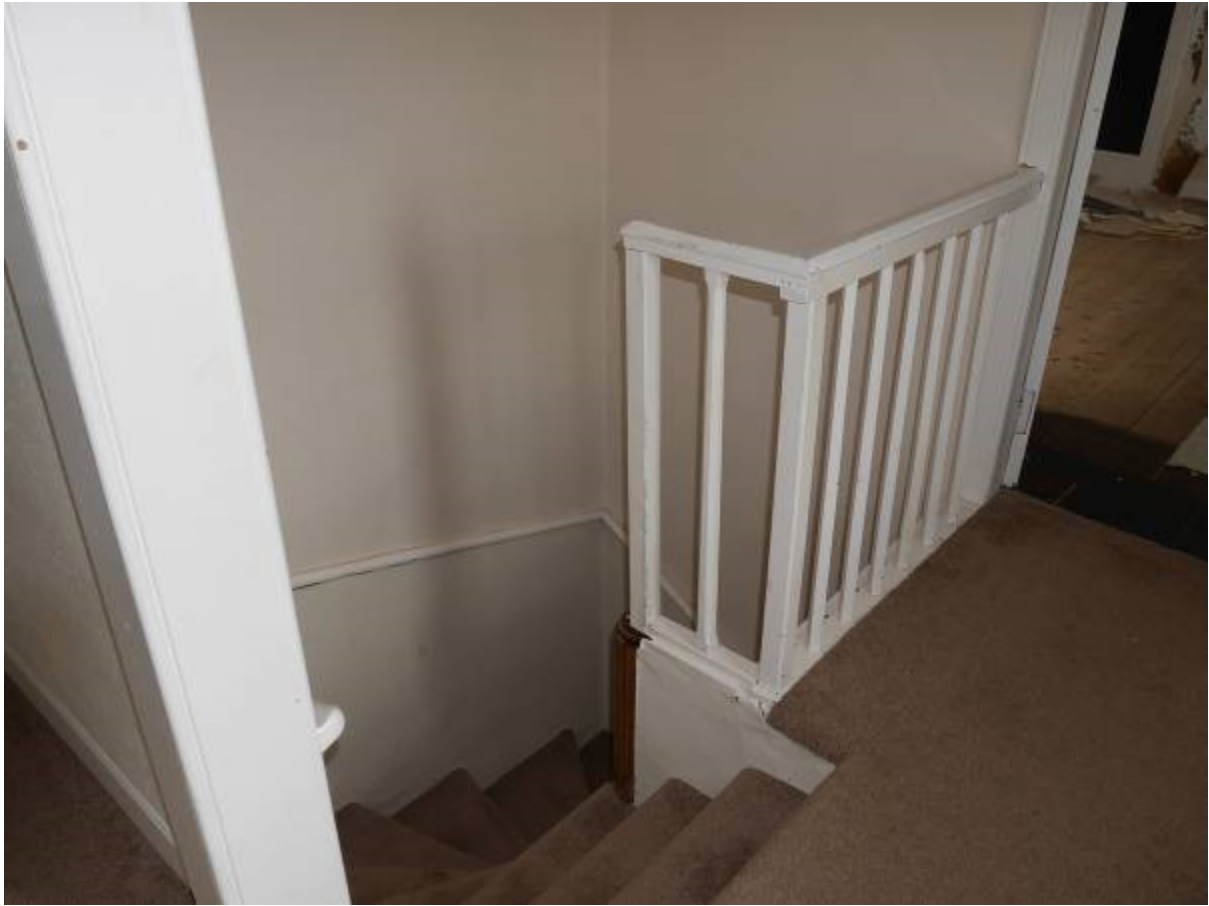
Illustration 23-Wooden balustrade at the top of the stairs
