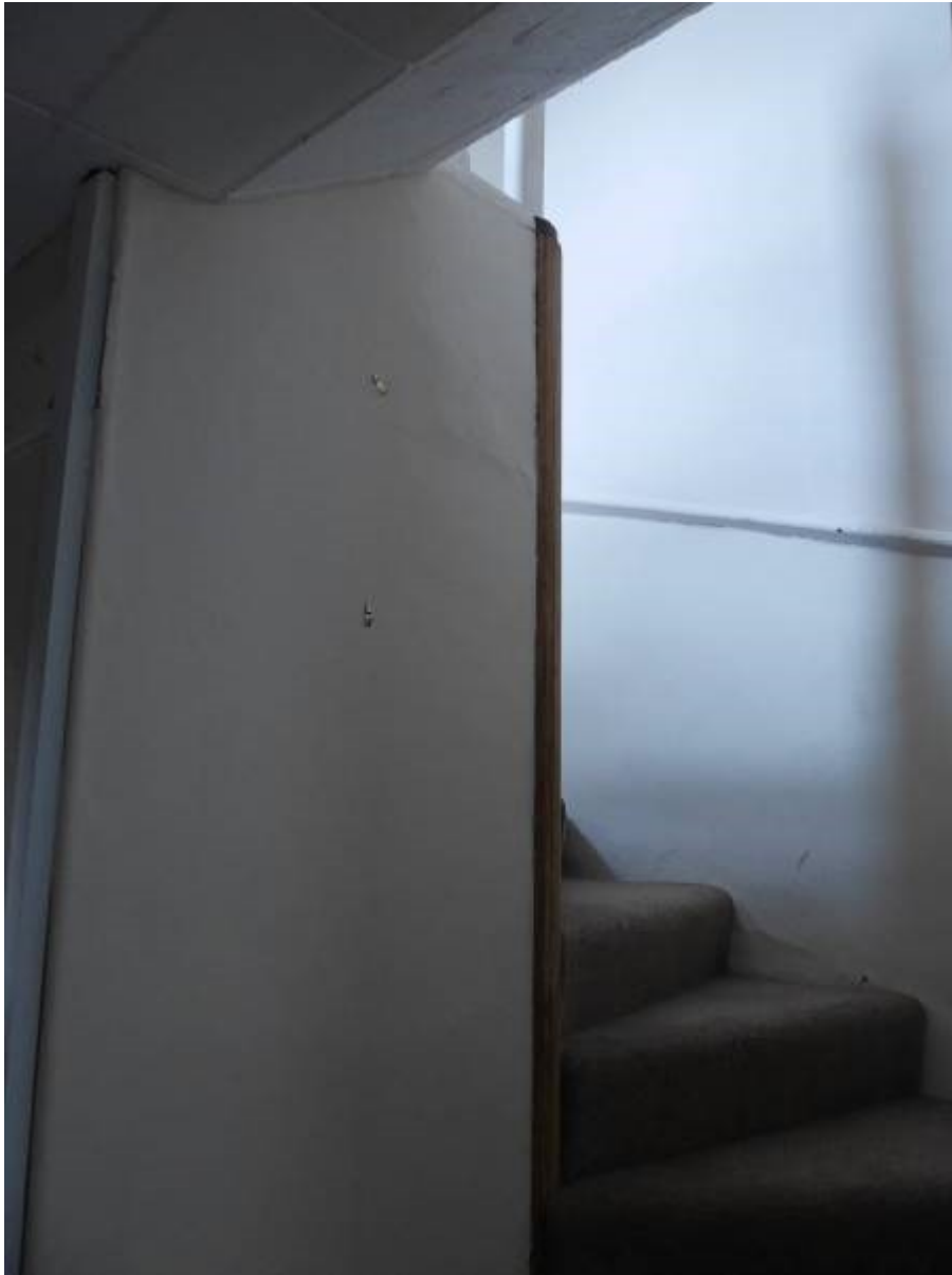
Illustration 22-Stairs up to first floor level showing central wooden pillar
