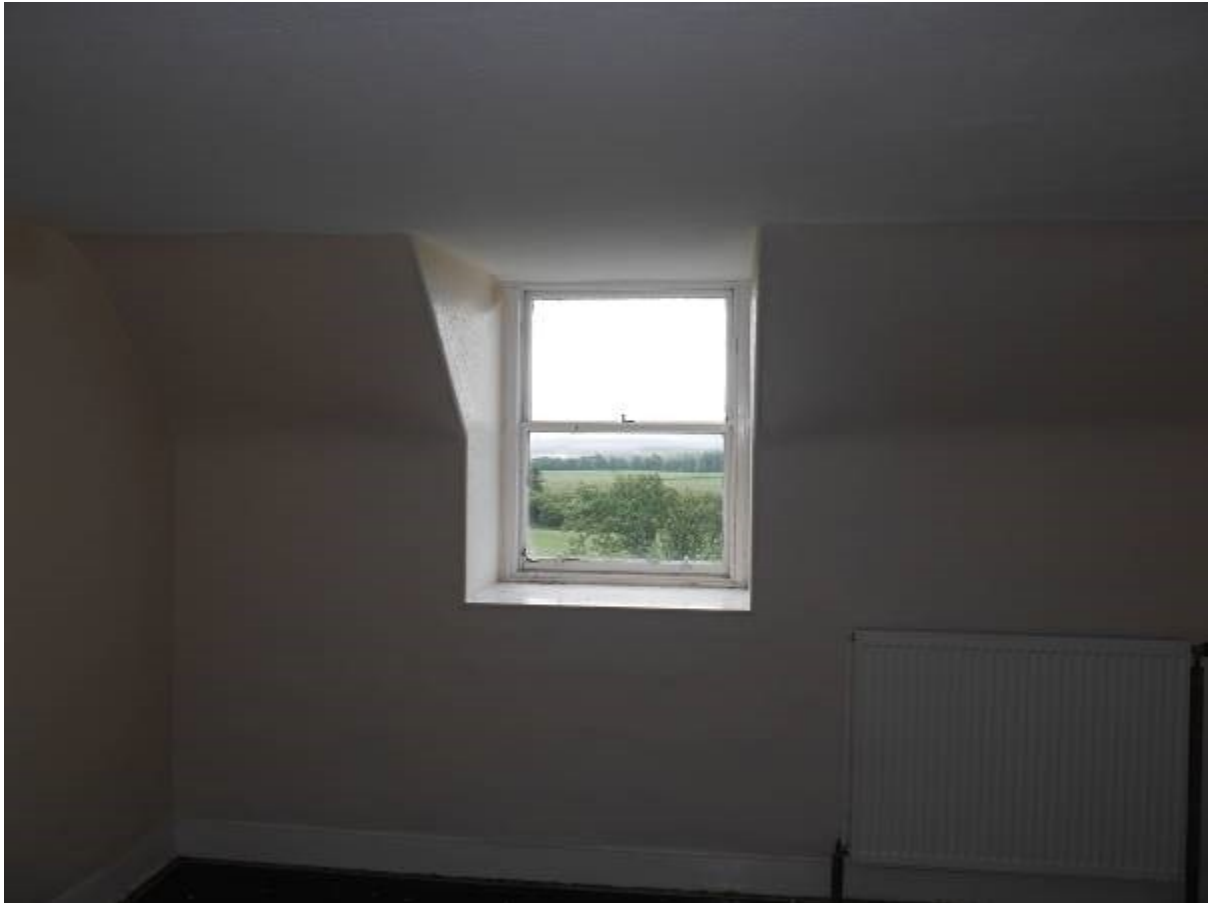
Illustration 26- Interior of gable window in upstairs bedroom (10) looking South
