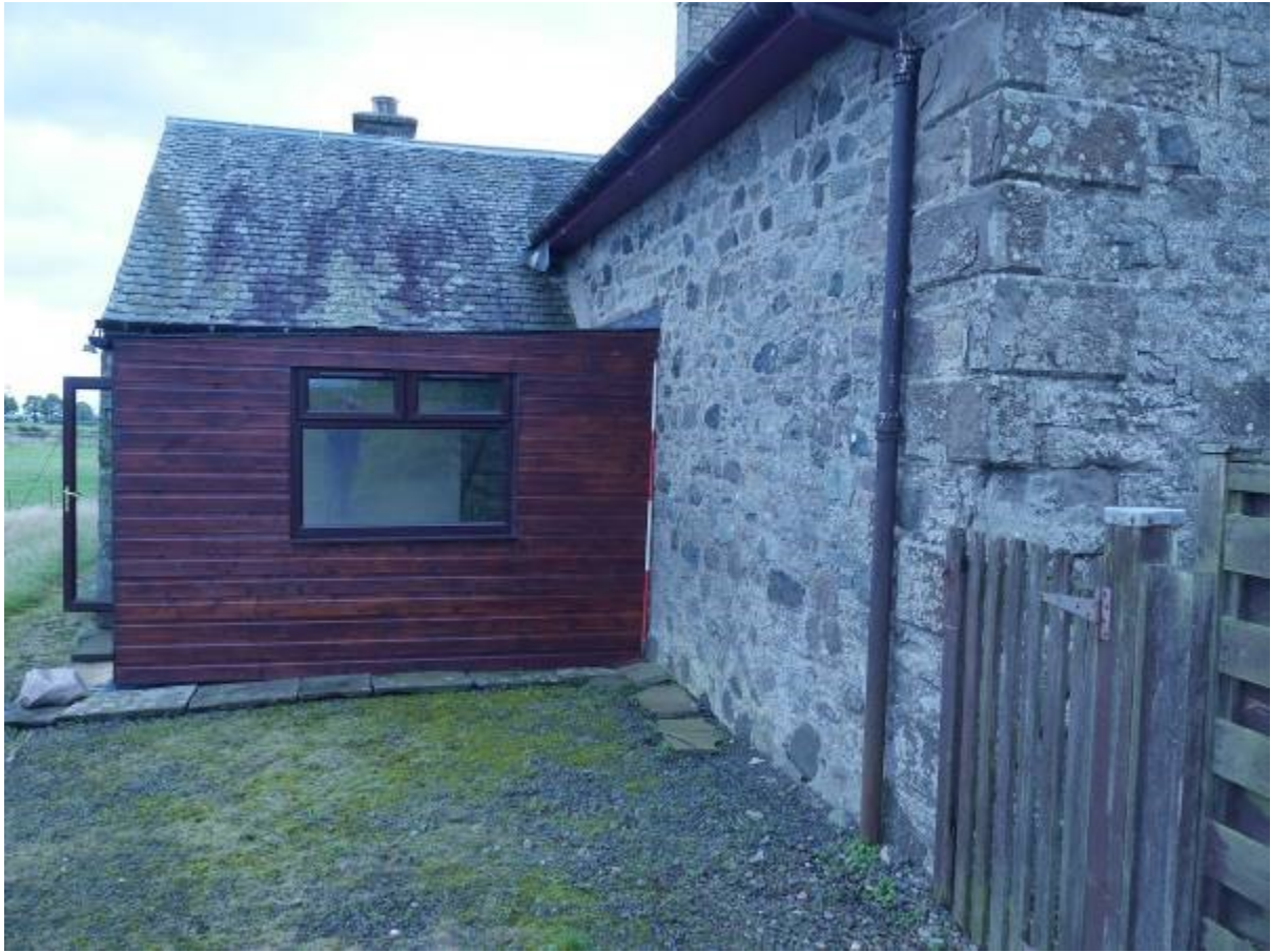
Illustration 12-Modern wooden porch (1) attached to Northern elevation of farmhouse looking East
