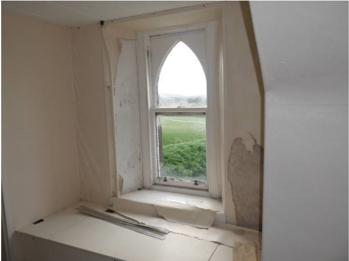
Illustration 24-Interior of window in pediment looking South from upper lobby (9)
