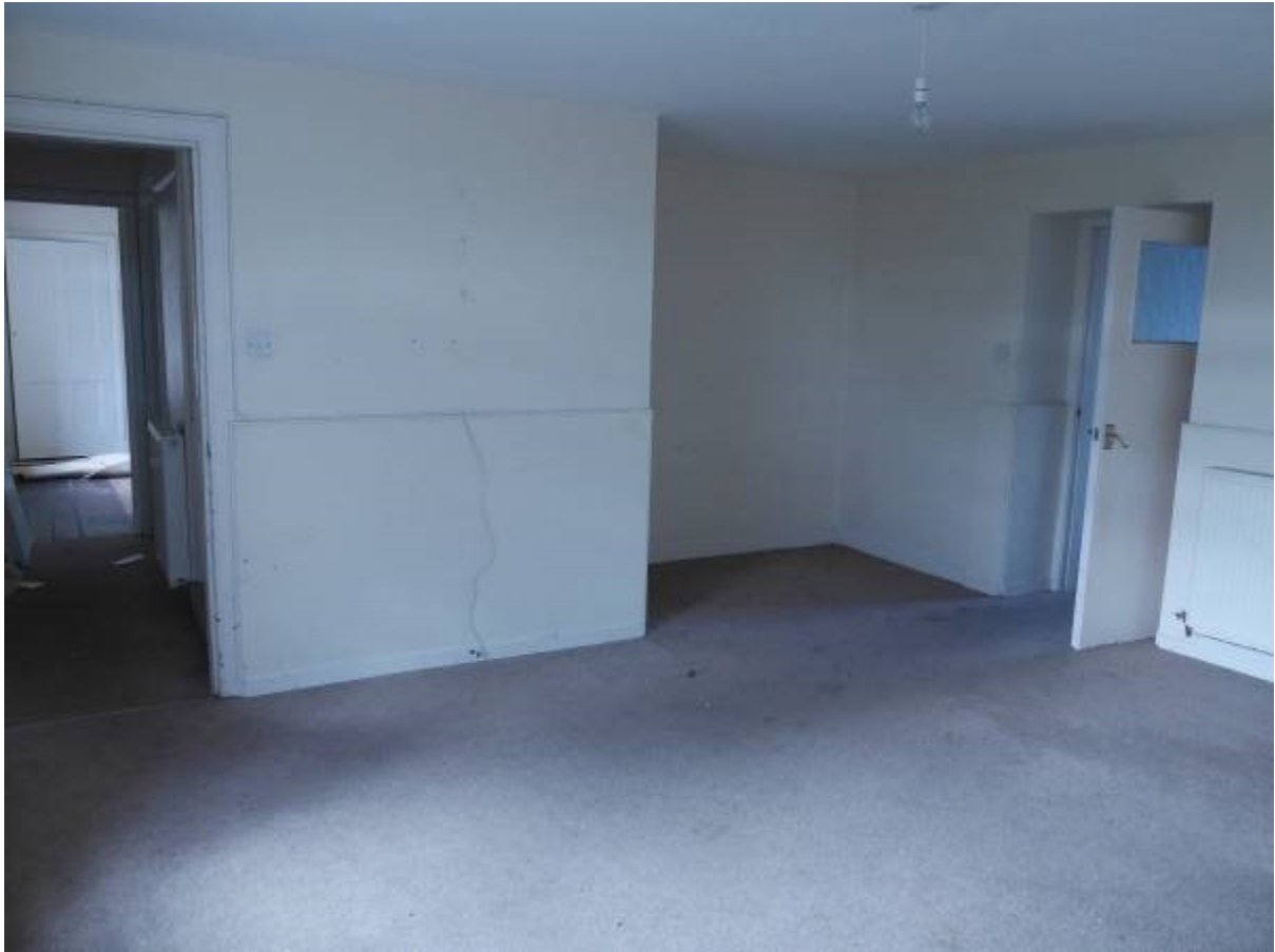
Illustration 15-Lounge (3) looking West showing enclosed stairwell to first floor
