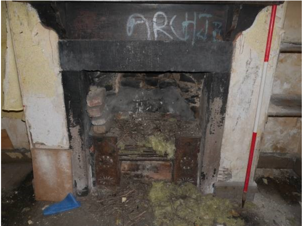
Illustration 33 -Detail of fireplace in 'bothy' (14) showing decorated cast iron grate and graffiti
