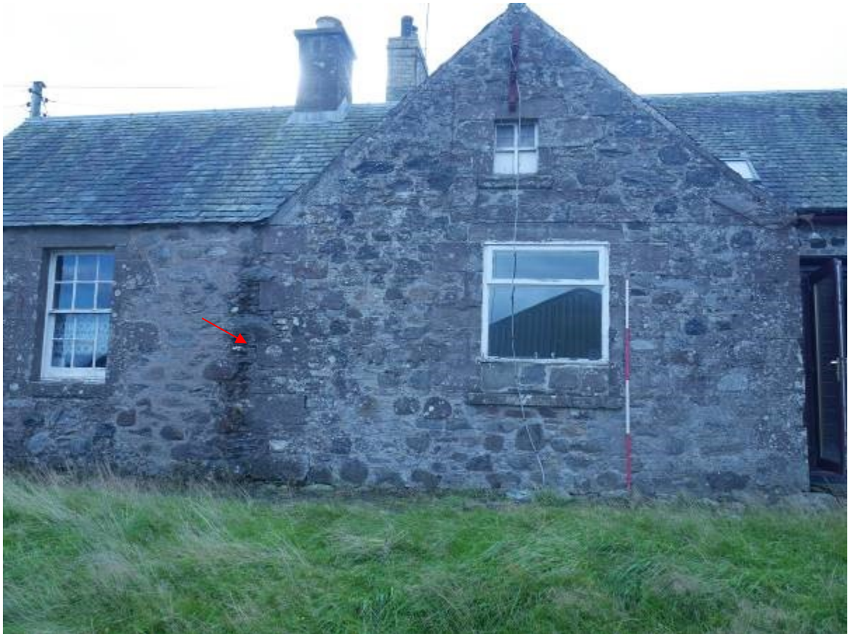
Illustration 8-Detail of Northern elevation showing junction of 'bothy' with original Eastern end of farmhouse, shaped ashlar quoins visible (red arrow)
