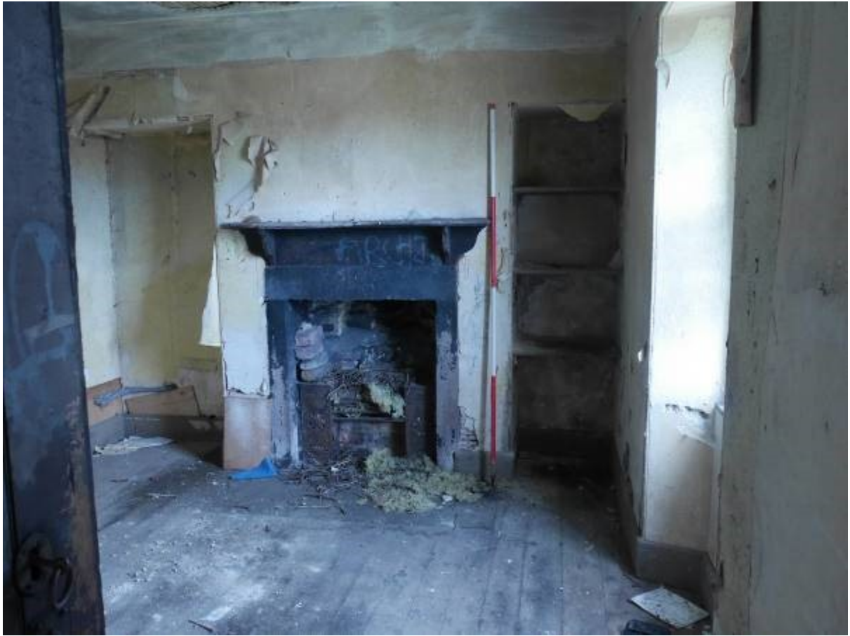
Illustration 31-General view of interior of 'bothy' (14) looking West
