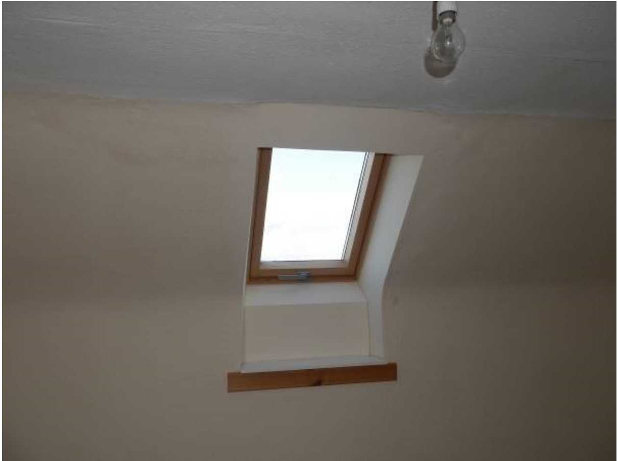
Illustration 28-Interior of gable window in upstairs bedroom (11) looking South
