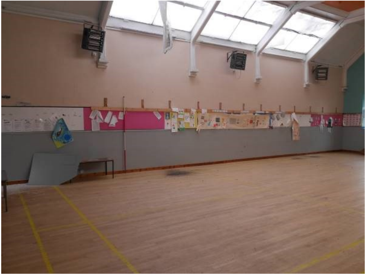
Illustration 50- Northern elevation of Main Hall in Building B looking North
