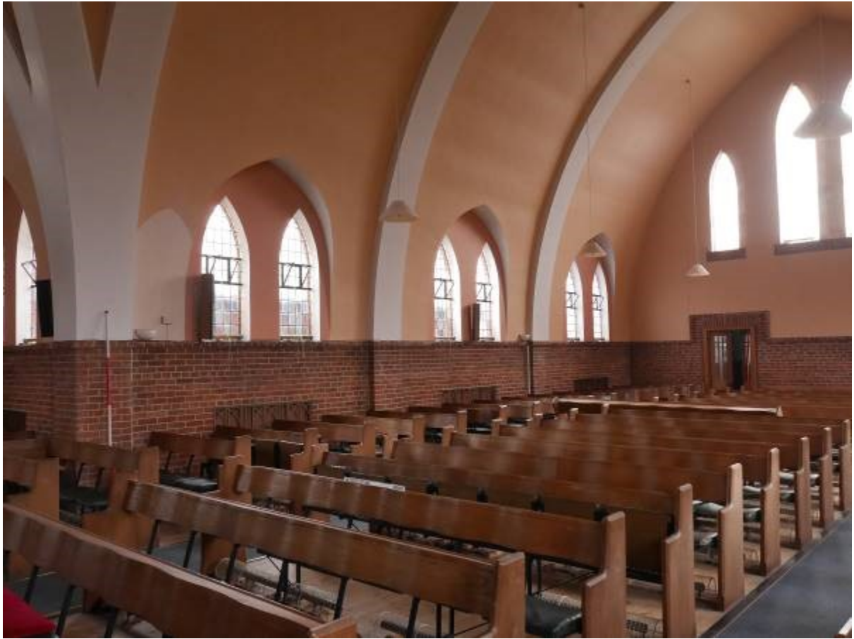
Illustration 25- Eastern elevation of Nave in Building A looking East
