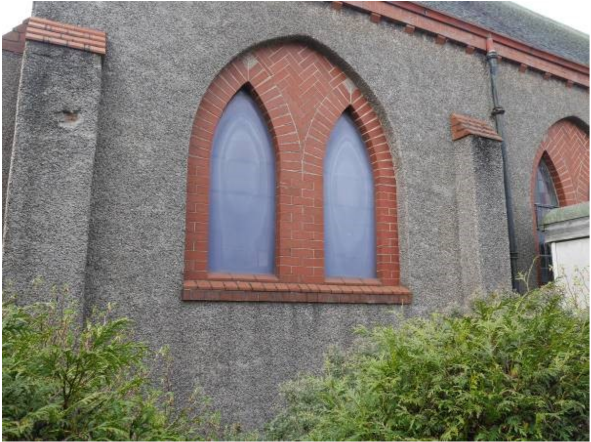
Illustration 14- Detail of windows in Eastern elevation of Nave (Building A)
