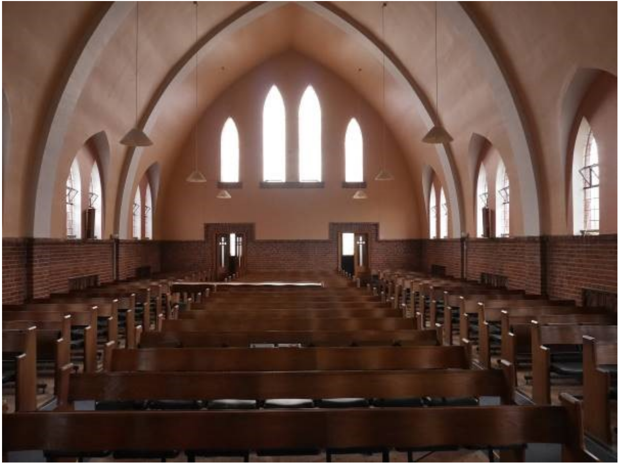
Illustration 23- General view of Nave in Building A looking South
