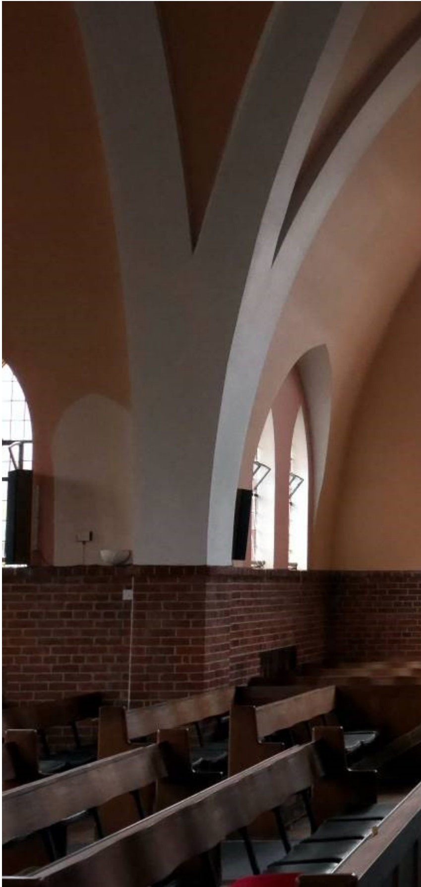
Illustration 28- Southern elevation of Western transept
