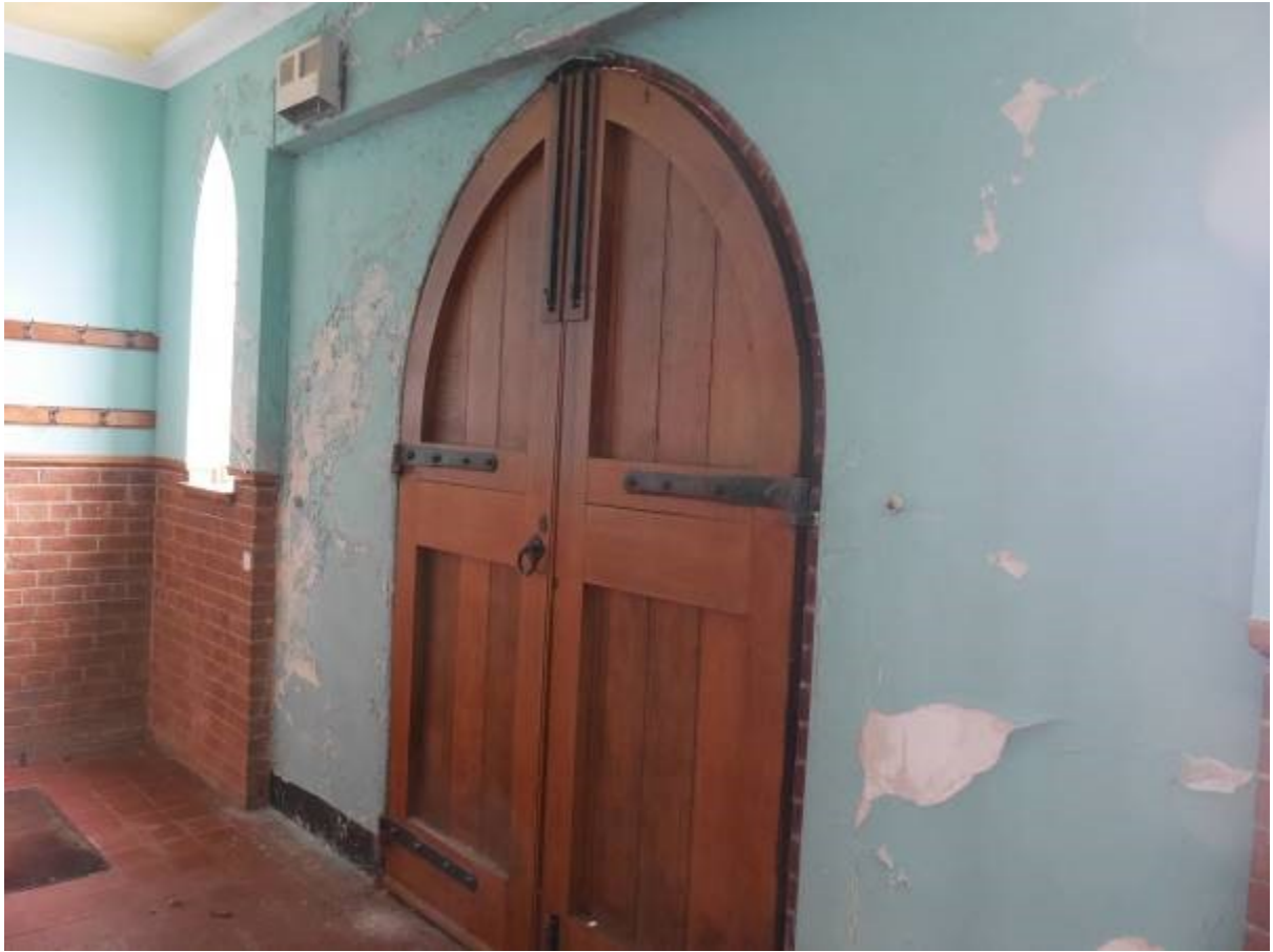
Illustration 22- Main doorway into Building A
