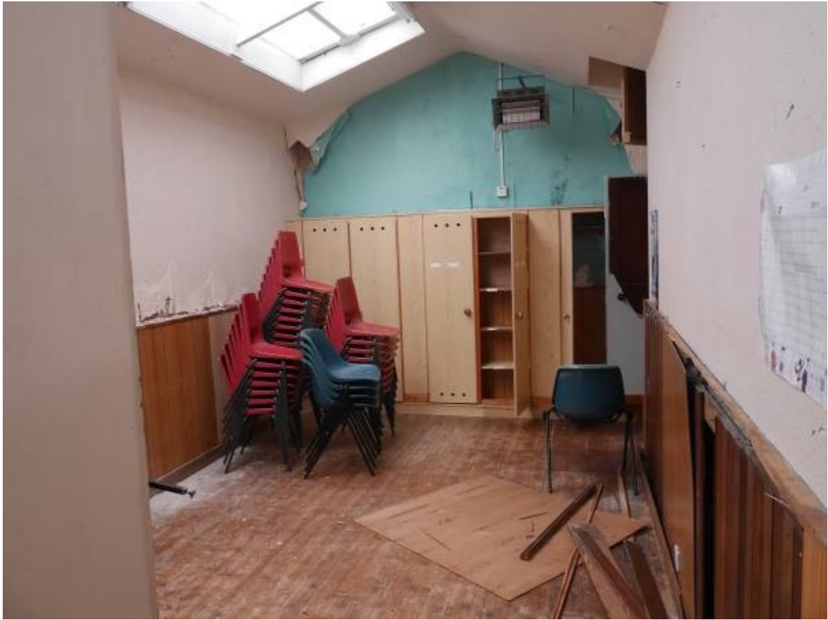
Illustration 56- Classroom in Building B looking North
