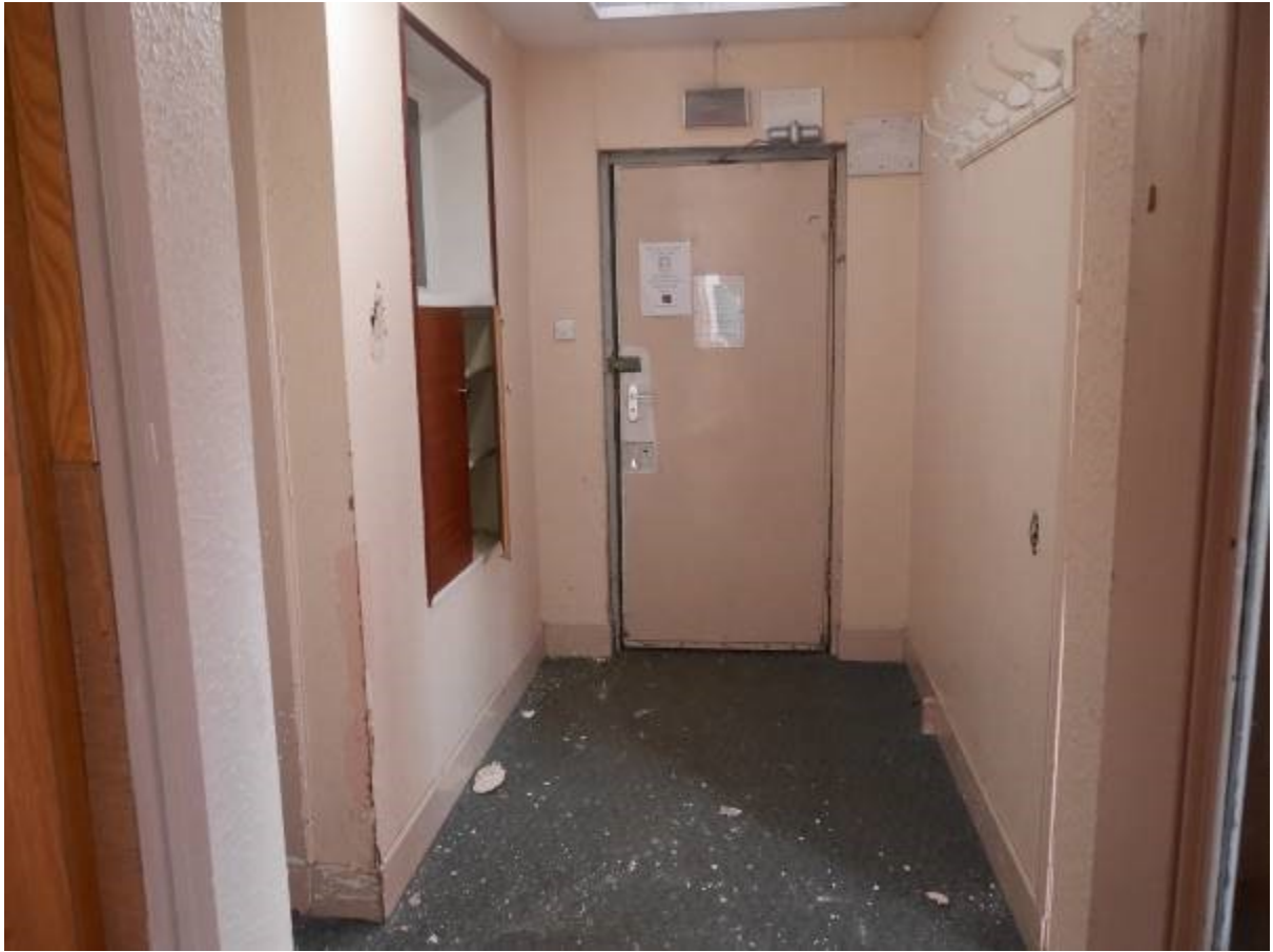
Illustration 59- Entrance hall in Building B looking South
