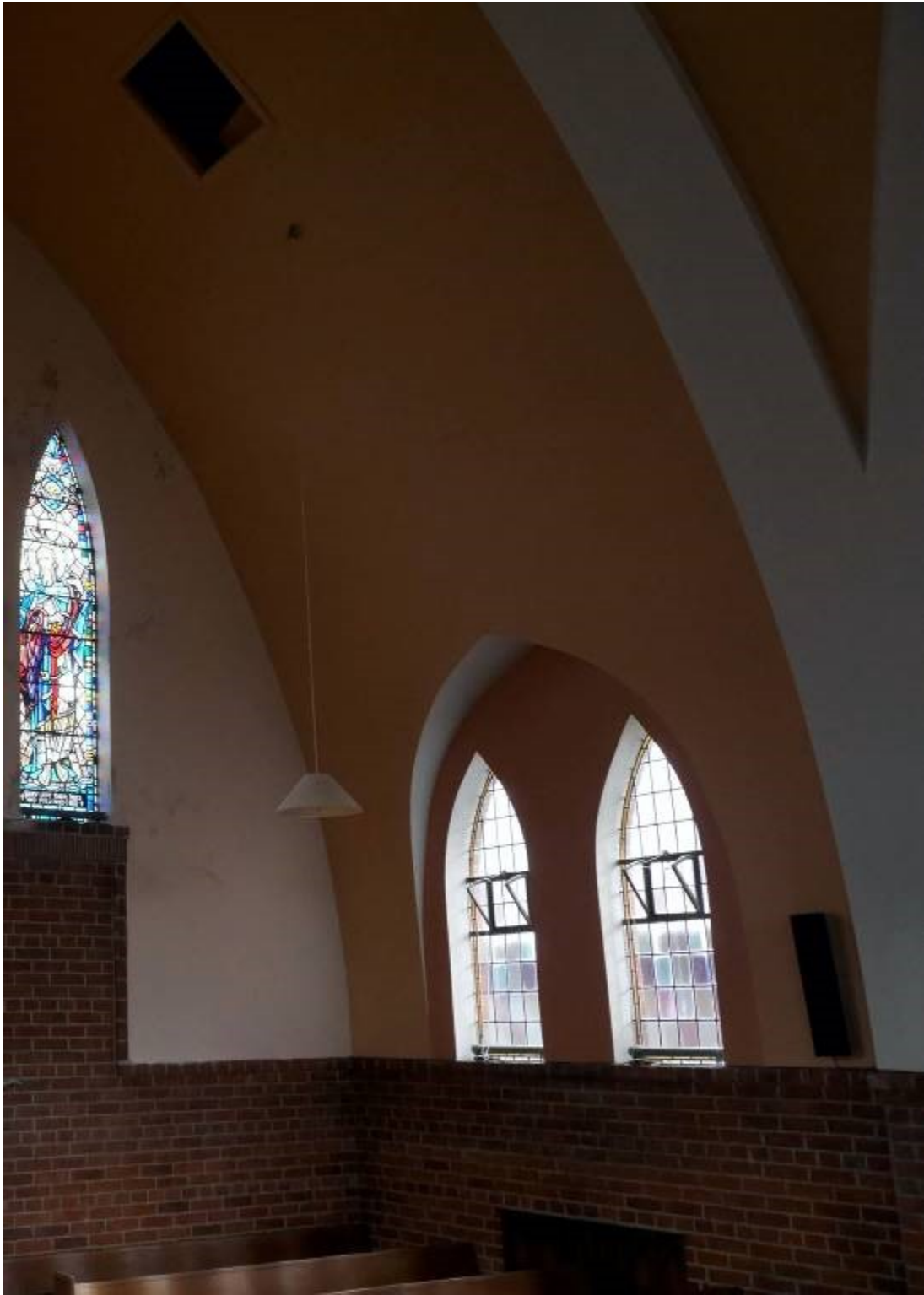
Illustration 33- Southern Elevation of Eastern transept
