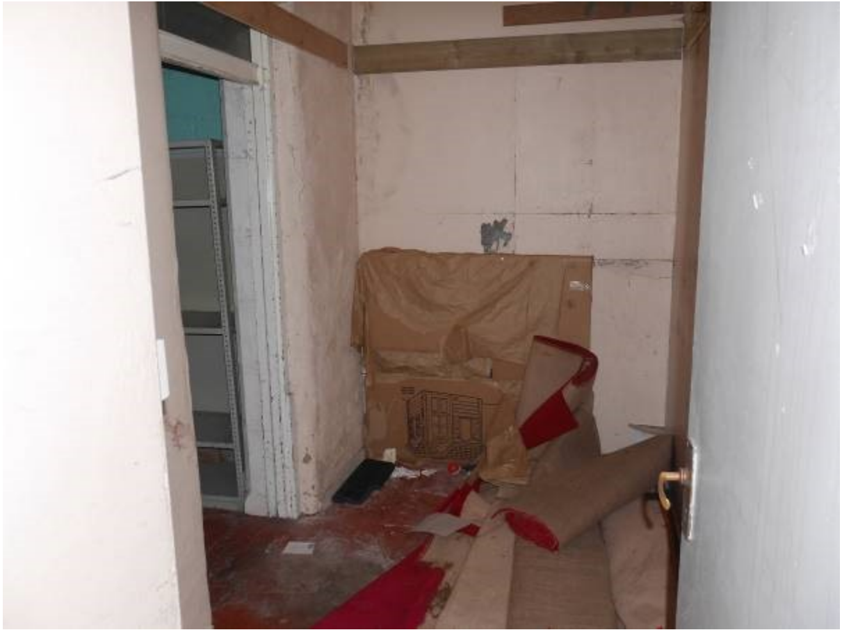
Illustration 54- Former Boiler House in Building B looking South
