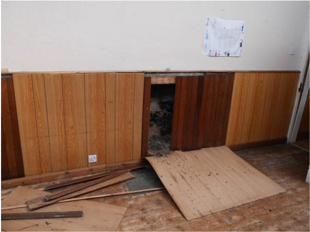
Illustration 57- Fireplace behind panelling in Eastern wall of classroom
