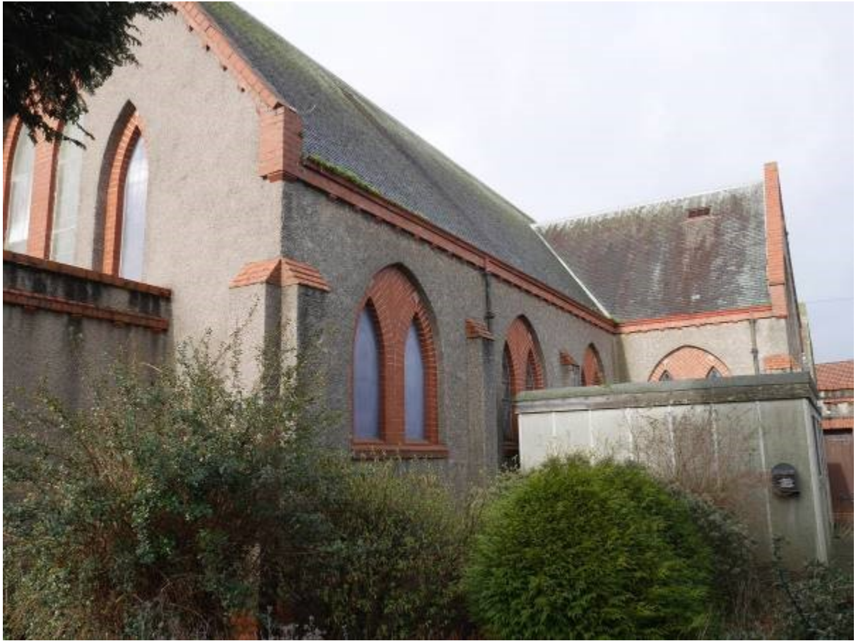
Illustration 13- Eastern Elevation to Building A showing location of Porta-cabin
