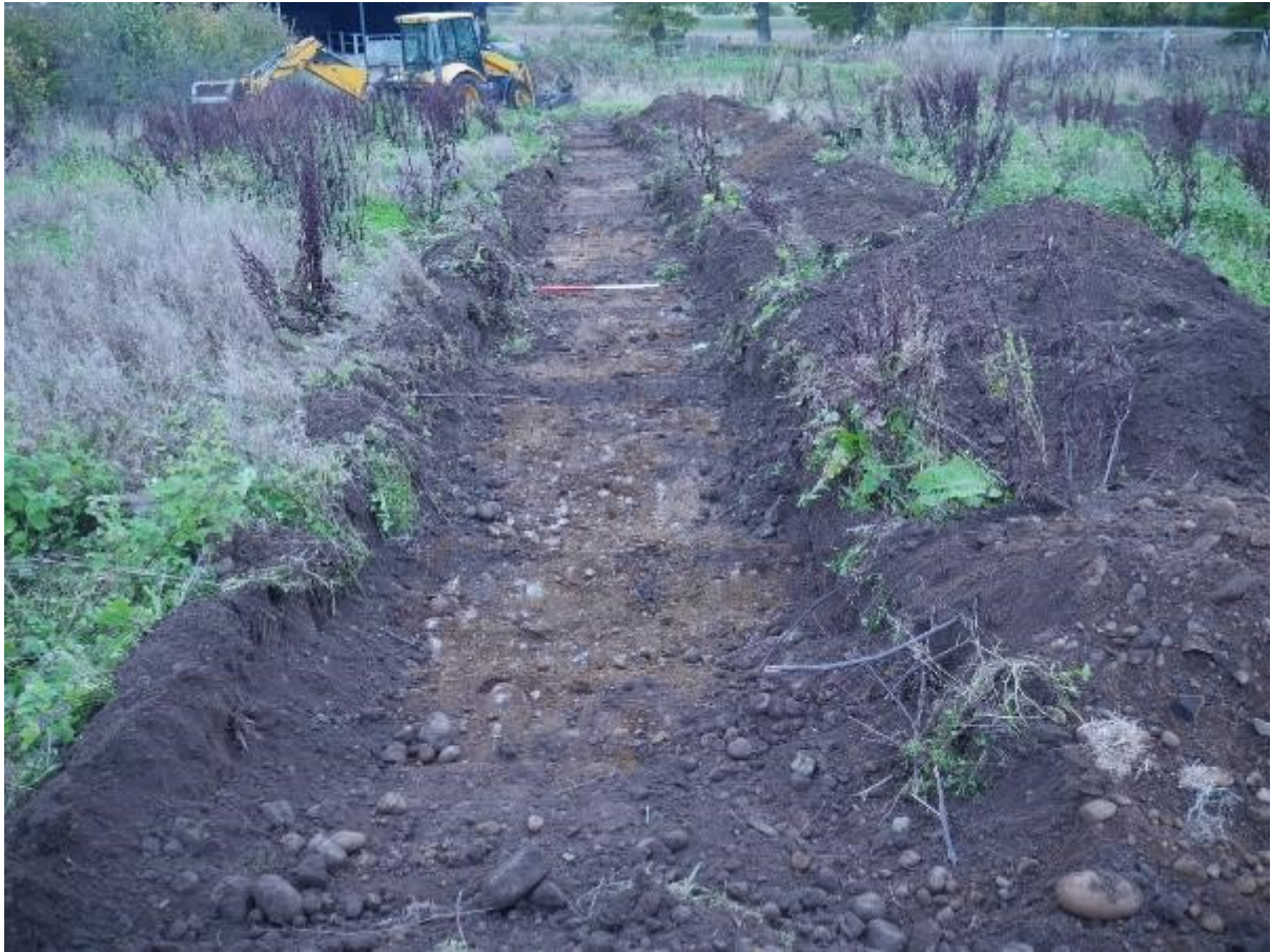
Illustration 21- Trench 11 fully excavated looking East
