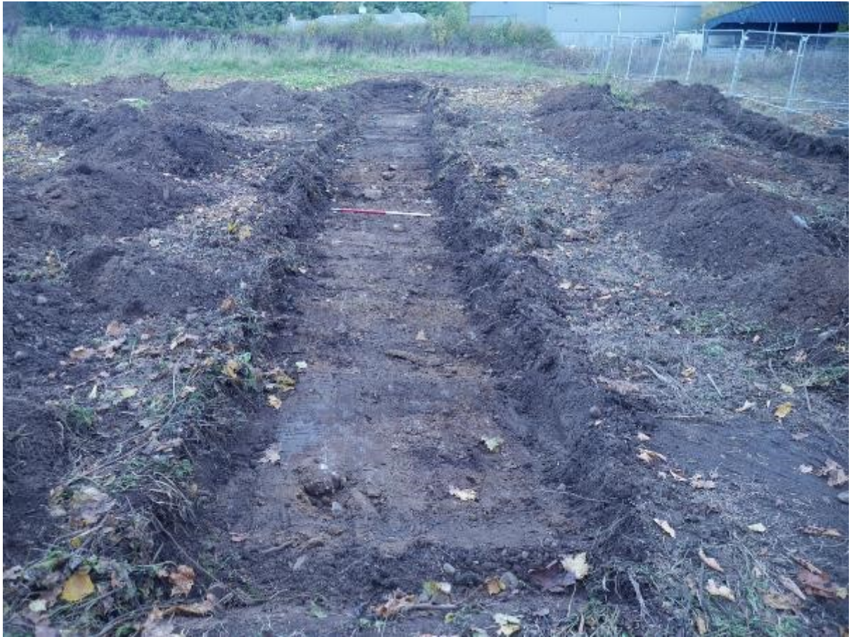
Illustration 8- Trench 6 fully excavated looking North East
