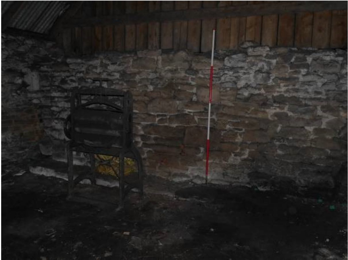
Illustration 18- Southern internal elevation of Steading 1 showing slightly wider wall foundation, mangle and base of wooden roof support.
