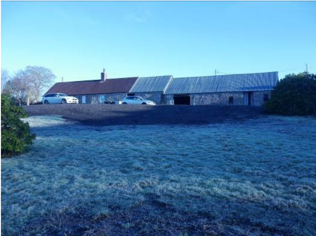
The Cottage, Collace looking East (buildings to be demolished have tin roof)
