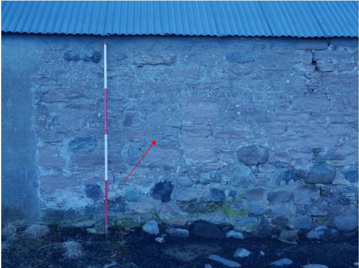
Illustration 9- Detail of Western elevation showing blocked window in Steading 2 (red arrow)
