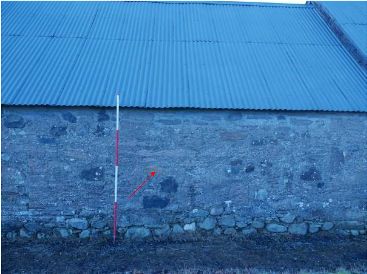
Illustration 14- Visible blocked window in Western elevation to building
