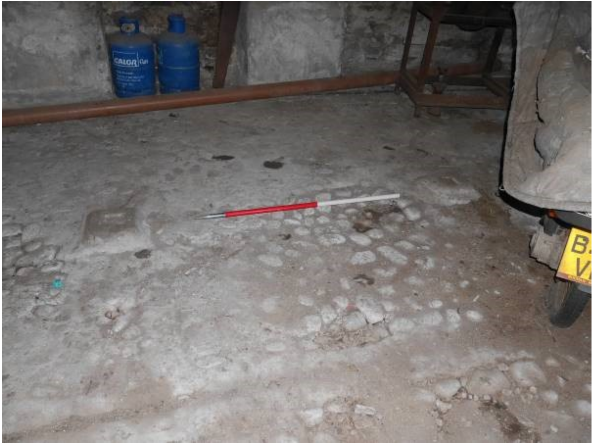
Illustration 30- General view of floor in Steading 3 looking East showing both socketed stones in the floor
