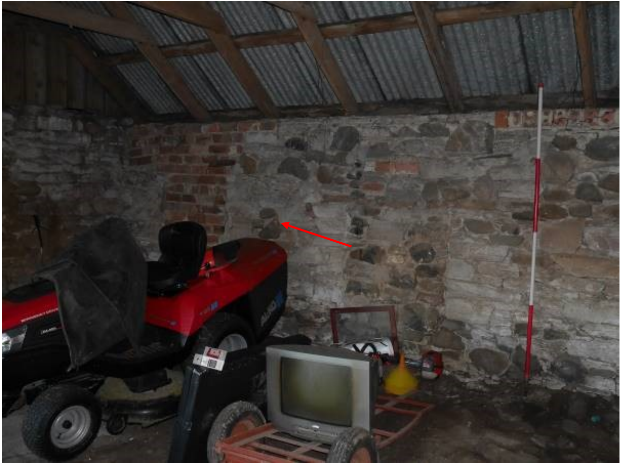
Illustration 22- Eastern elevation of Steading 2 showing third blocked window (red arrow)
