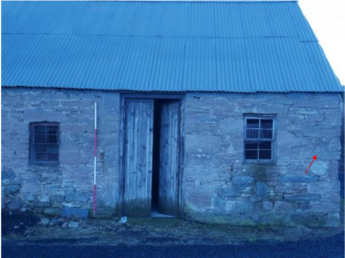
Illustration 10- Detail of southern end of Western elevation, alternate shaped quoins at corner marked with red arrow
