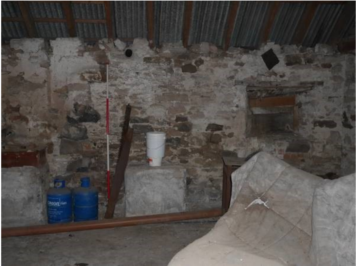
Illustration 26- Eastern internal elevation of Steading 3 showing blocked window
