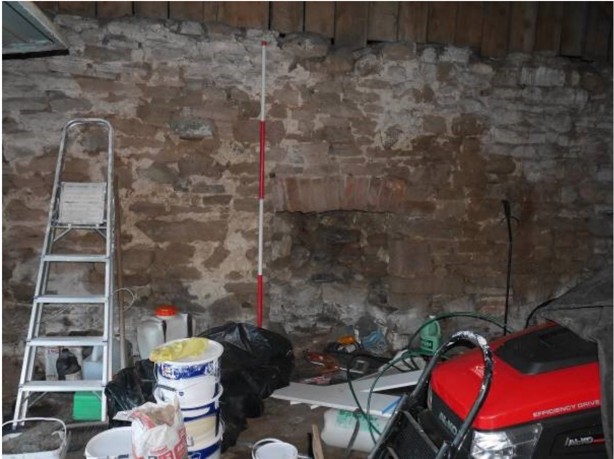
Illustration 20- Northern elevation of Steading 2 showing fireplace with brick arch and base of wooden roof support
