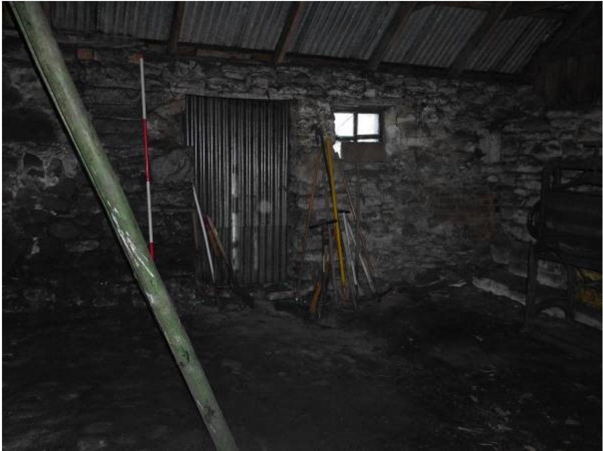
Illustration 17- Eastern internal elevation of Steading 1 showing doorway and window
