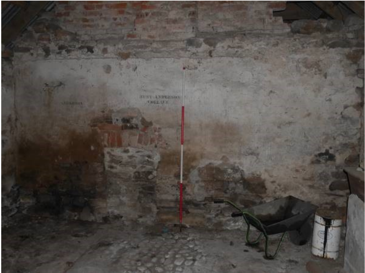
Illustration 25- Northern internal elevation of Steading 3 showing blocked fireplace, stencilled names on wall face and brick support for roof
