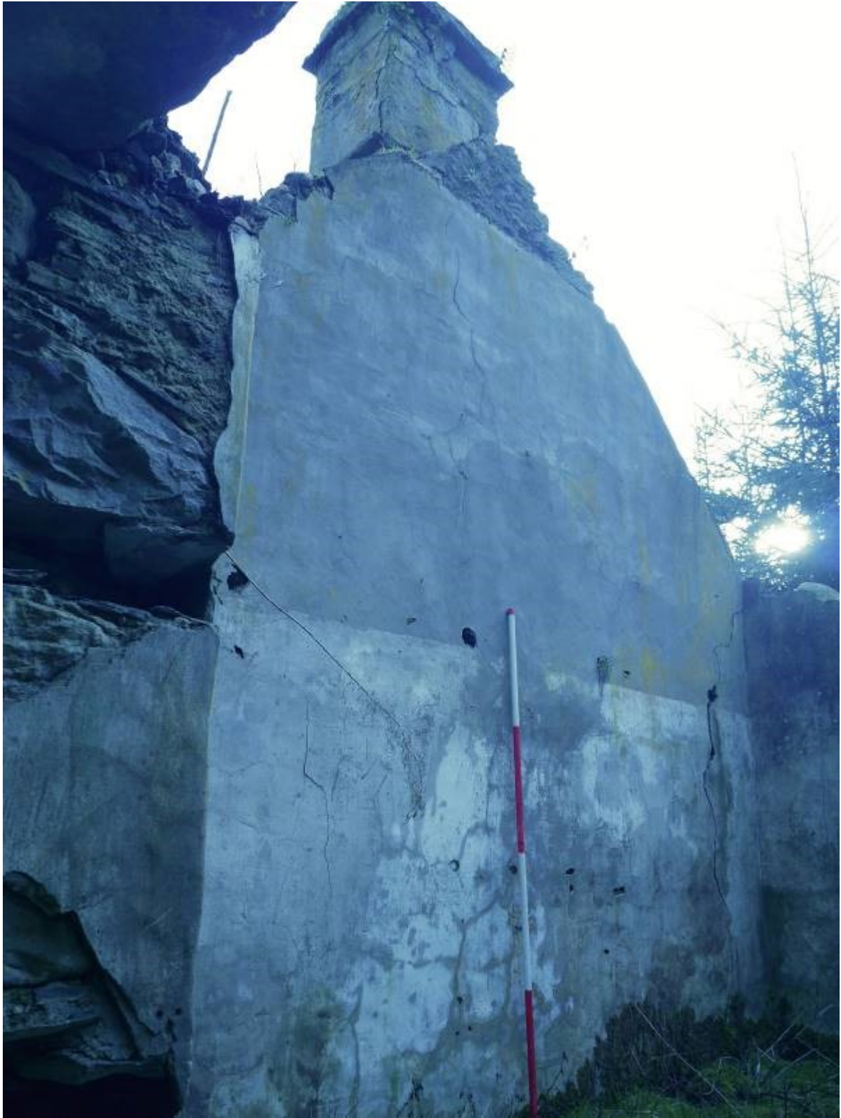
Illustration 19 – Western elevation of Building 2 visible behind butt jointed Building 3
