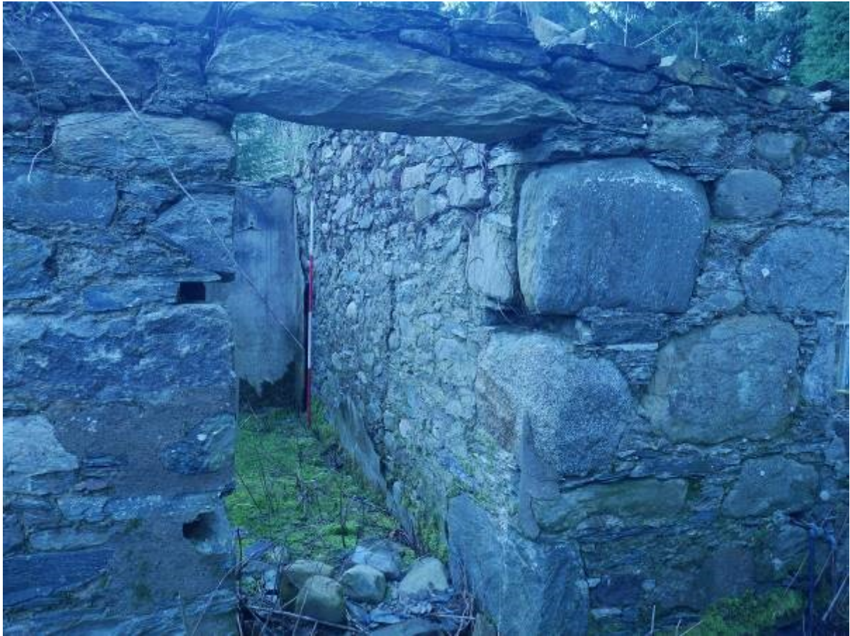
Illustration 26 – Internal Eastern elevation of Room 3a in Building 3
