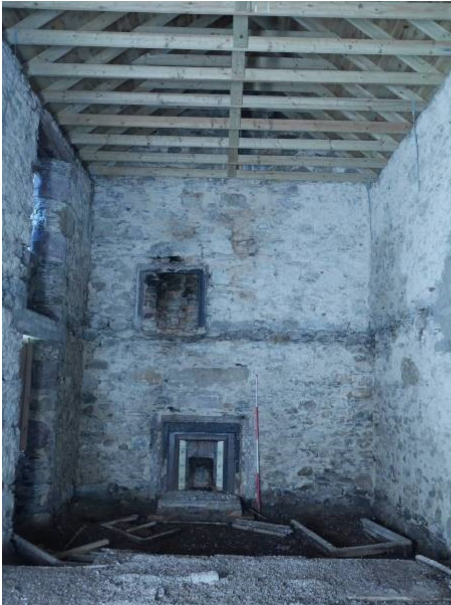
Illustration 11 - Internal Northern elevation of Building 1
