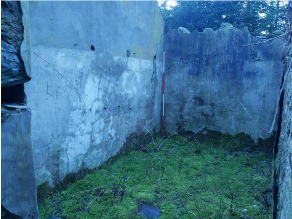
Illustration 25 – Plastered internal Northern and Western elevations of Room 3a in Building 3
