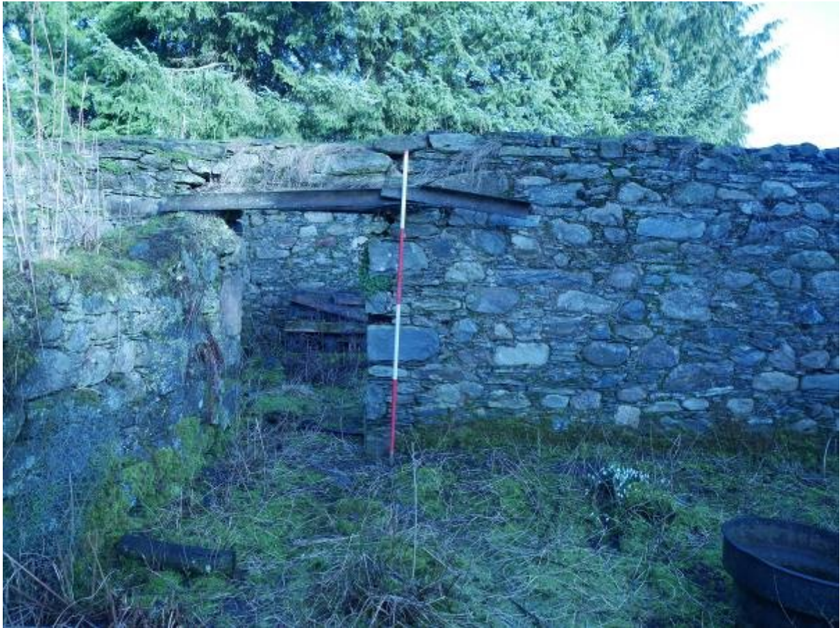
Illustration 24 - Southern Elevation of Building 3 showing doorway into Room 3b
