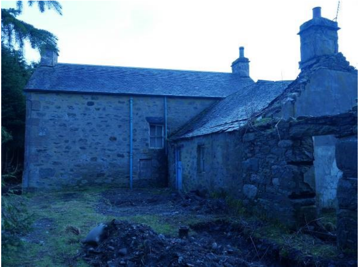
Illustration 9- Western elevation of Building 1 showing Buildings 2 and 3 built against it.
