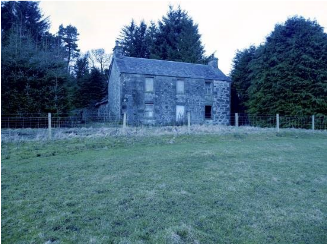
Building 1 at Mucklarie Farmhouse from the East
