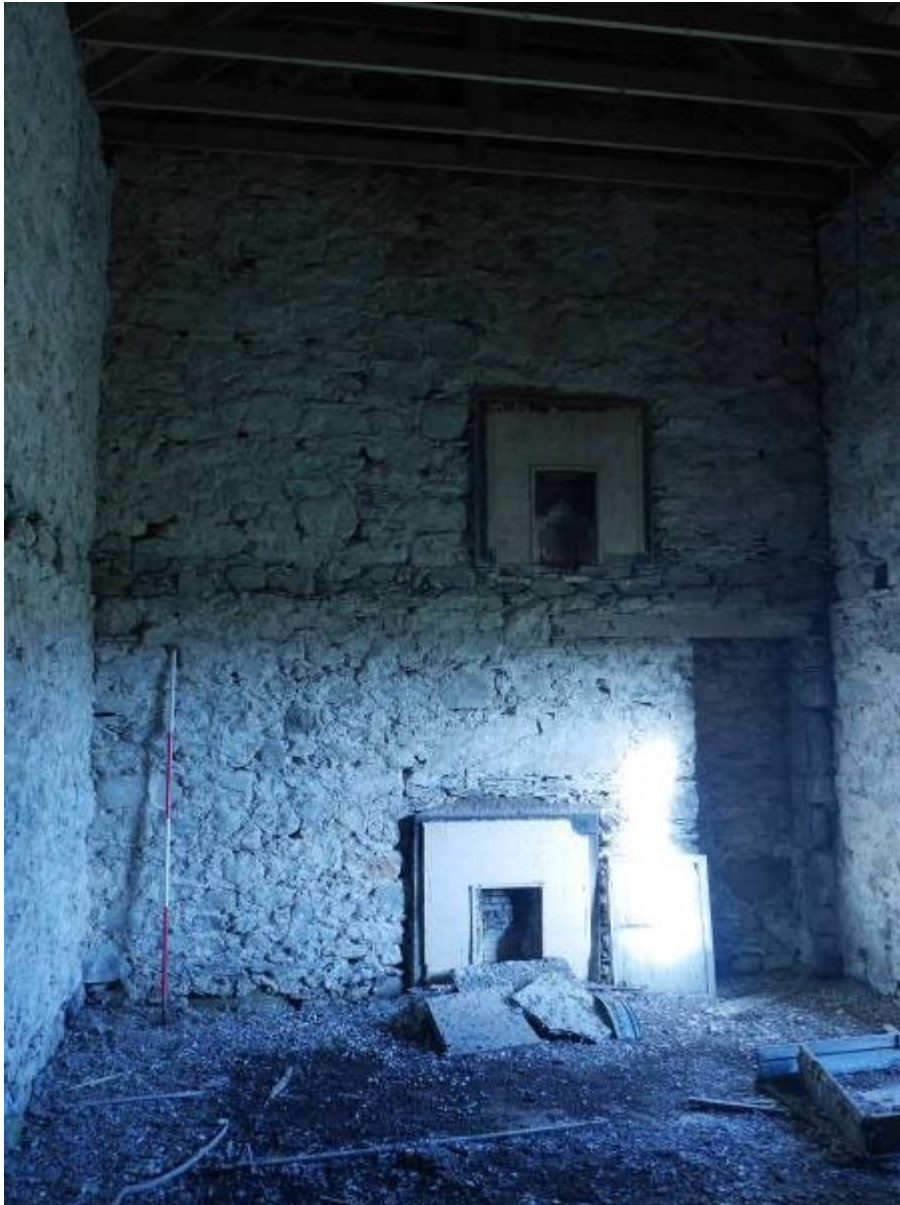
Illustration 14- Southern internal elevation of Building 1 showing fireplaces on first and ground floor level.
