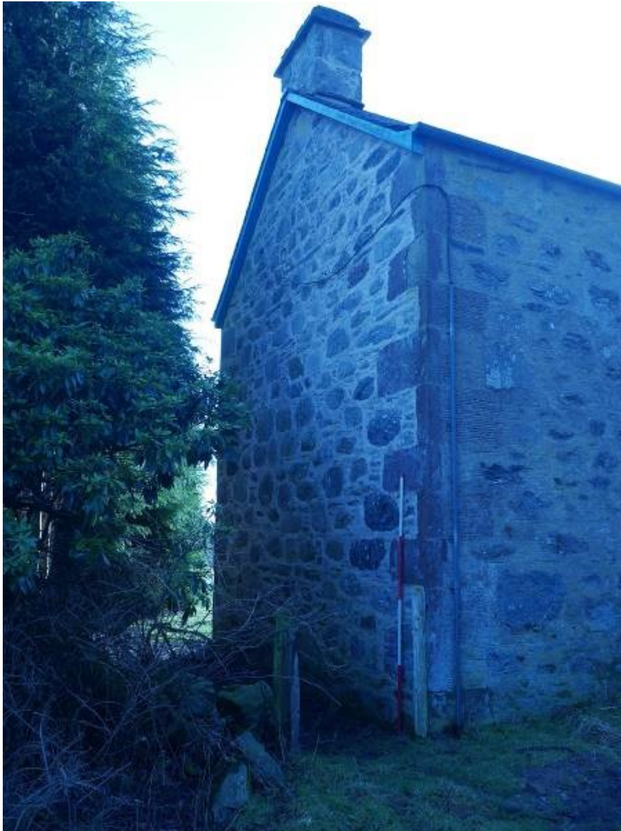
Illustration 7- Northern elevation of Building 1
