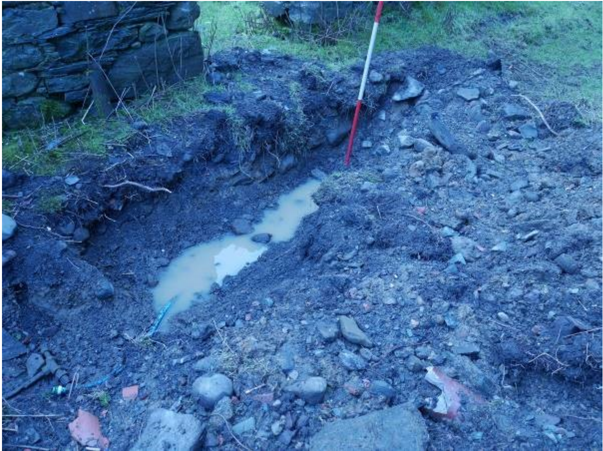
Illustration 34 – General view of machine dug trench 2
