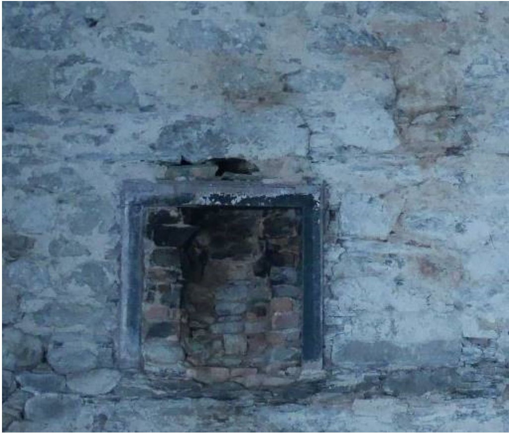
Illustration 12- Fireplace at first floor level in internal Northern elevation of Building 1
