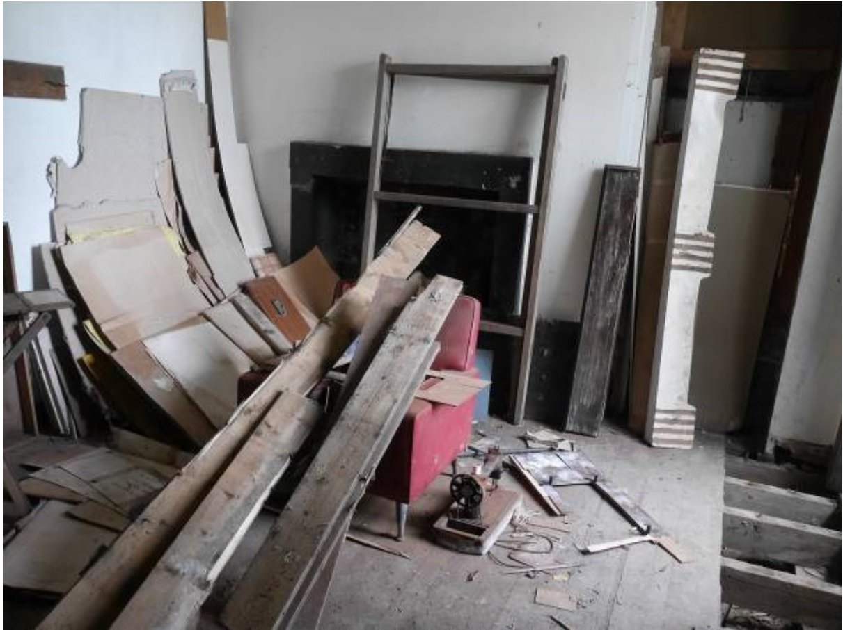
Illustration 16 – Building A Room 1 (backroom) showing fireplace in West wall
