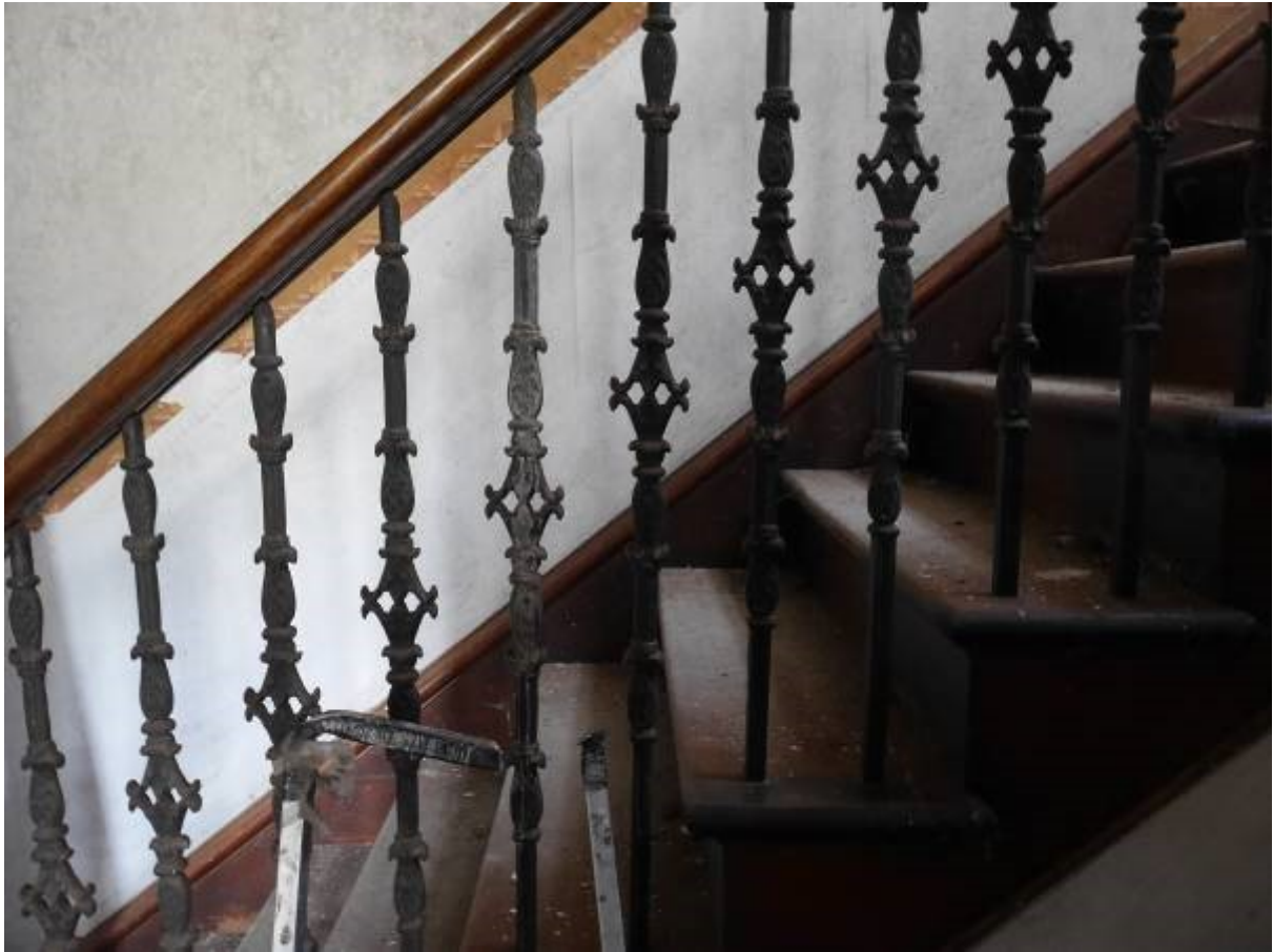
Illustration 26 - Building A detail of decorated cast iron balustrade on staircase to first floor
