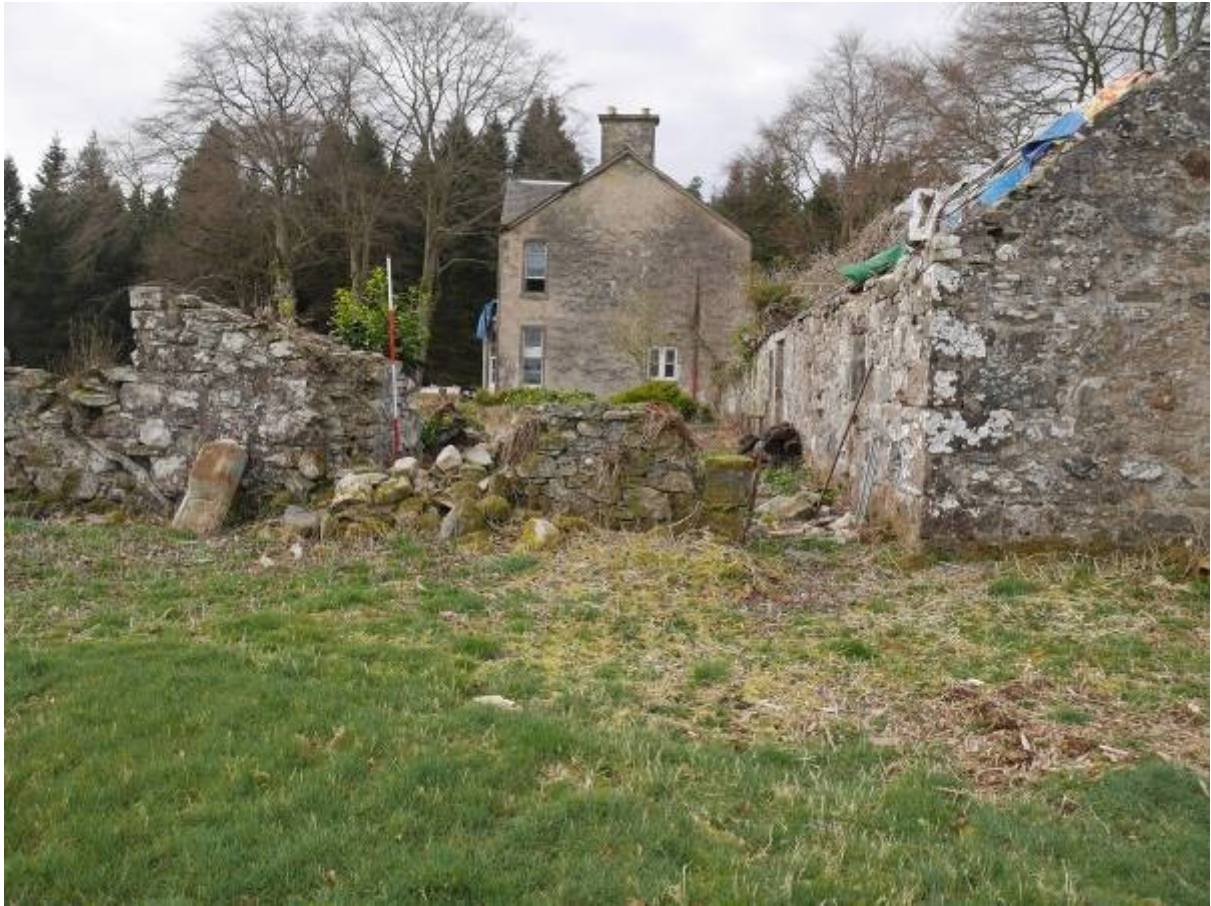
Illustration 44 - Buildings B and C looking West with Building A in background
