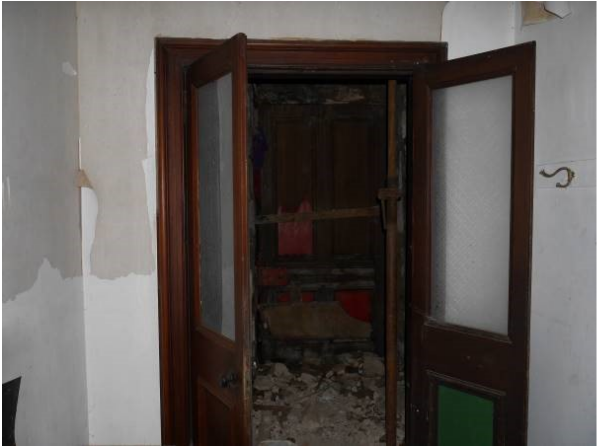
Illustration 23 - Building A small entrance lobby for main entrance looking South
