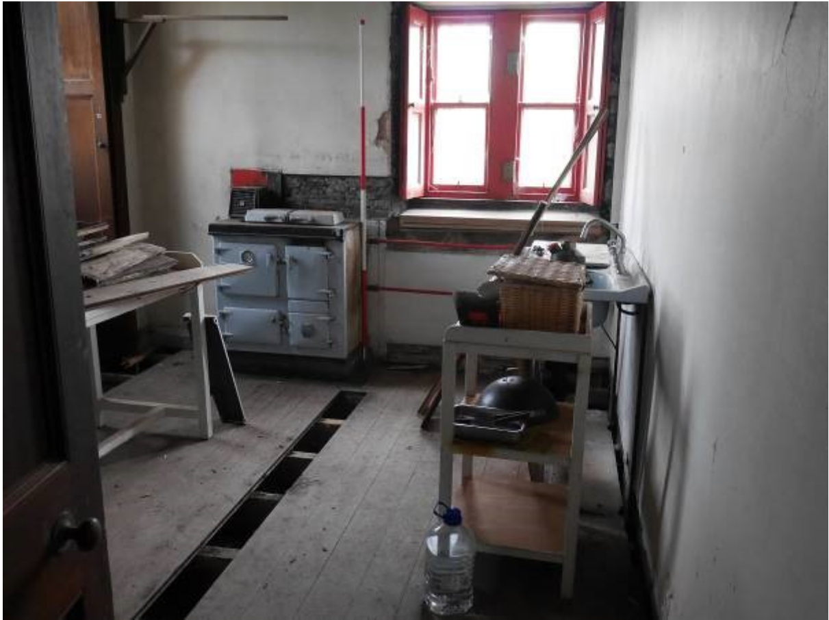
Illustration 20 - Building A Room 3 (Kitchen) looking East
