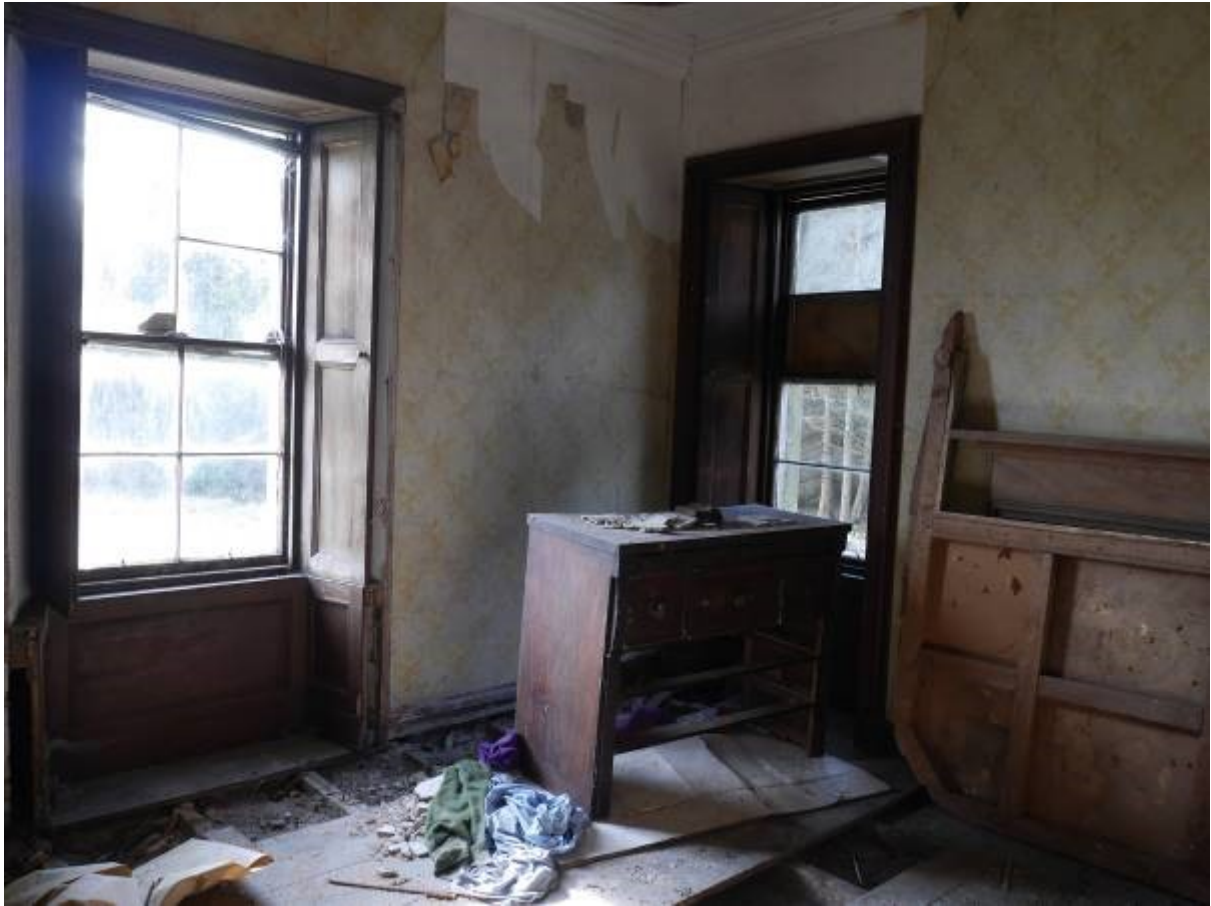
Illustration 33 - Building A Room 10 (Western bedroom) showing shuttered windows
