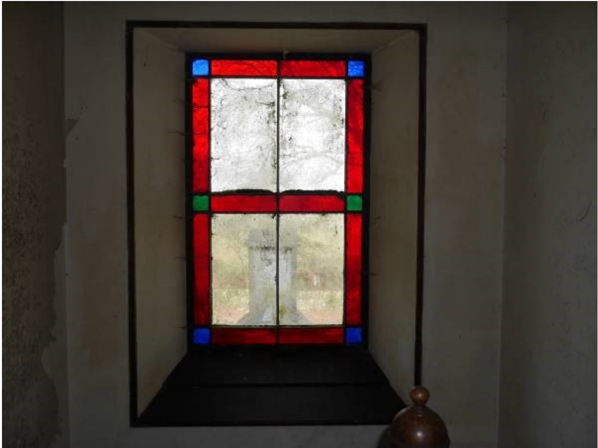
Illustration 27 - Building A coloured leaded glass window half way up staircase to first floor
