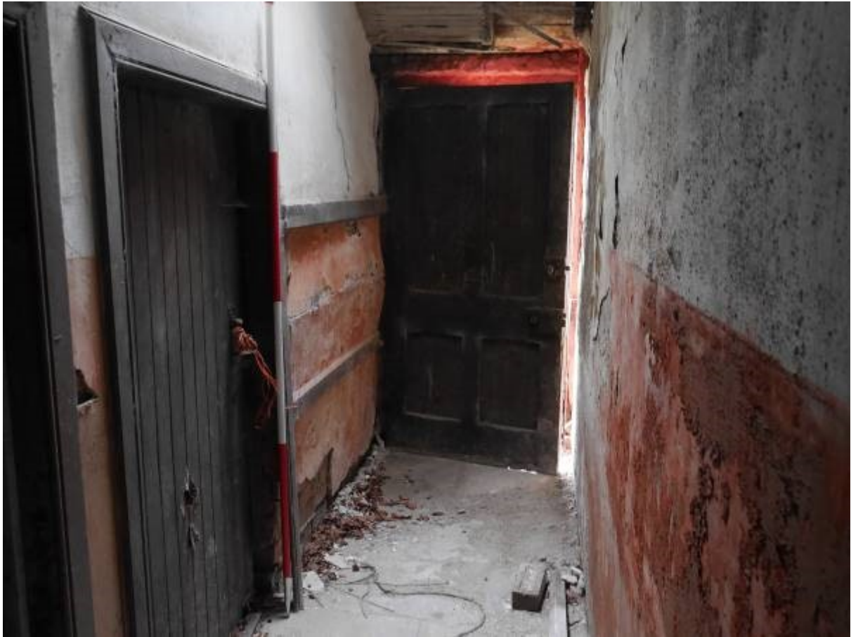
Illustration 14 - Corridor in Boiler House/Stores looking East
