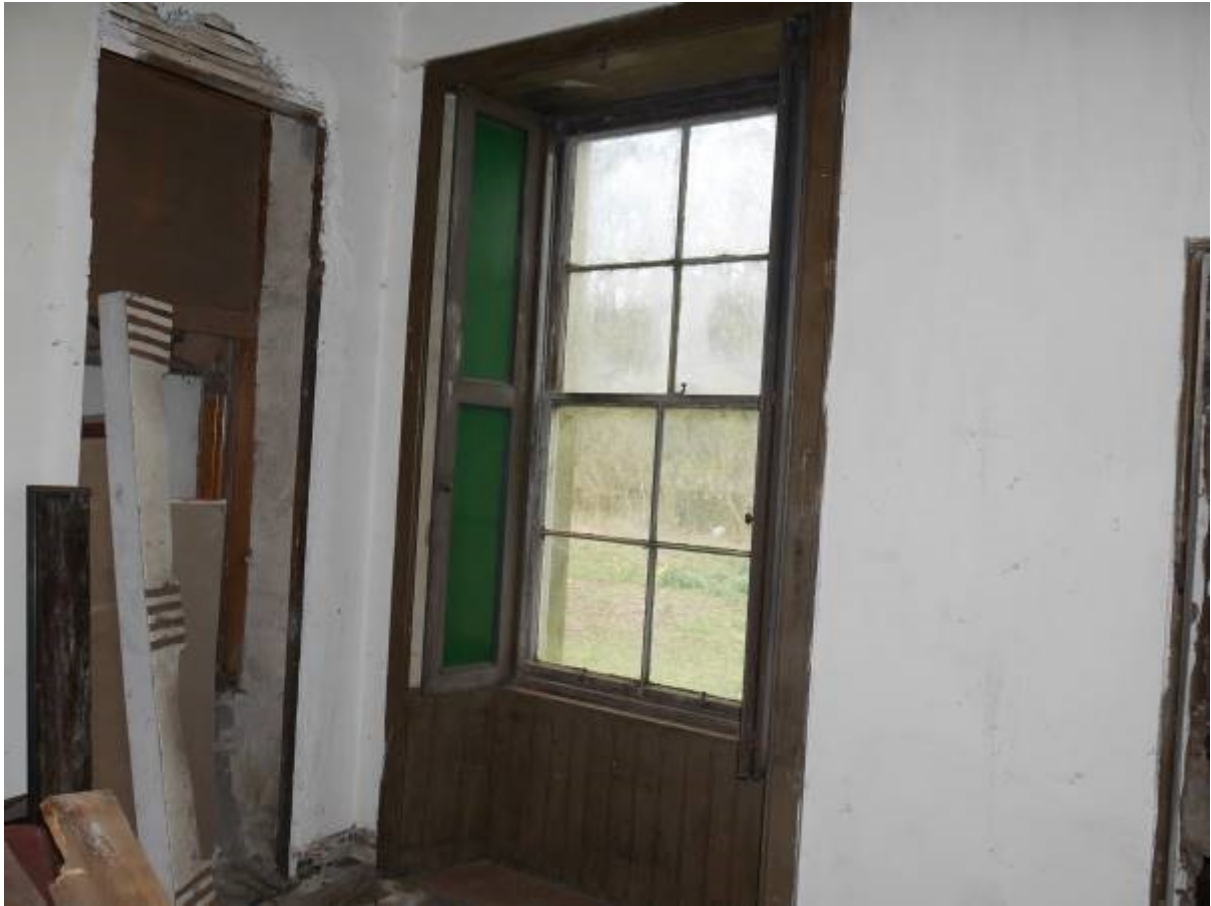
Illustration 15 - Building A Room 1 (backroom) shuttered window in North wall
