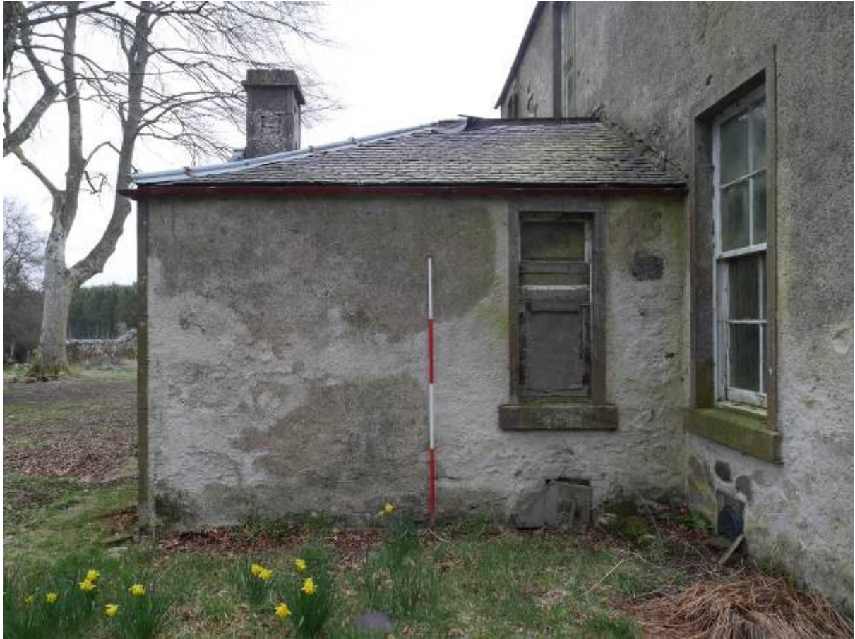
Illustration 11 - Boiler House and stores Western elevation
