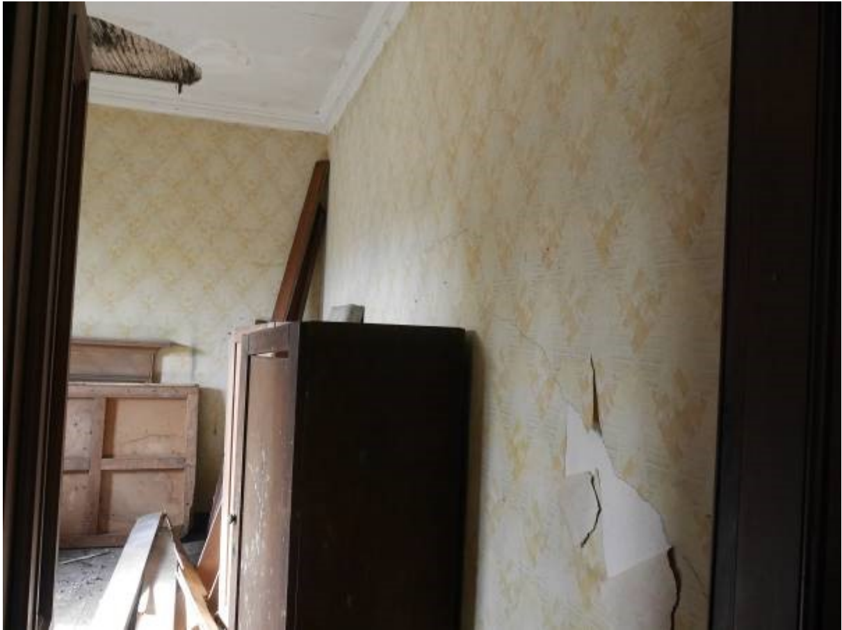
Illustration 34 - Building A Room 10 (Western bedroom) showing wallpaper and plain moulding, top of fireplace visible behind board against Western wall
