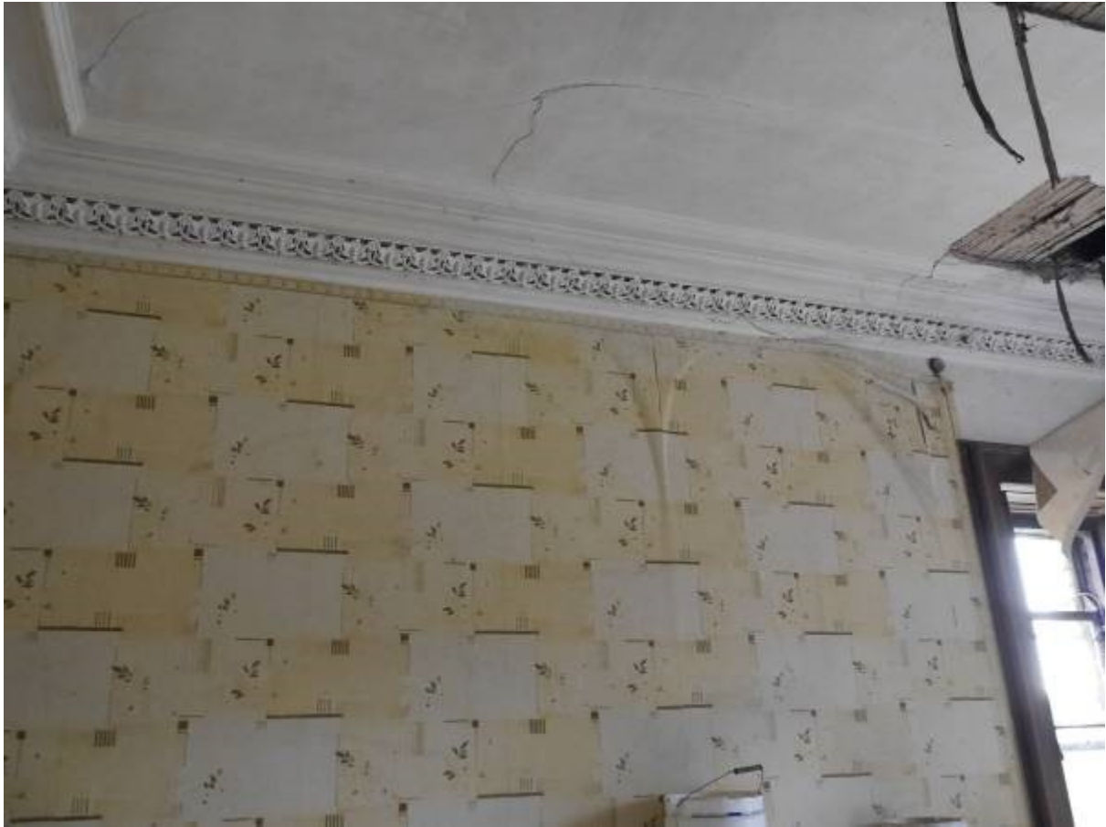
Illustration 32 – Building A Room 8 (Eastern bedroom) showing ornate moulding around ceiling
