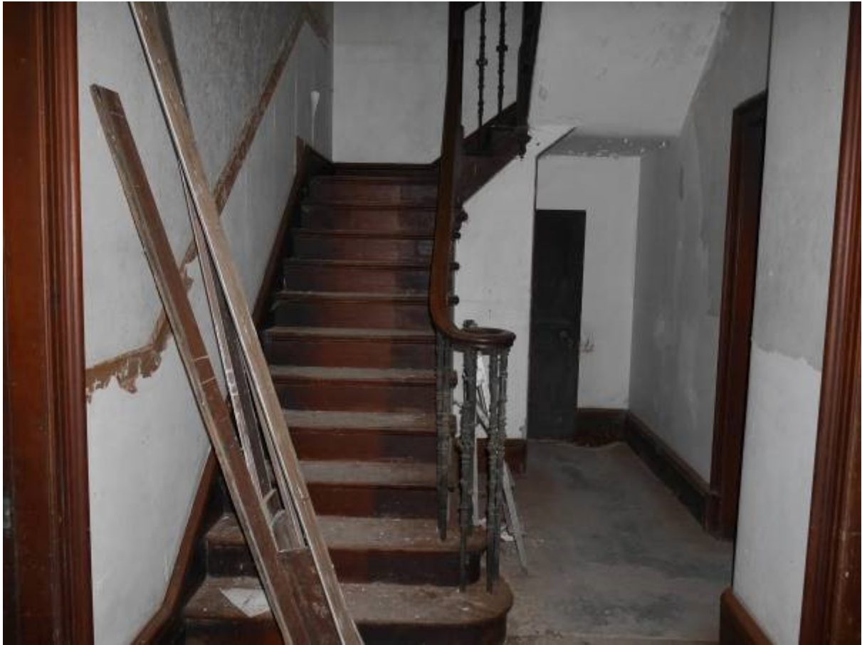
Illustration 19 - Building A ground floor lobby showing staircase to first floor
