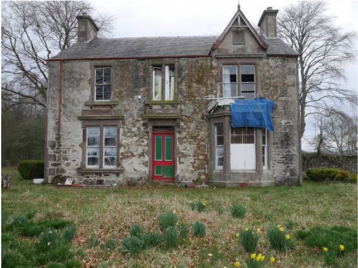
Illustration 7 - Building A Southern Elevation (note datestone of 1870 in small gable)
