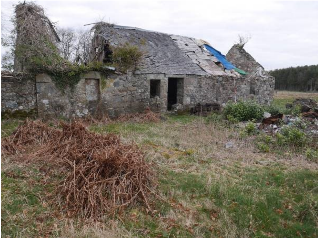
Illustration 39 - Building B Southern elevation showing visible straight joint with garden wall
