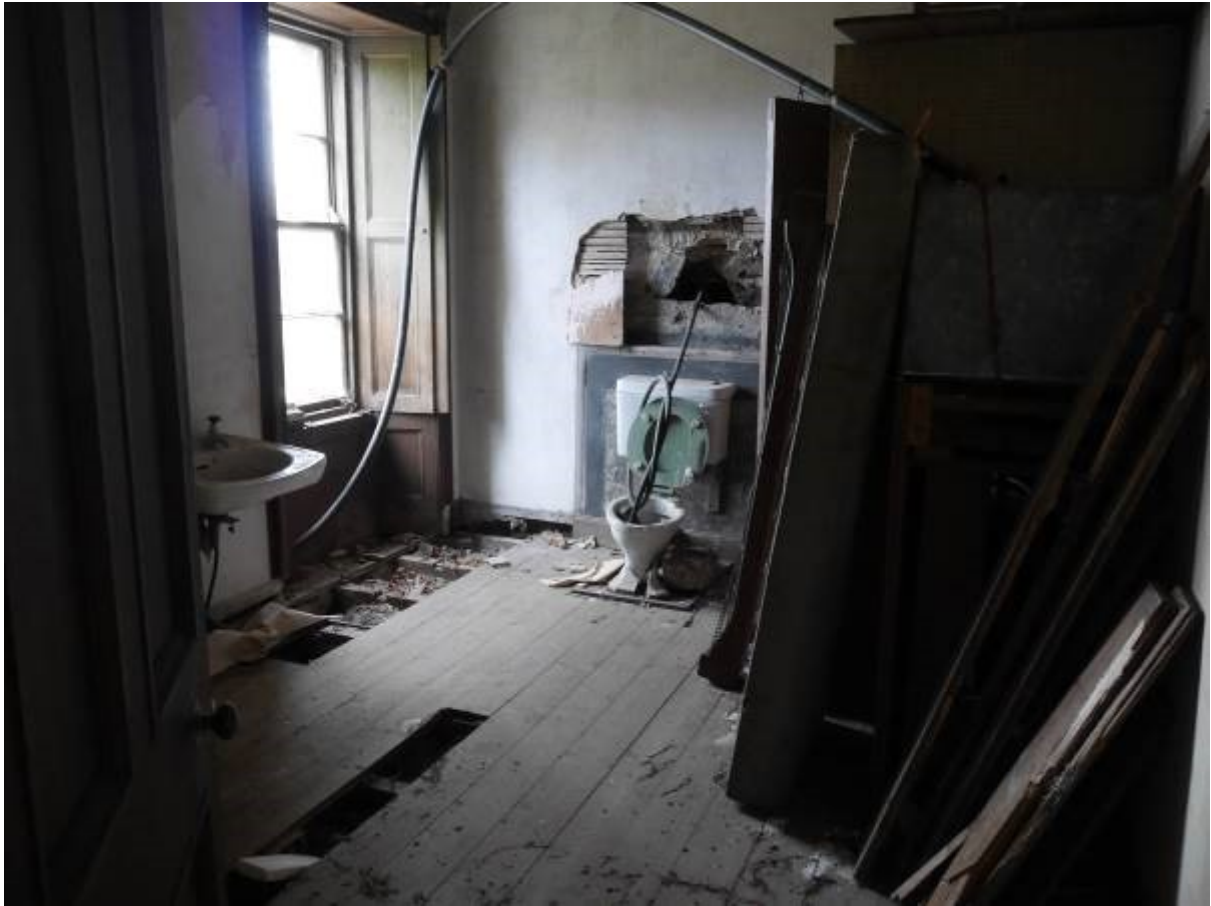
Illustration 30 – Building A Room 7 (bathroom) showing shuttered window
