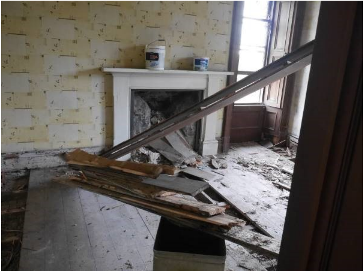
Illustration 31 - Building A Room 8 (Eastern bedroom) showing fireplace in East wall
