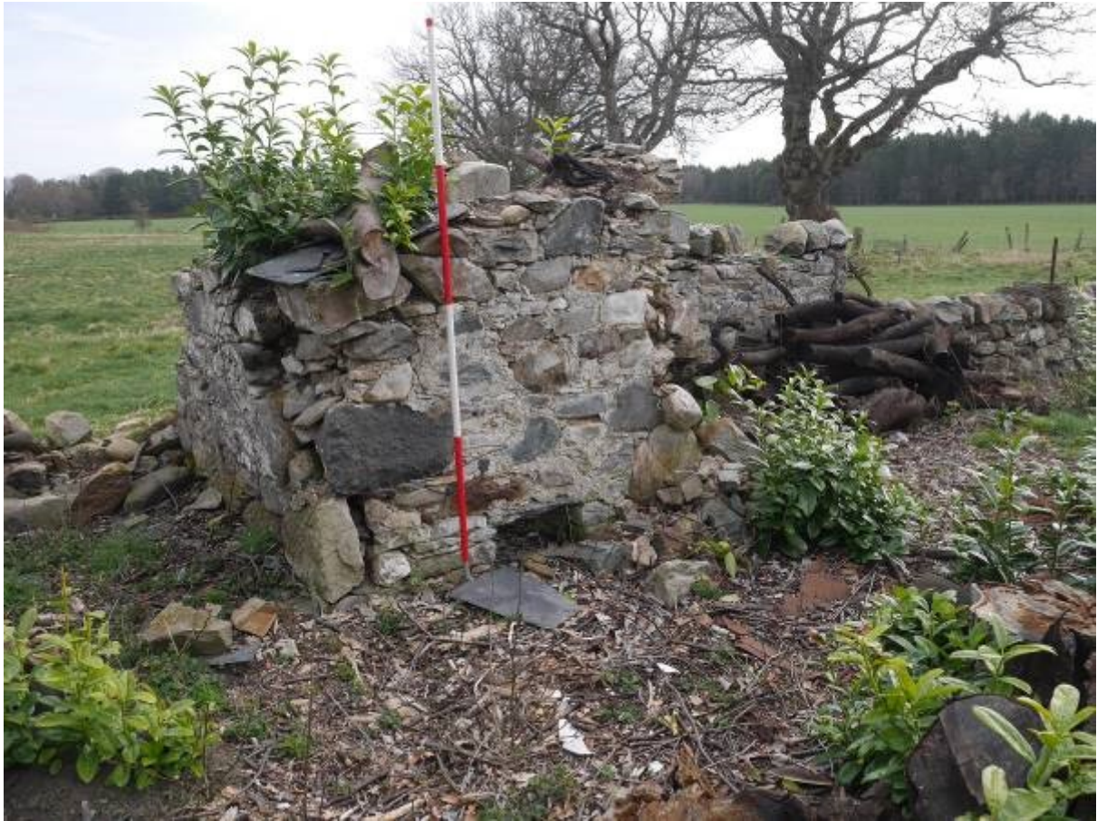
Illustration 43 - Building C Western elevation showing ventilation hole at base of wall
