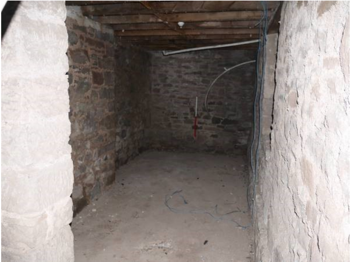
Illustration 12 – South Western section of tollhouse basement
