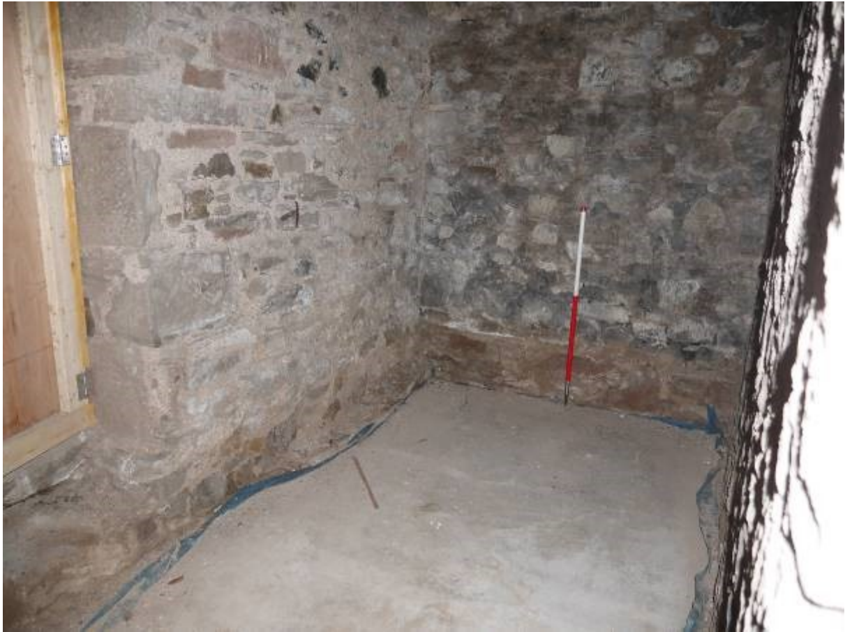
Illustration 11 – Northern section of basement, entrance door visible to left
