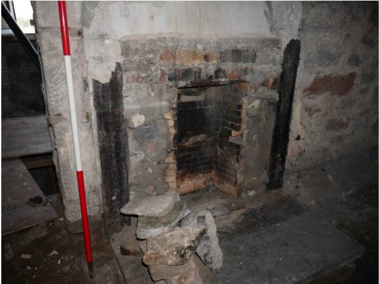
Illustration 22 – Fireplace on North Eastern side of wall in centre of ground floor of tollbooth
