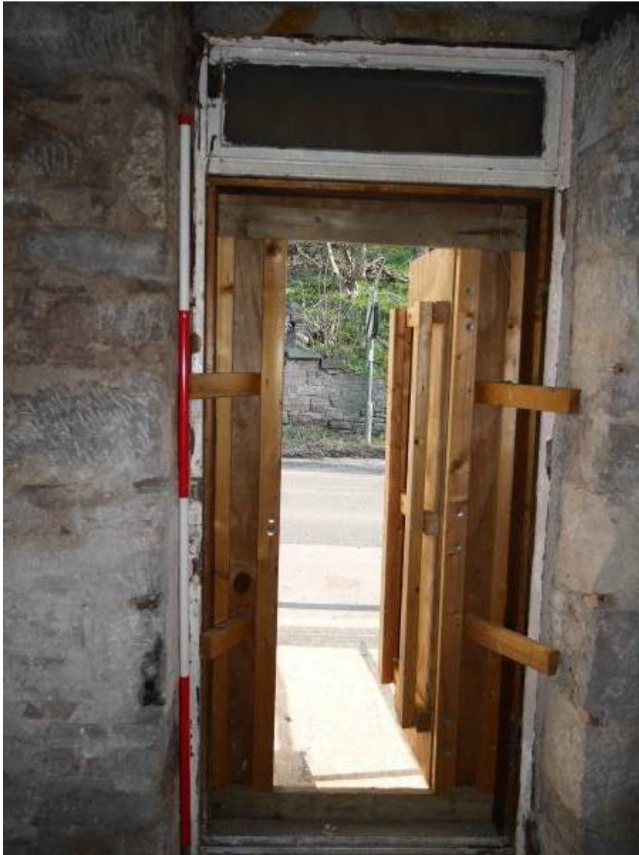
Illustration 21 - Doorway into tollhouse from road level in internal North Eastern elevation
