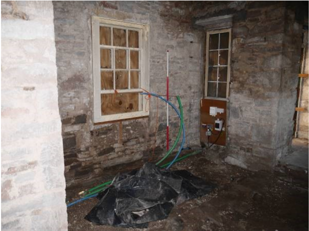
Illustration 20 – General view of internal North Eastern elevation of portico in tollhouse
