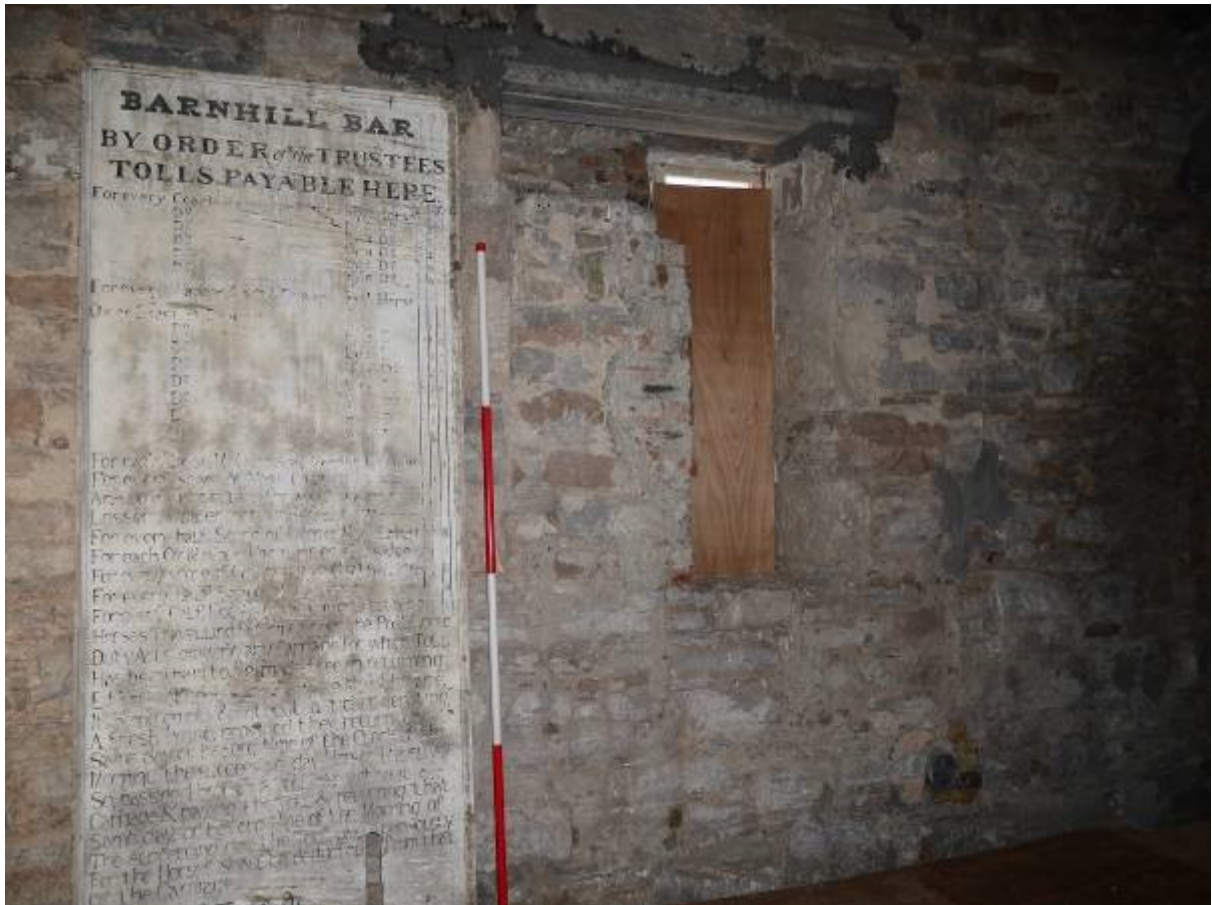
Illustration 15 – North Western internal elevation showing partially blocked window and table of dues propped against wall face
