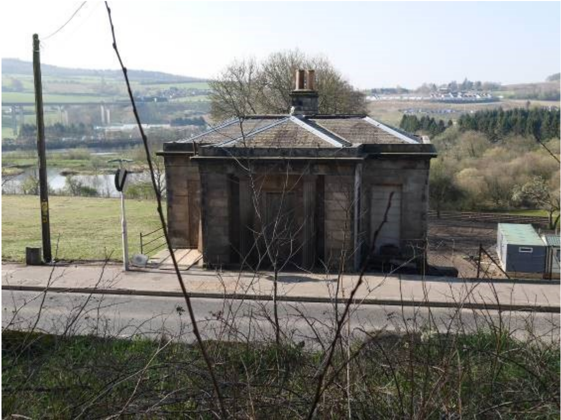
Barnhill Tollhouse looking South East (Friarton bridge visible in background)
