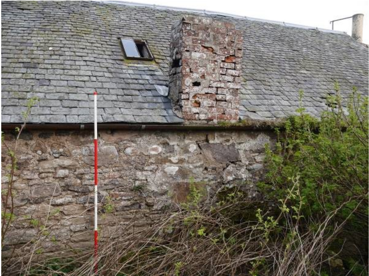
Illustration 8 – Chimney in roof line of the South Eastern elevation of Building 1
