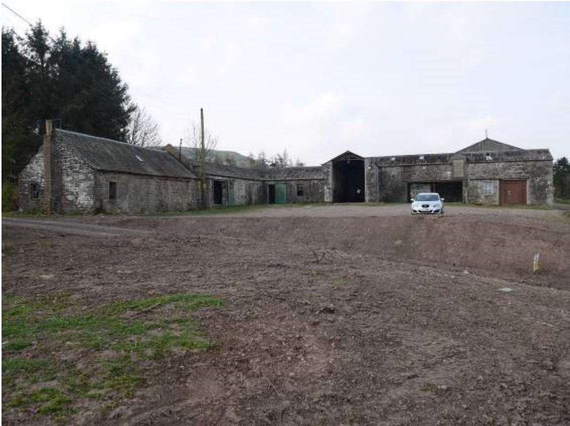
Farm steadings to be demolished at Cornhill looking South West
