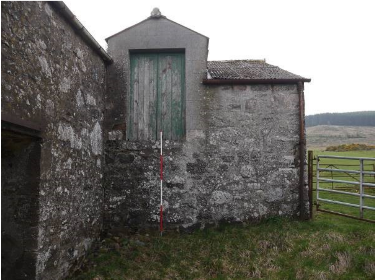
Illustration 24 – South Western elevation of Building 4 beyond its junction with Building 5
