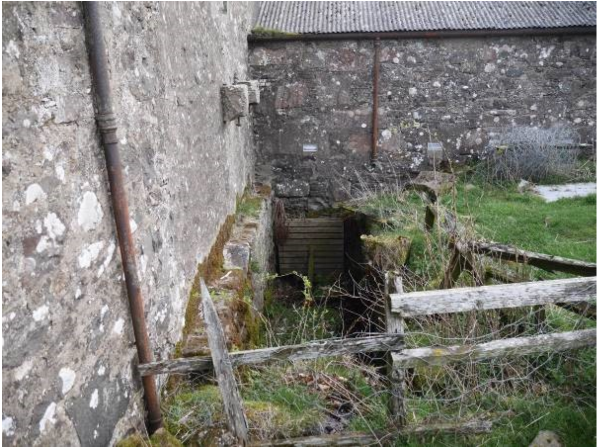
Illustration 27 – Water wheel pit against South Eastern elevation of Building 4 looking North East
