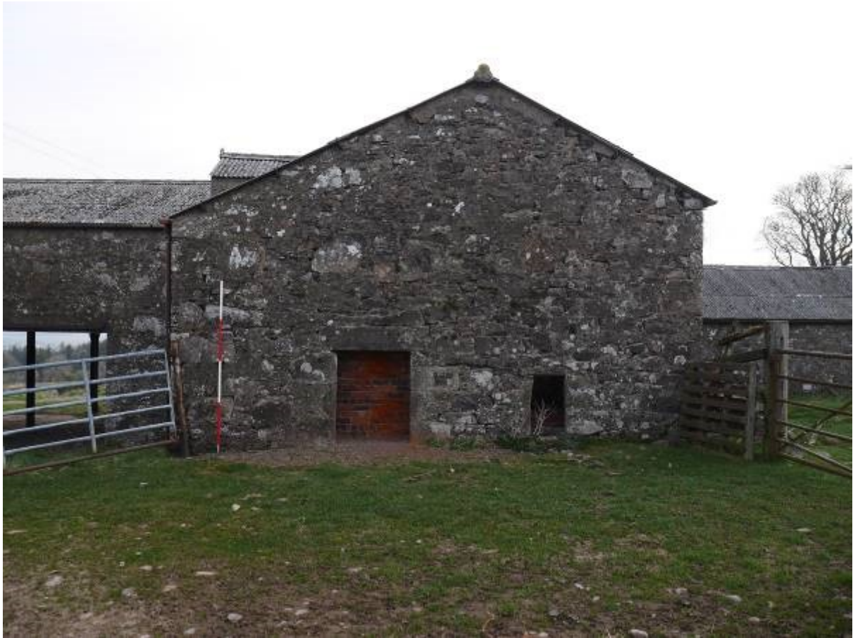
Illustration 25 – South Western elevation of Building 4 showing internally blocked doorway and window
