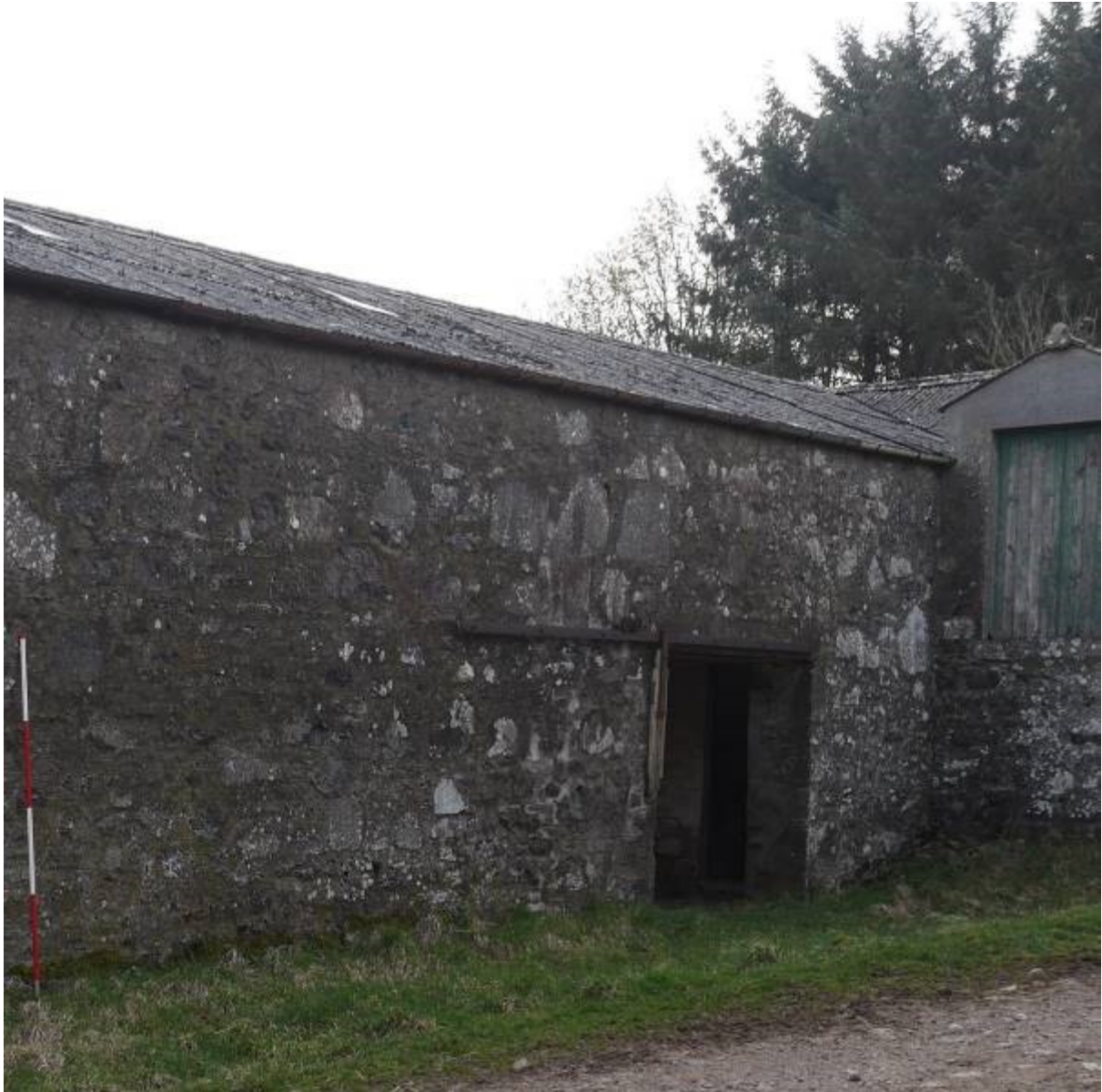
Illustration 32 – South Western elevation of Building 5
