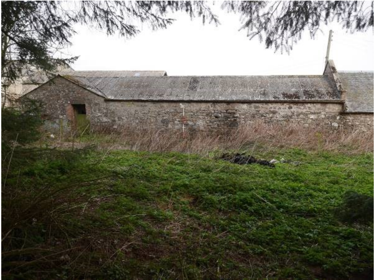
Illustration 15 – South Eastern elevation of Building 2
