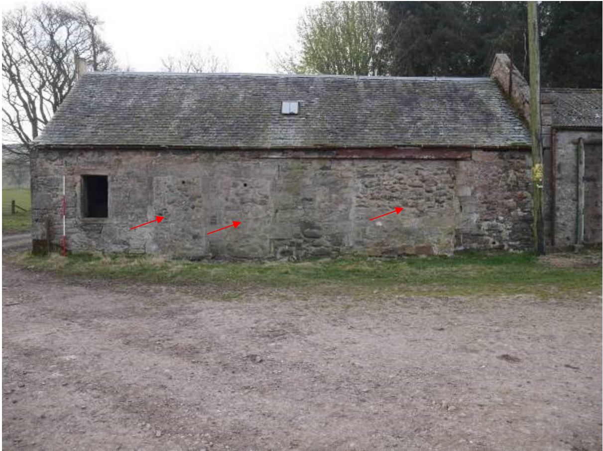
Illustration 6 – North Western elevation of Building 1 (blocked doorways marked with red arrows)
