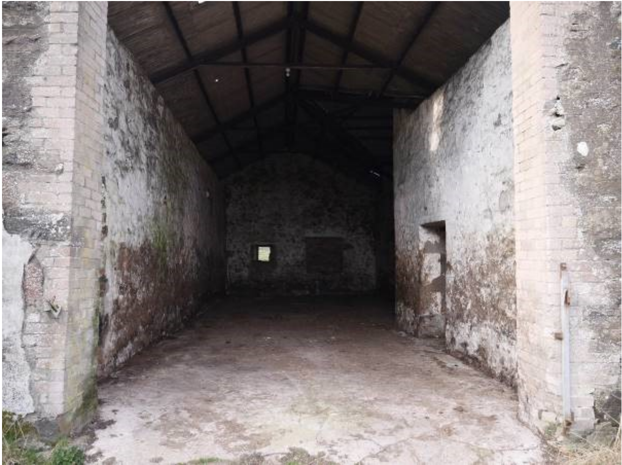
Illustration 28 – Internal view of Building 4 looking South West
