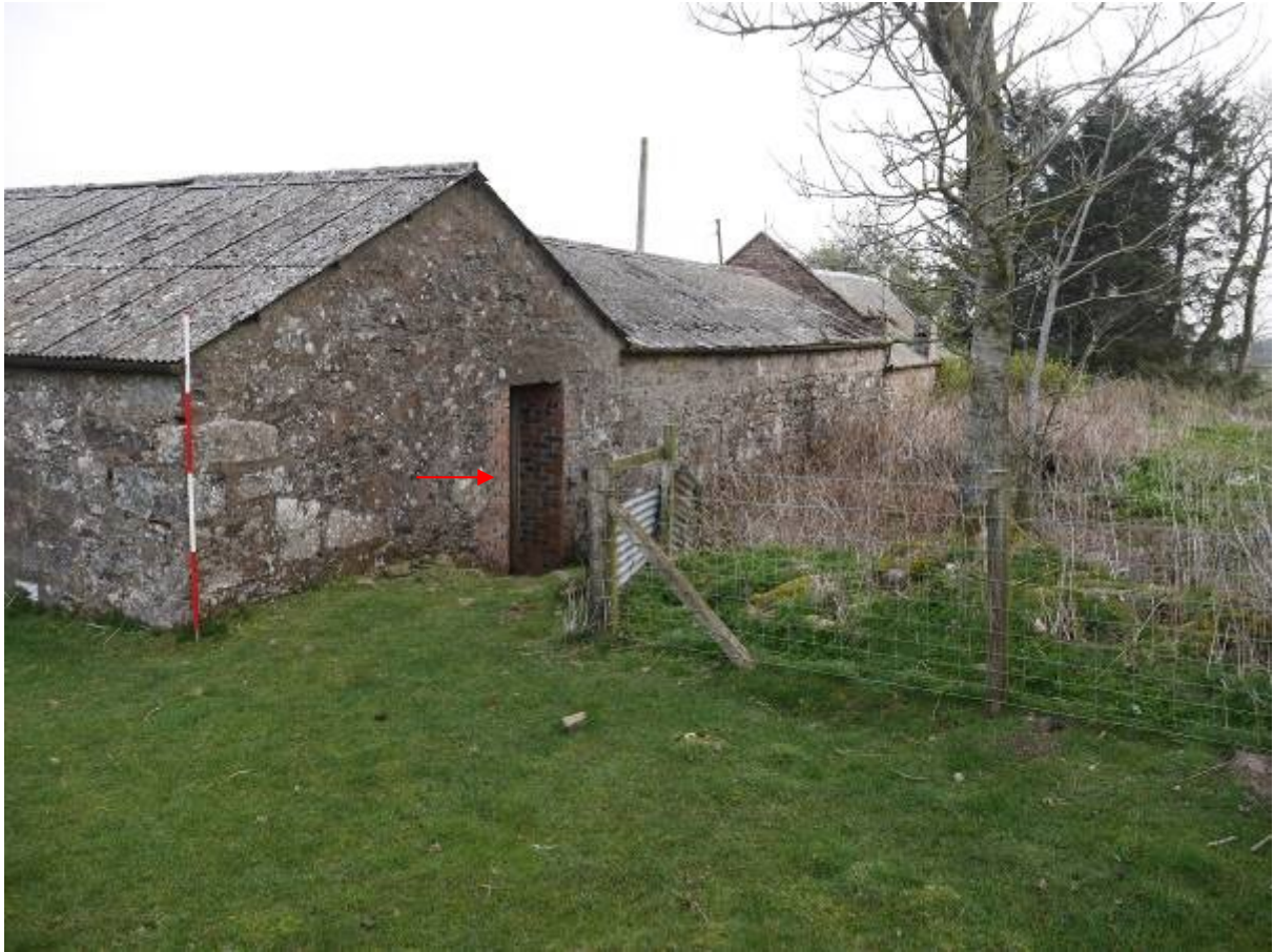
Illustration 20 - South Eastern elevation of Building 3 (doorway marked with red arrow)
