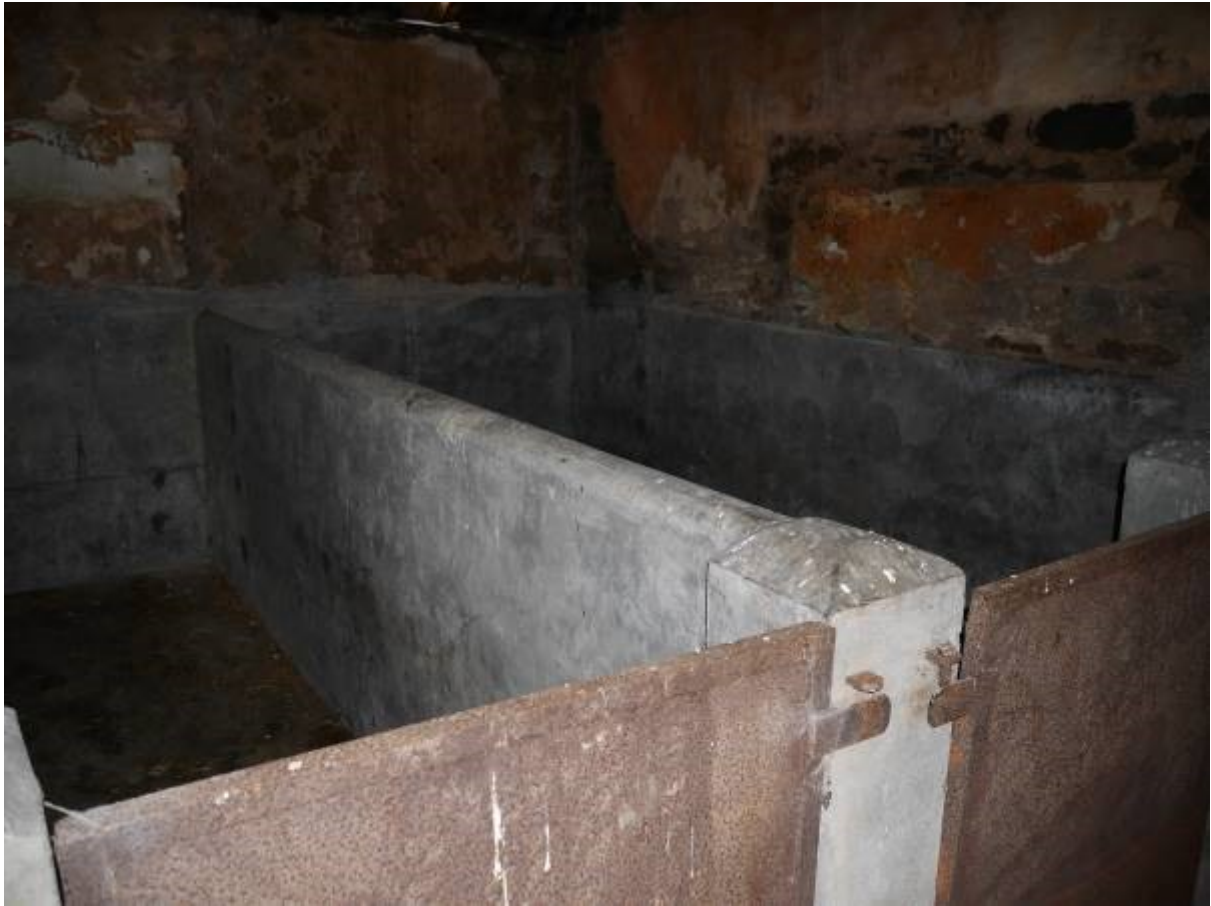
Illustration 11 - Animal pens with metal doors in Room a of Building 1 looking South
