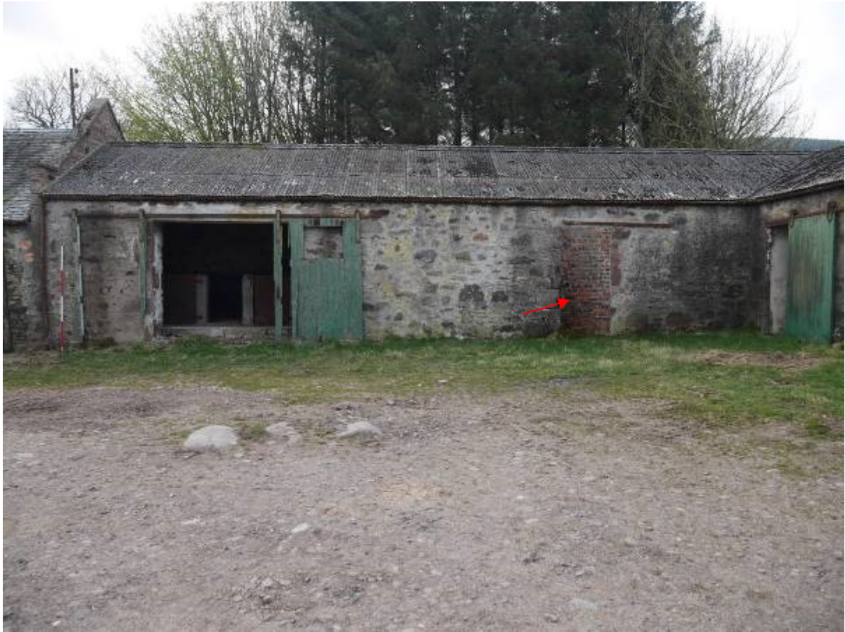
Illustration 14 – North Western elevation of Building 2, blocked doorway marked with red arrow
