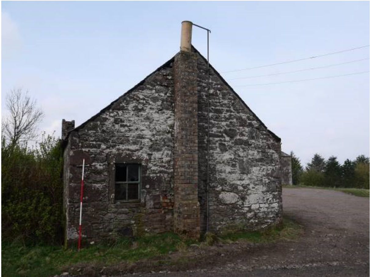
Illustration 9 – North Eastern gable elevation of Building 1
