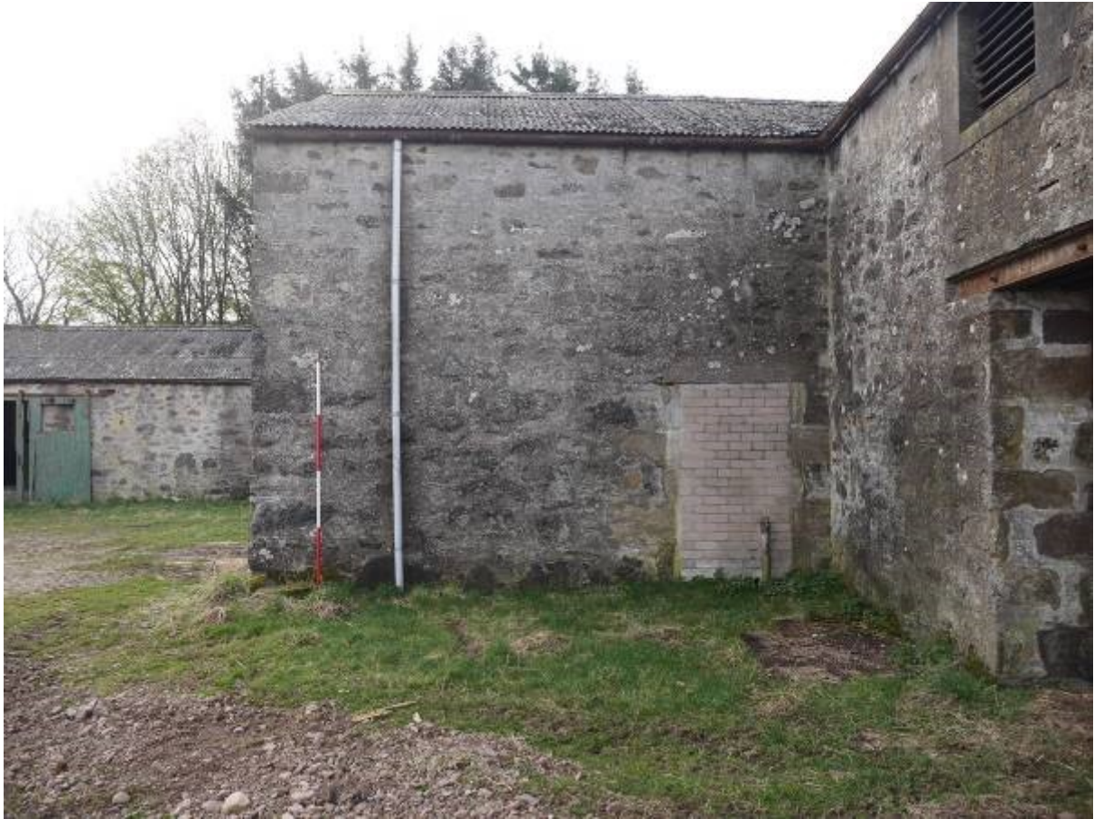
Illustration 23 – North Western elevation of Building 4 blocked doorway visible to right
