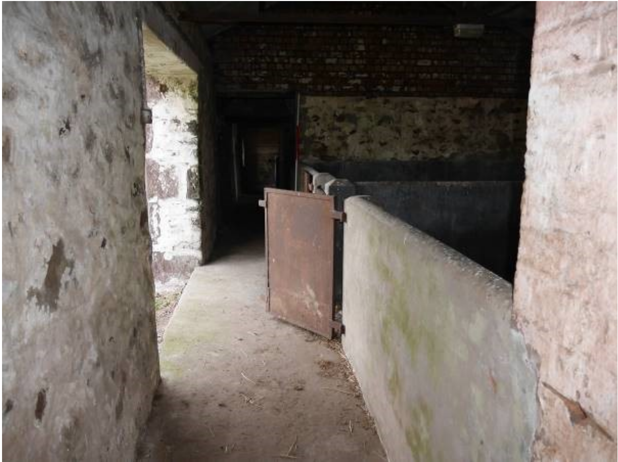
Illustration 16 – animal pens in room a of Building 2 looking North East
