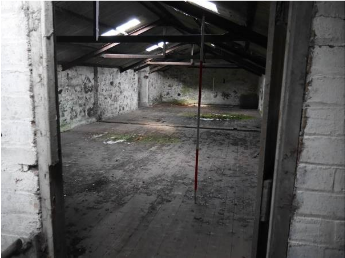
Illustration 34 – Upper floor of Buildings 5 and 6 looking North West
