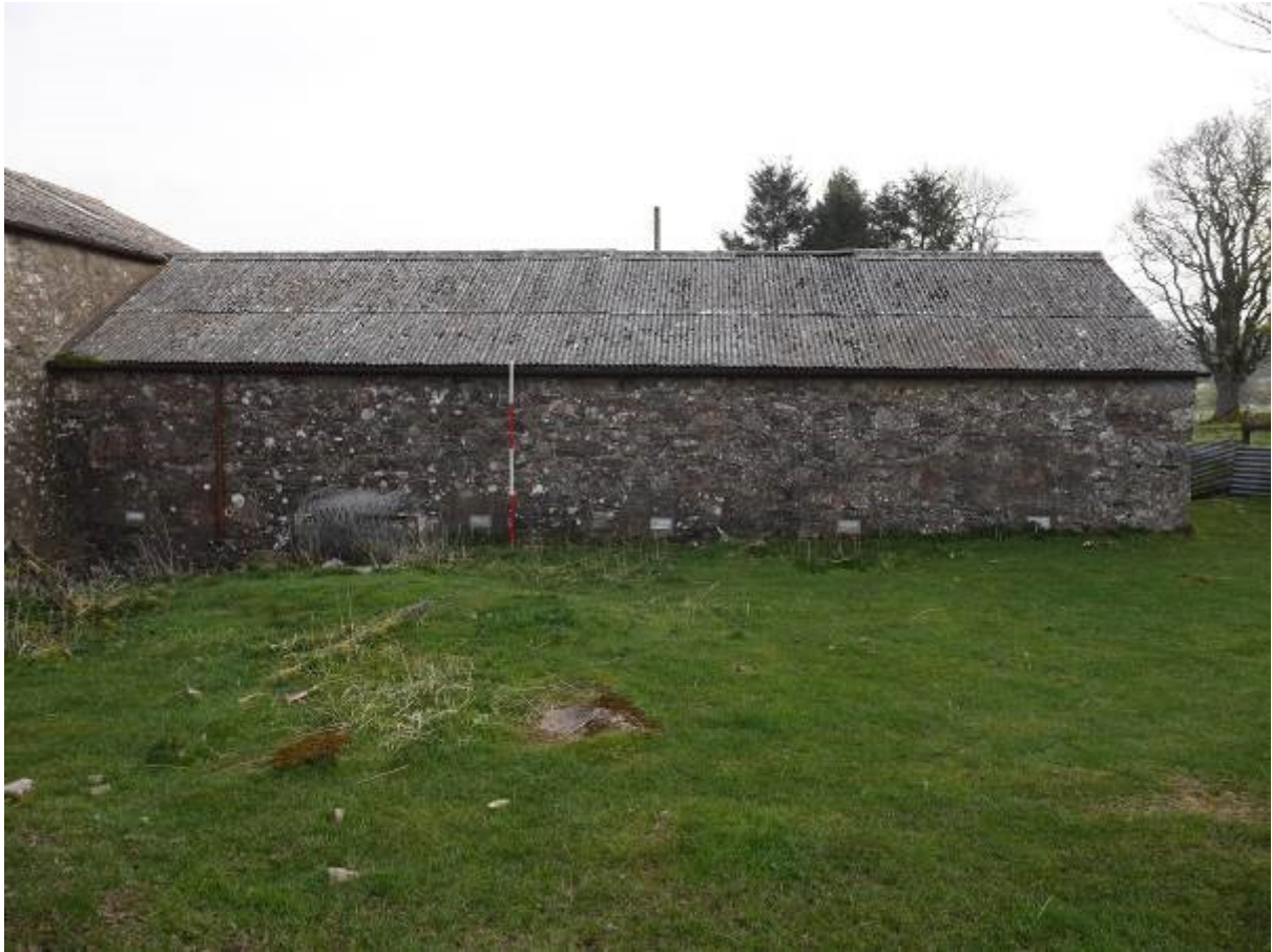
Illustration 19 – South Western elevation of Building 3
