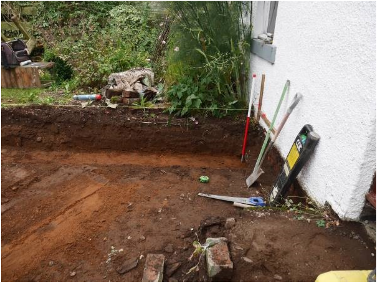
Illustration 7- Southern foundation trench totally excavated showing Context 200 lying on natural sand 201.
