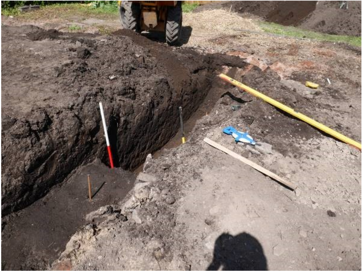
Illustration 9 Trench D looking North showing stepped new foundation cut into soil 103
