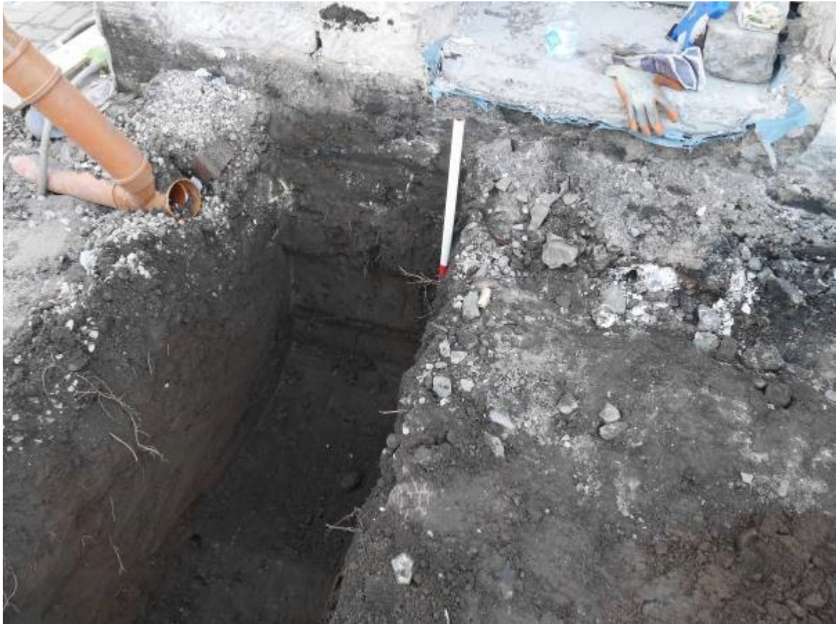
Illustration 11 Trench F looking South West showing deep soil build up 103 adjacent to standing building at 67 Blackness Road
