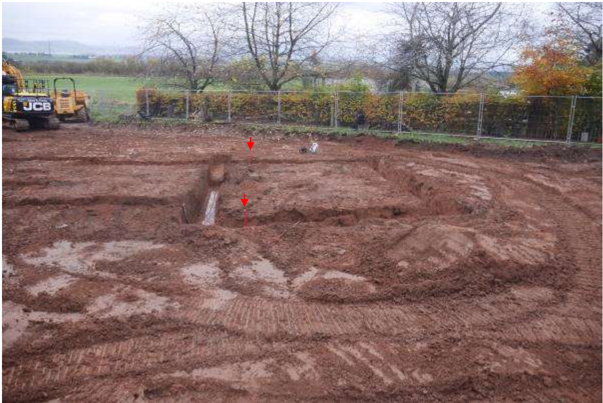
Illustration 12 - Detail view across excavated foundation trenches for new house looking South West. Line of cut feature 102 is marked by ranging rods (red arrows).
