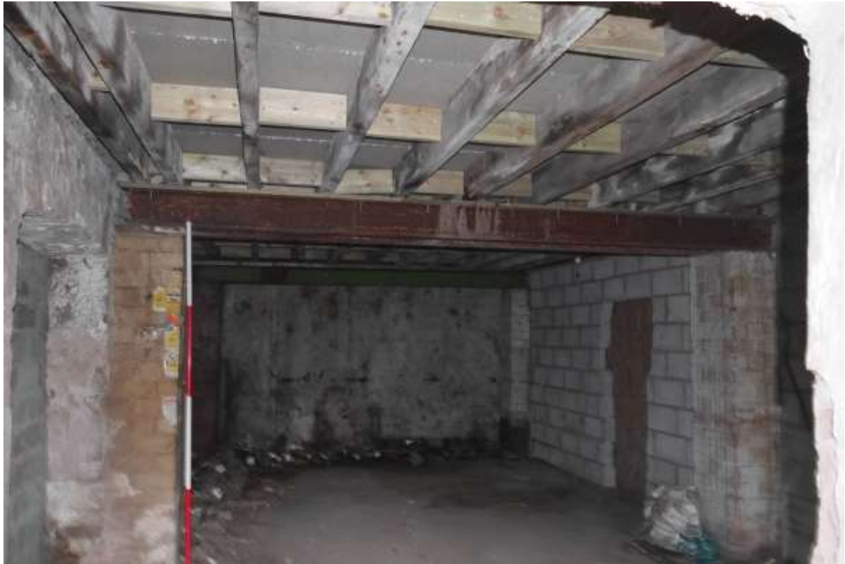
Illustration 20- Basement floor at Northern end of mill building looking East.
