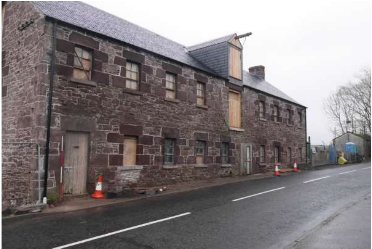
Illustration 16- General view of North Eastern elevation fronting onto road.
