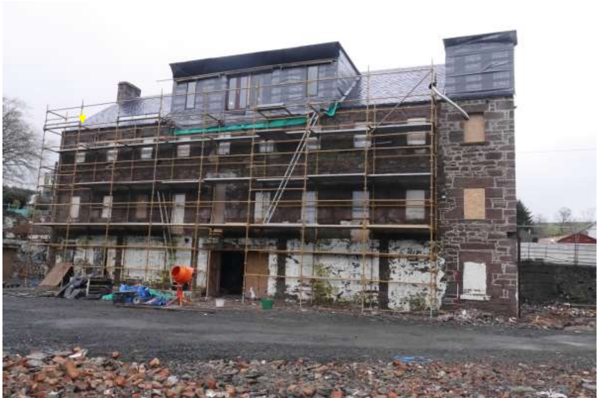
Illustration 13- South Western elevation of Mill building showing new roof and dormers.
