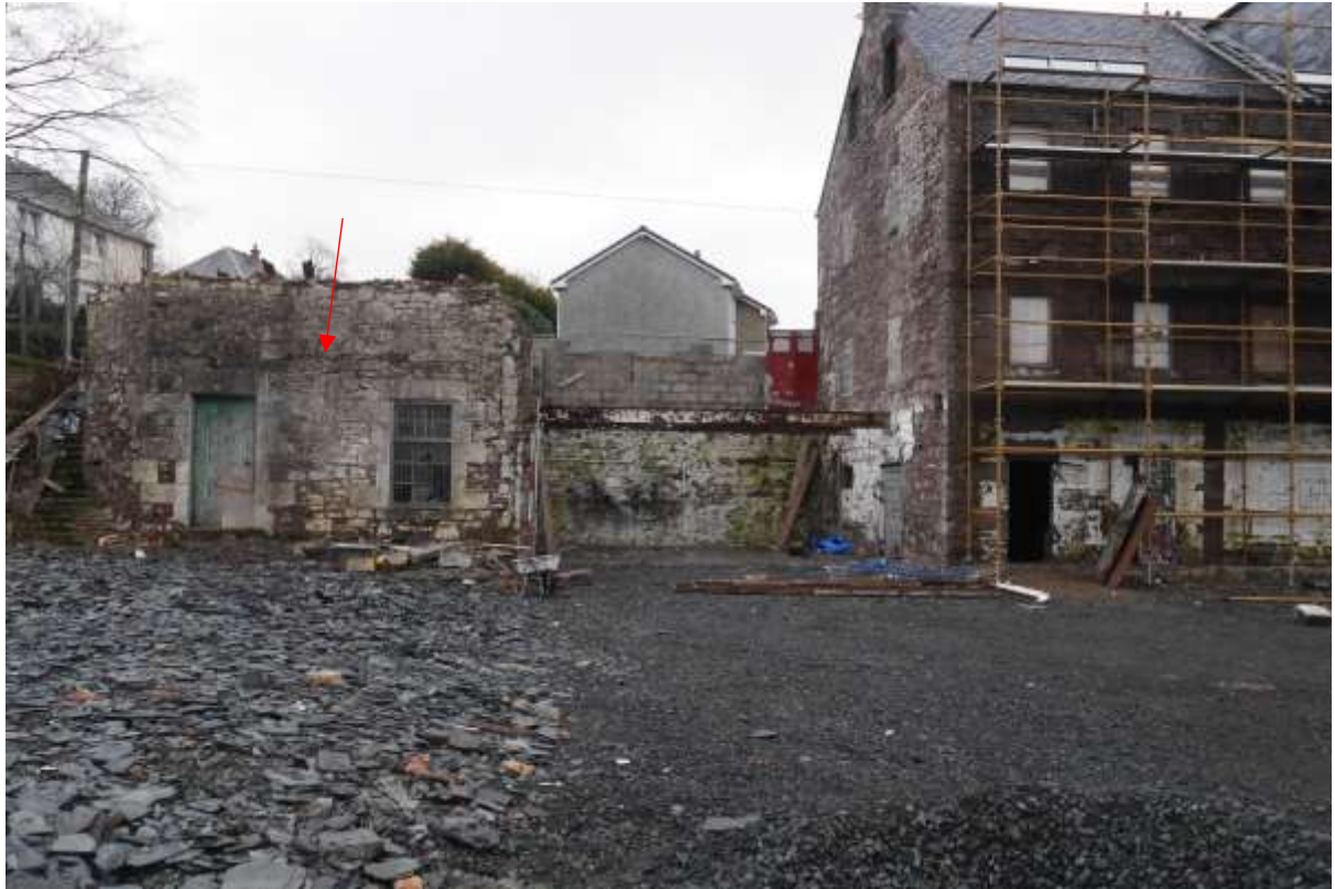
Illustration 22- Small building on North West side of mill building (red arrow).
