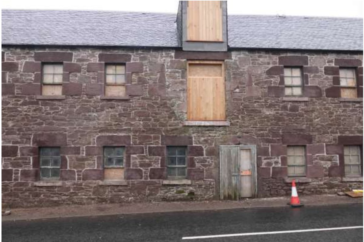
Illustration 18- Centre of North Eastern elevation.
