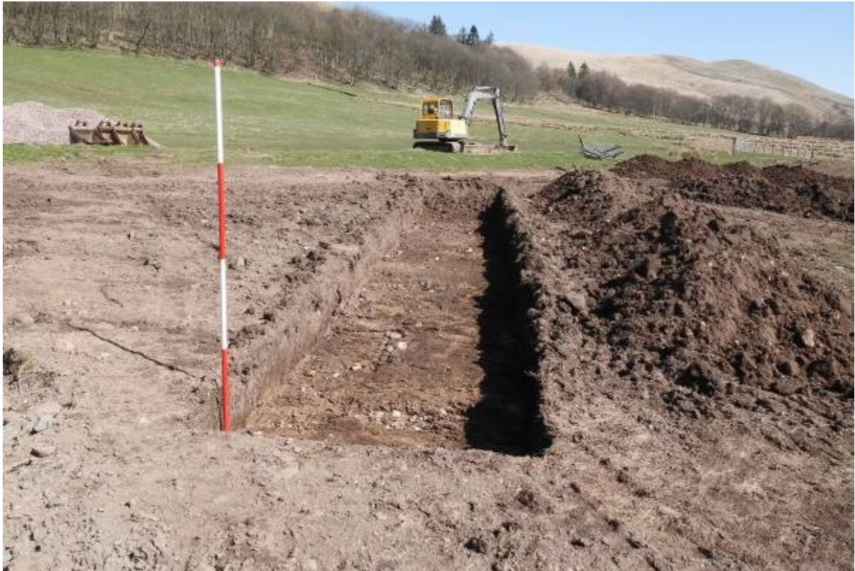
Illustration 13- Evaluation trench A excavated to top of natural 101 looking NE.
