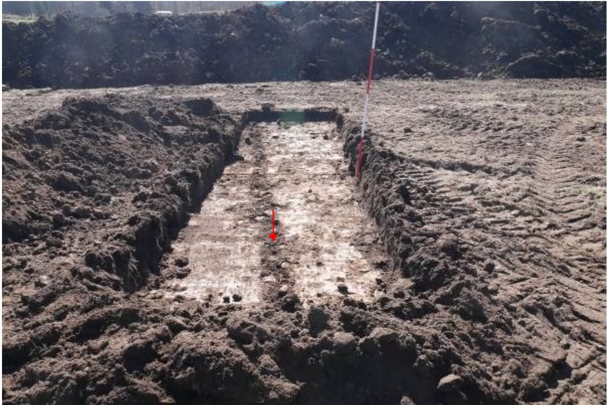
Illustration 15- Evaluation trench B excavated to top of natural 201 looking S, line of field drain 203 visible at red arrow.
