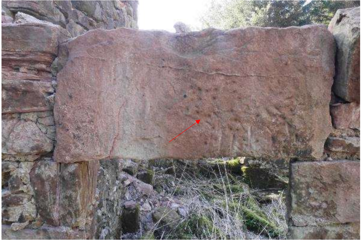
Illustration 27- Red sandstone lintel of window in Room A in Northern elevation of building red arrow shows visible pecked tool marks (no 7).
