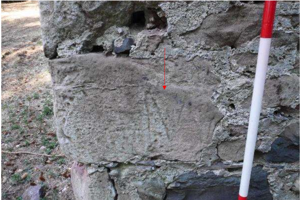
Illustration 20- Detail of lower reused piece of yellow sandstone (no 3) with incised letter 'M' in Eastern gable of building.
