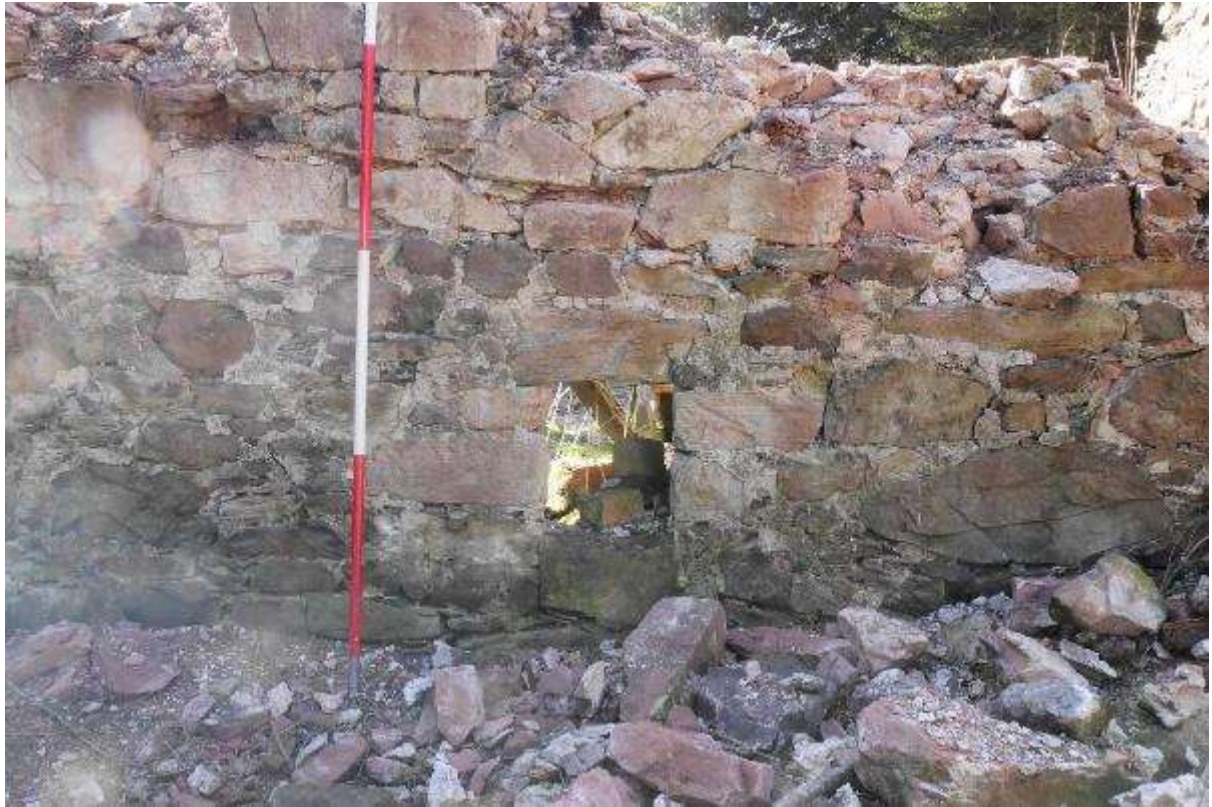
Illustration 28- Small window in Room A in Northern elevation of building.
