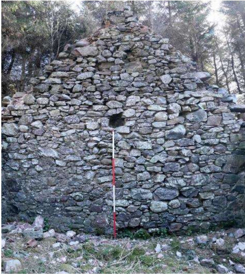
Illustration 42- Internal Western elevation of Room B.
