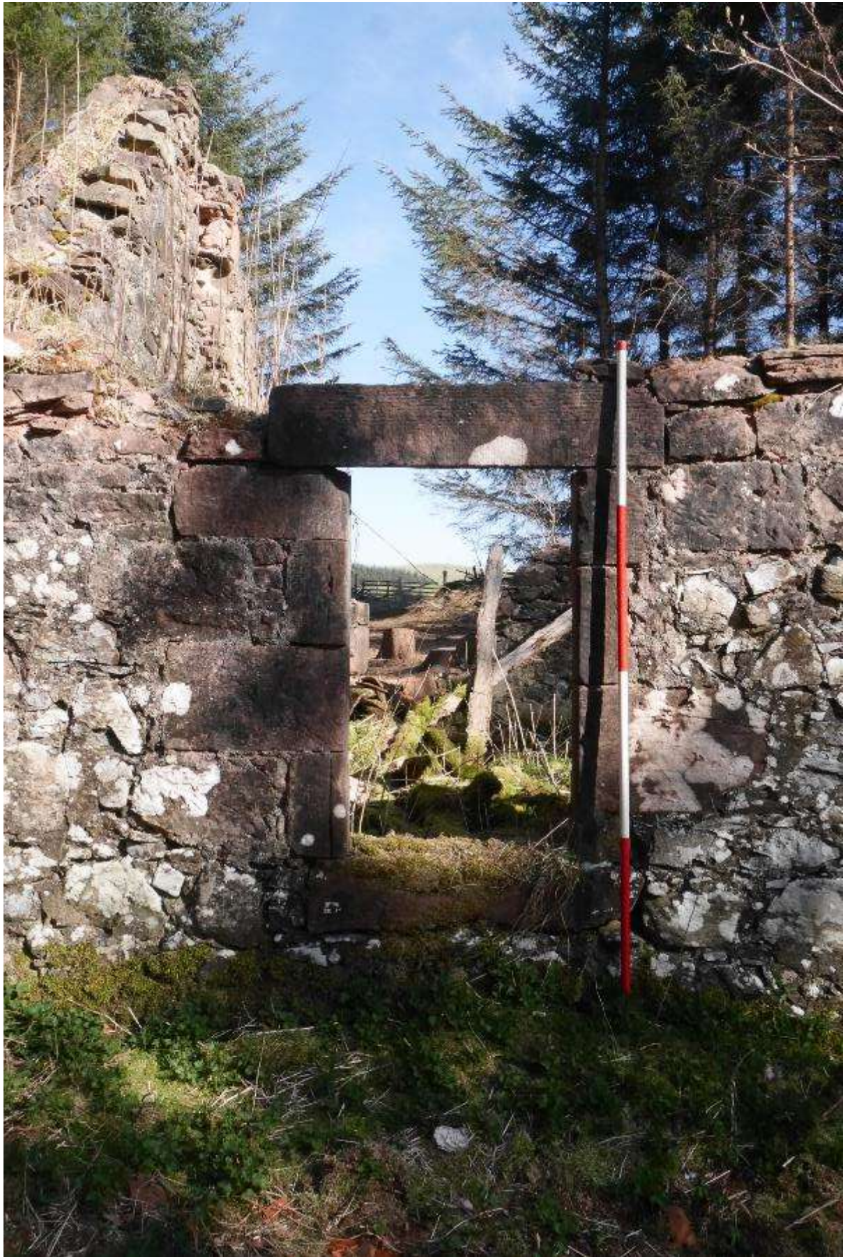
Illustration 13- Window in Room A at Western end of Southern elevation.
