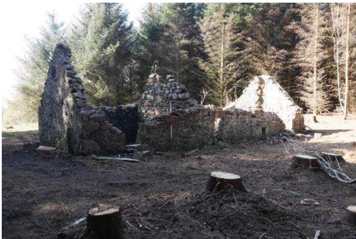
Illustration 21- Northern elevation of building looking South West.
