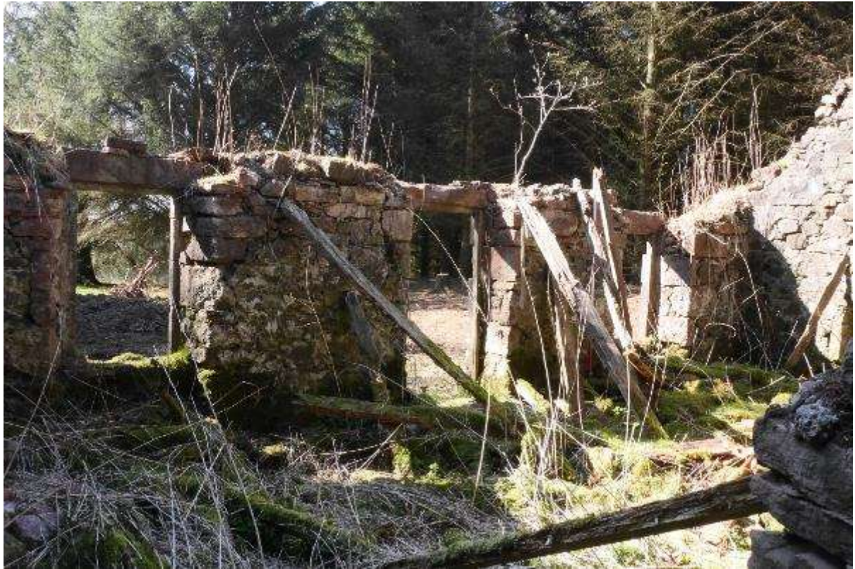
Illustration 38- Southern internal elevation of Room A.
