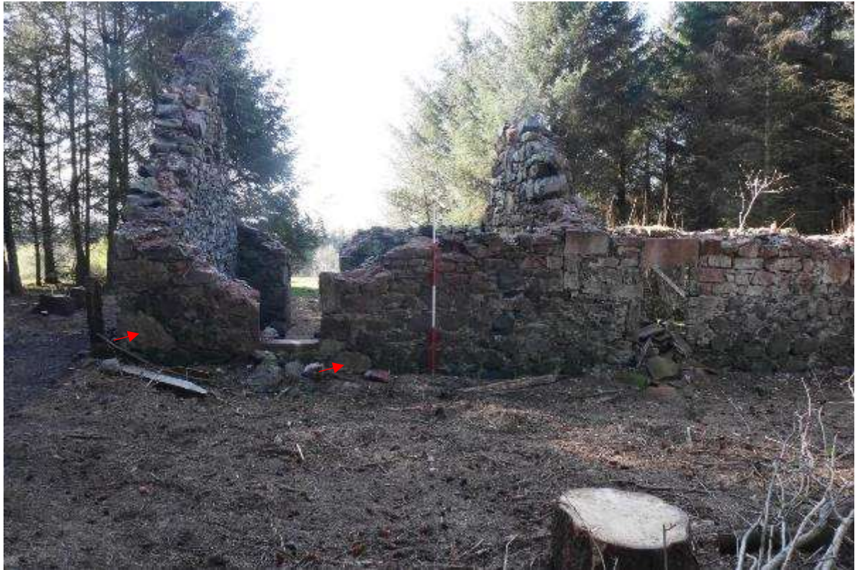
Illustration 22- Window in Room B at Eastern end of Northern elevation of building, red arrows show location of reused stones with visible toolmarks (numbers 4 and 5).
