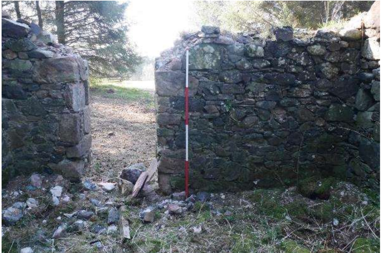
Illustration 43- Internal Northern elevation of Room B.
