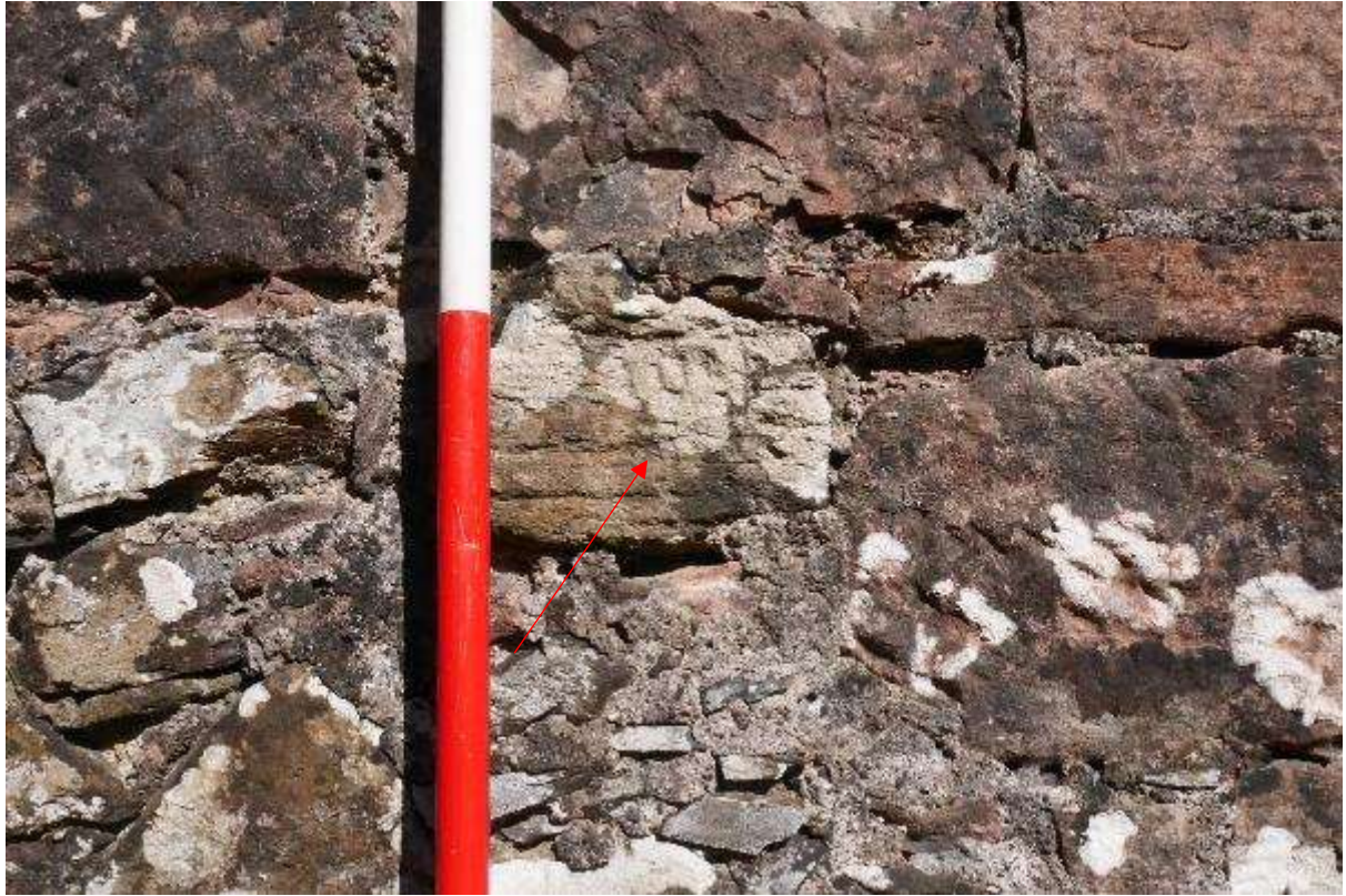
Illustration 15- Piece of yellow sandstone with toolmarks (no 1) in Southern elevation of Room A.
