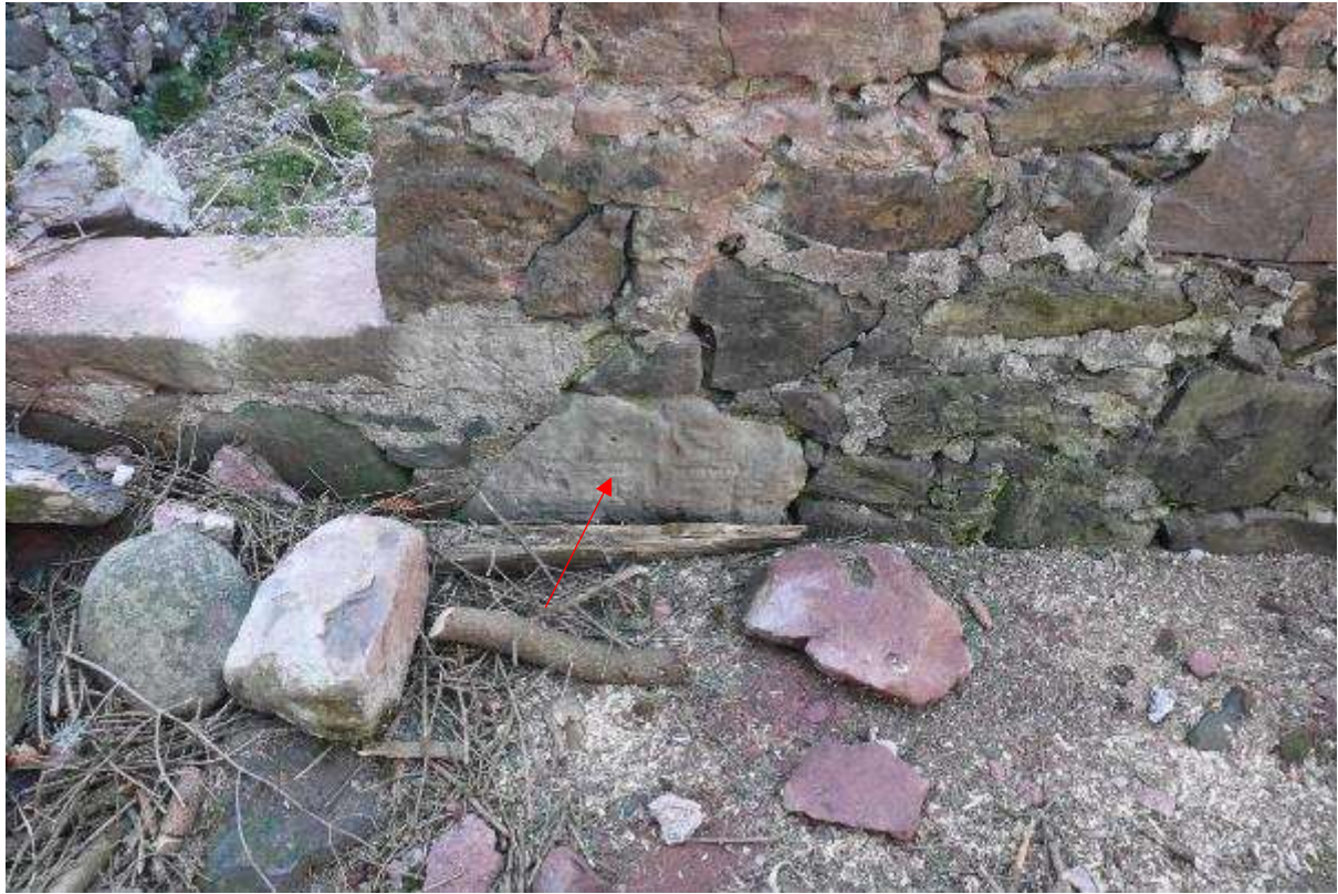
Illustration 24- Detail of reused piece of yellow sandstone (no 5) on Western side of window in Room B in Northern elevation with visible tool marks.
