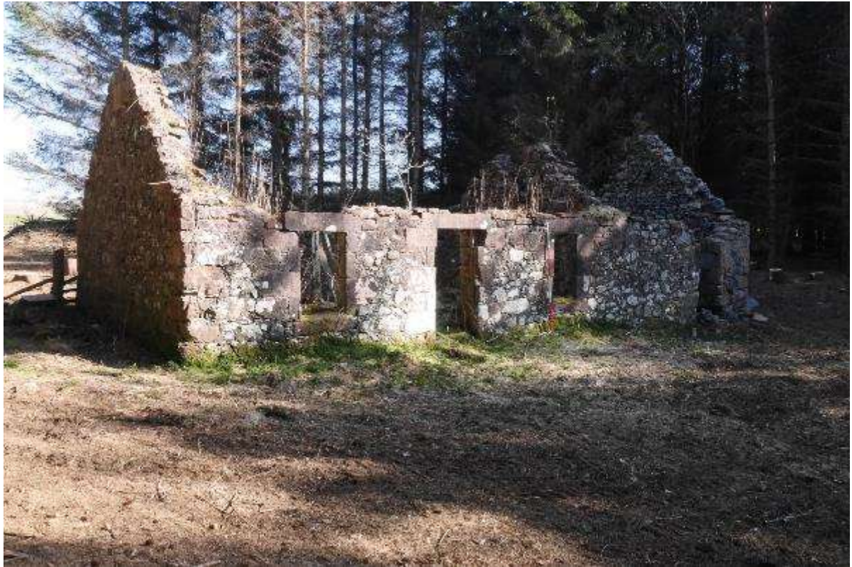
Illustration 12- Southern elevation of building looking North East.
