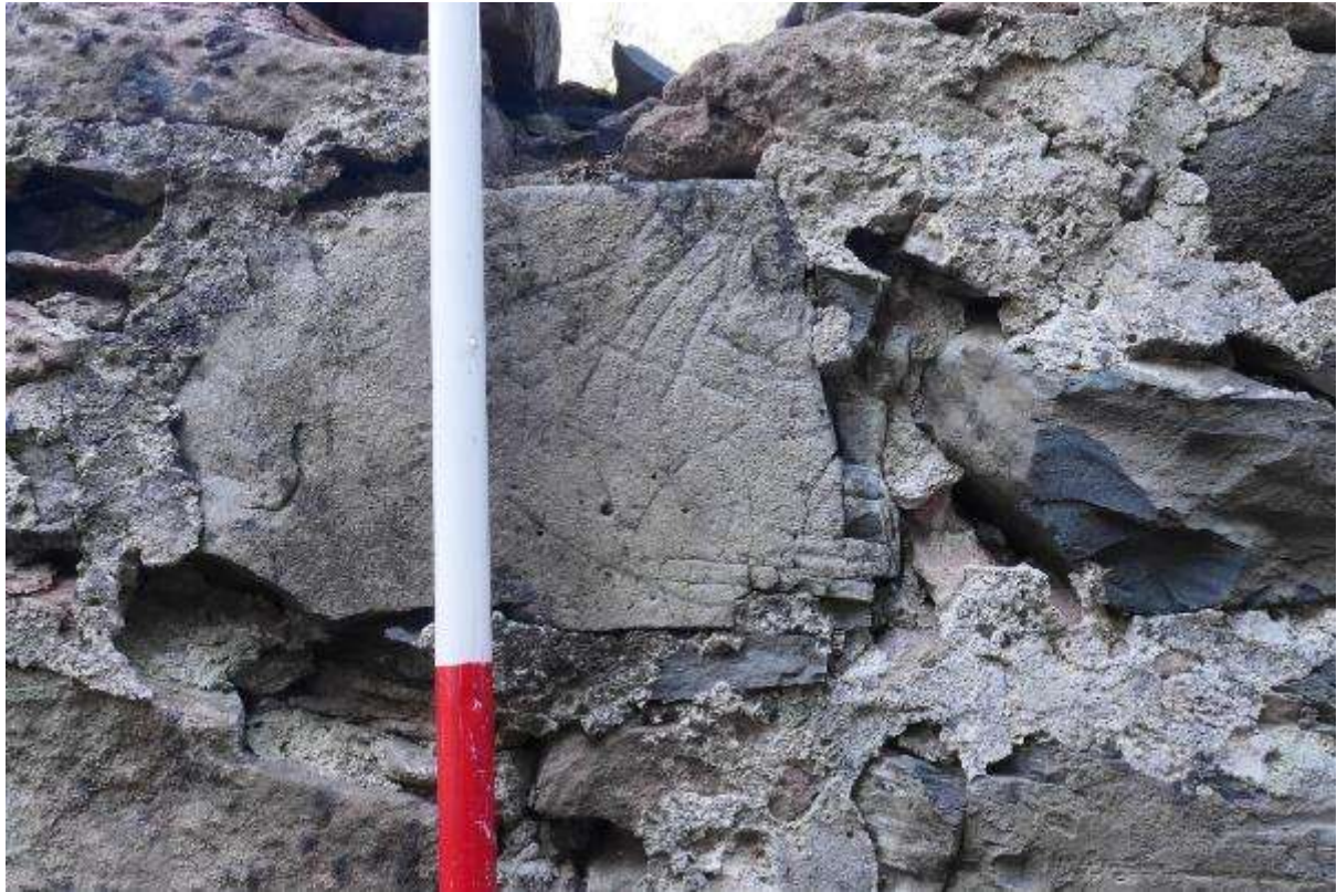
Illustration 19- Detail of upper reused piece of yellow sandstone (no 2) in Eastern elevation of building with incised lines.
