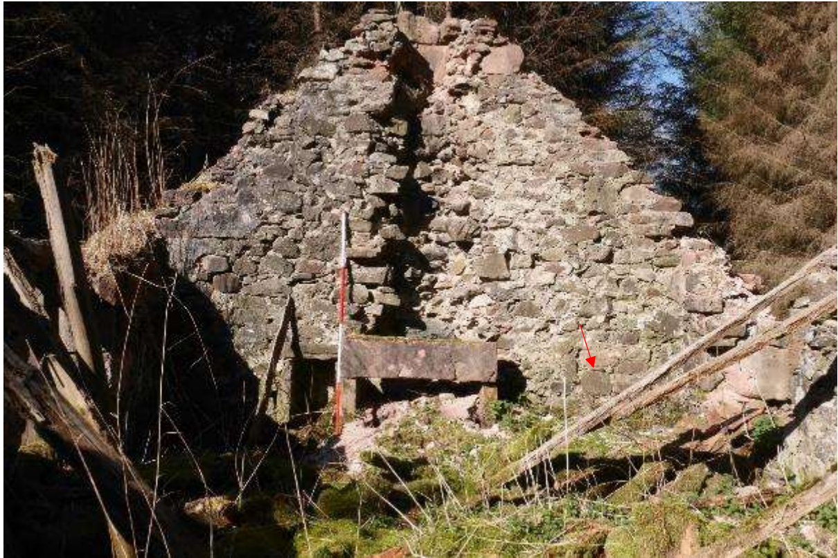
Illustration 33- Central fireplace in Eastern elevation of Room A with small cupboard visible to left and blocked cupboard at red arrow, chimney scar visible in wall face.
