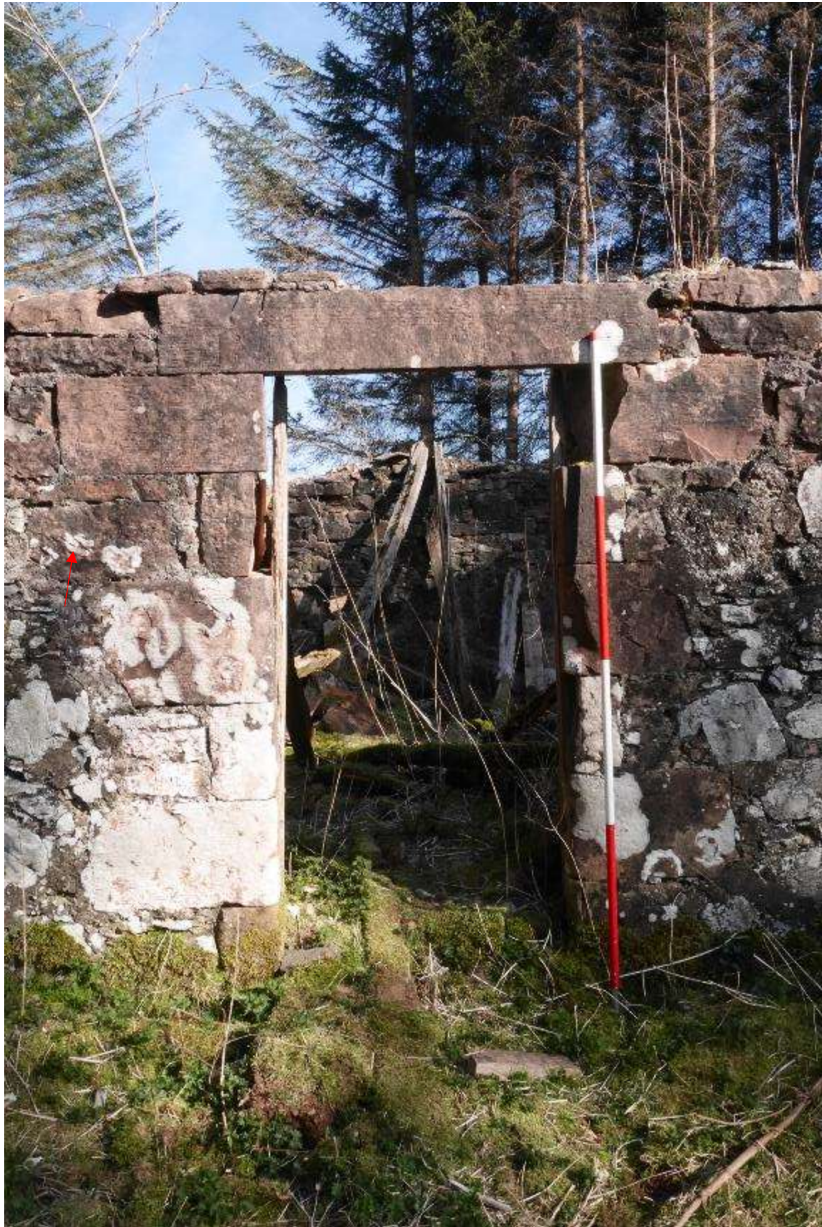
Illustration 14- Doorway Room A in Southern elevation of building, red arrow indicates stone with toolmarks (no 1).
