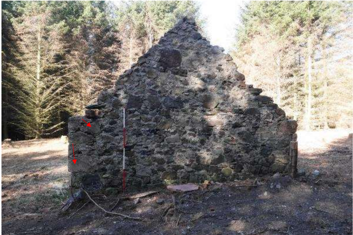
Illustration 18- Eastern elevation of building, red arrow shows location of reused stones with incised lines (no 2 upper) and incised letter 'M' (no 3 lower).
