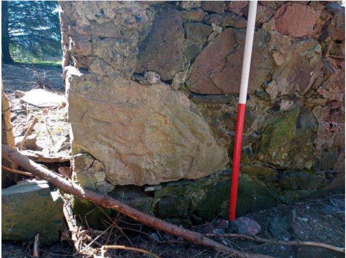
Illustration 23 – Reused piece of yellow sandstone with toolmarks (no 4) at NE corner of N elevation.
