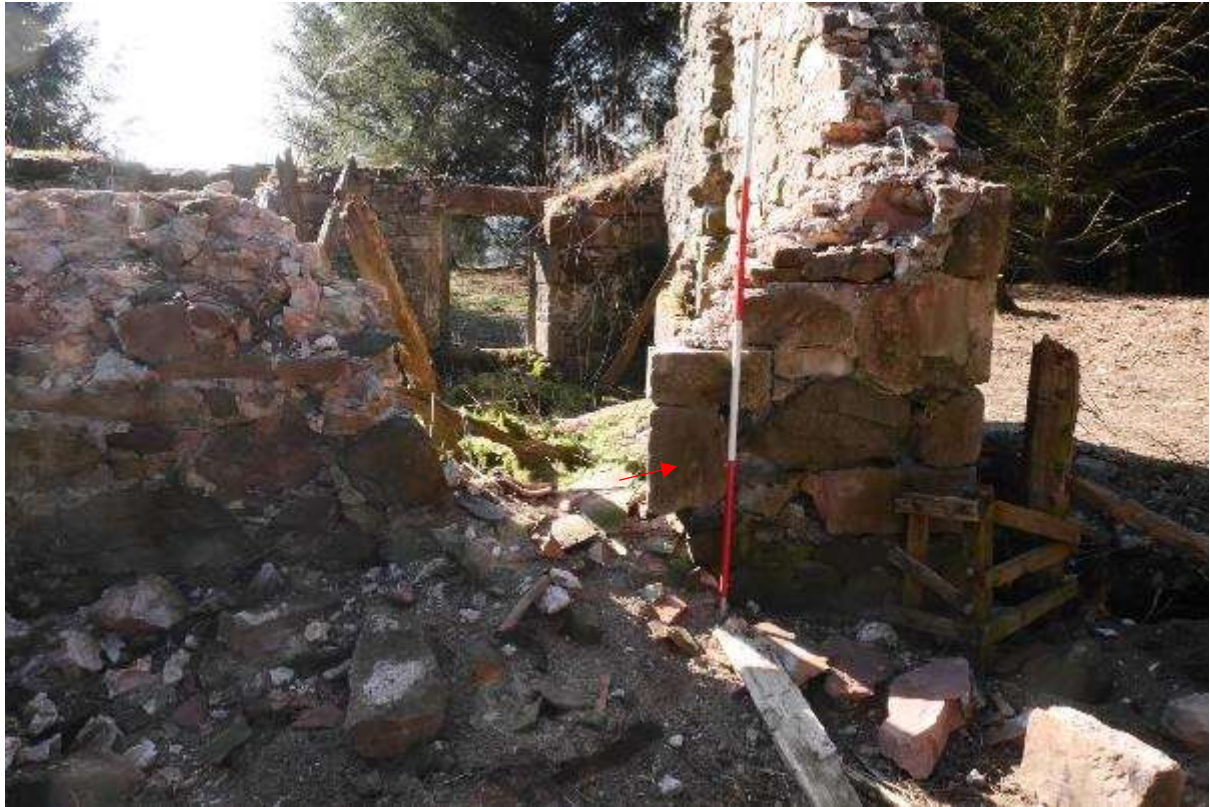
Illustration 29- Window in Room A in Northern elevation of the building, red arrow indicates reused architectural fragment (no 8).
