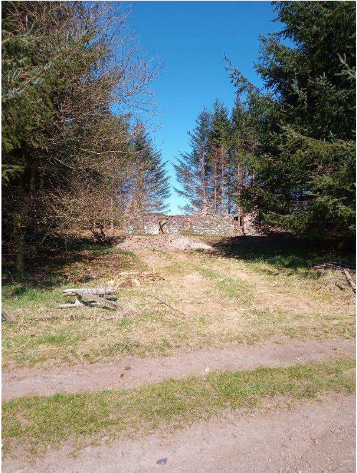
Illustration 11- General view of ruinous building at 'Windy Walls' in tree plantation looking North.
