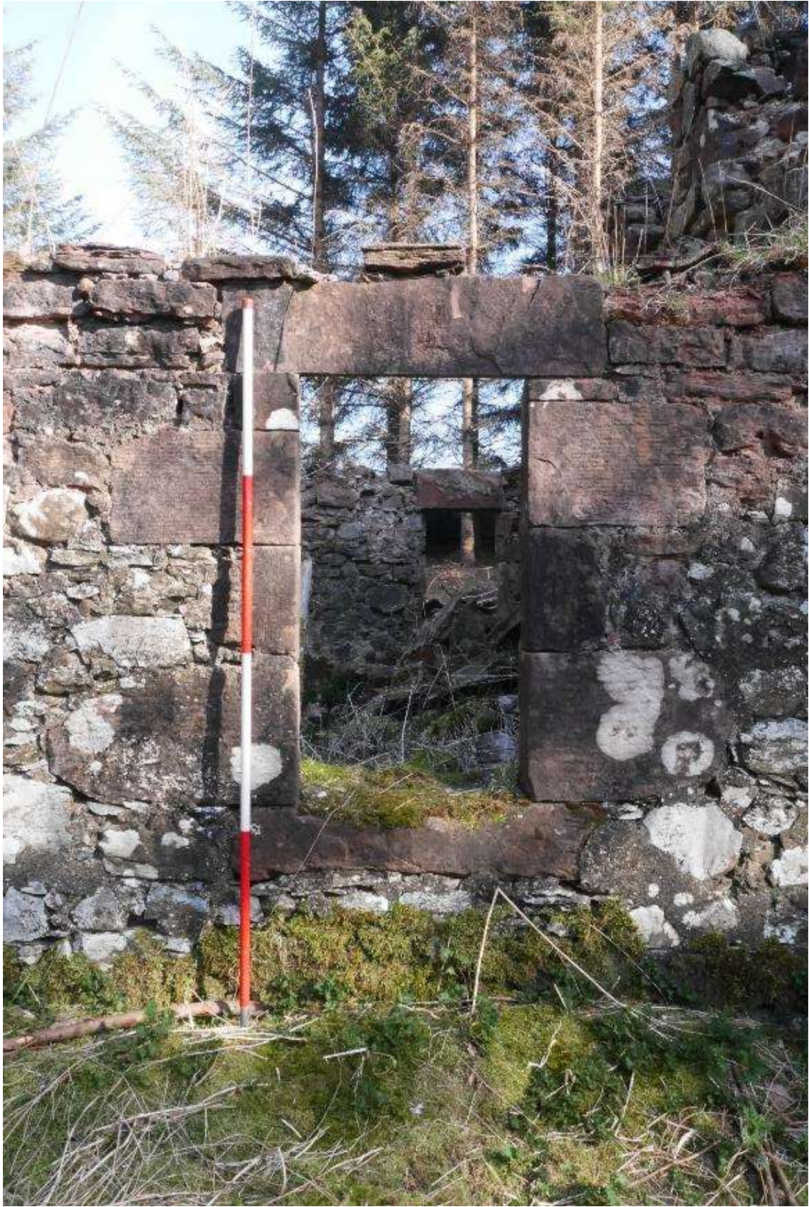
Illustration 16- Window in Room A in Southern elevation of building.
