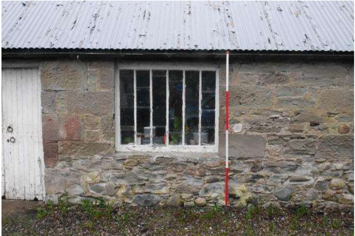
Illustration 7- Window in Eastern elevation of Building 1.
