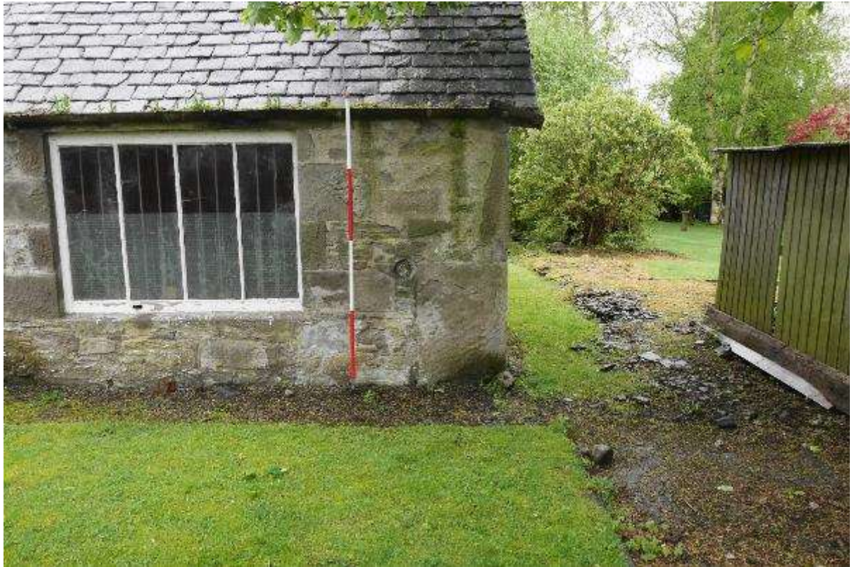
Illustration 19- Western end of North facing elevation of Building 2 looking South.
