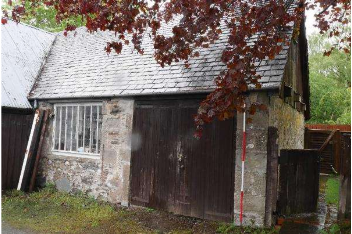
Illustration 15- South facing external elevation of Building 2 looking North.
