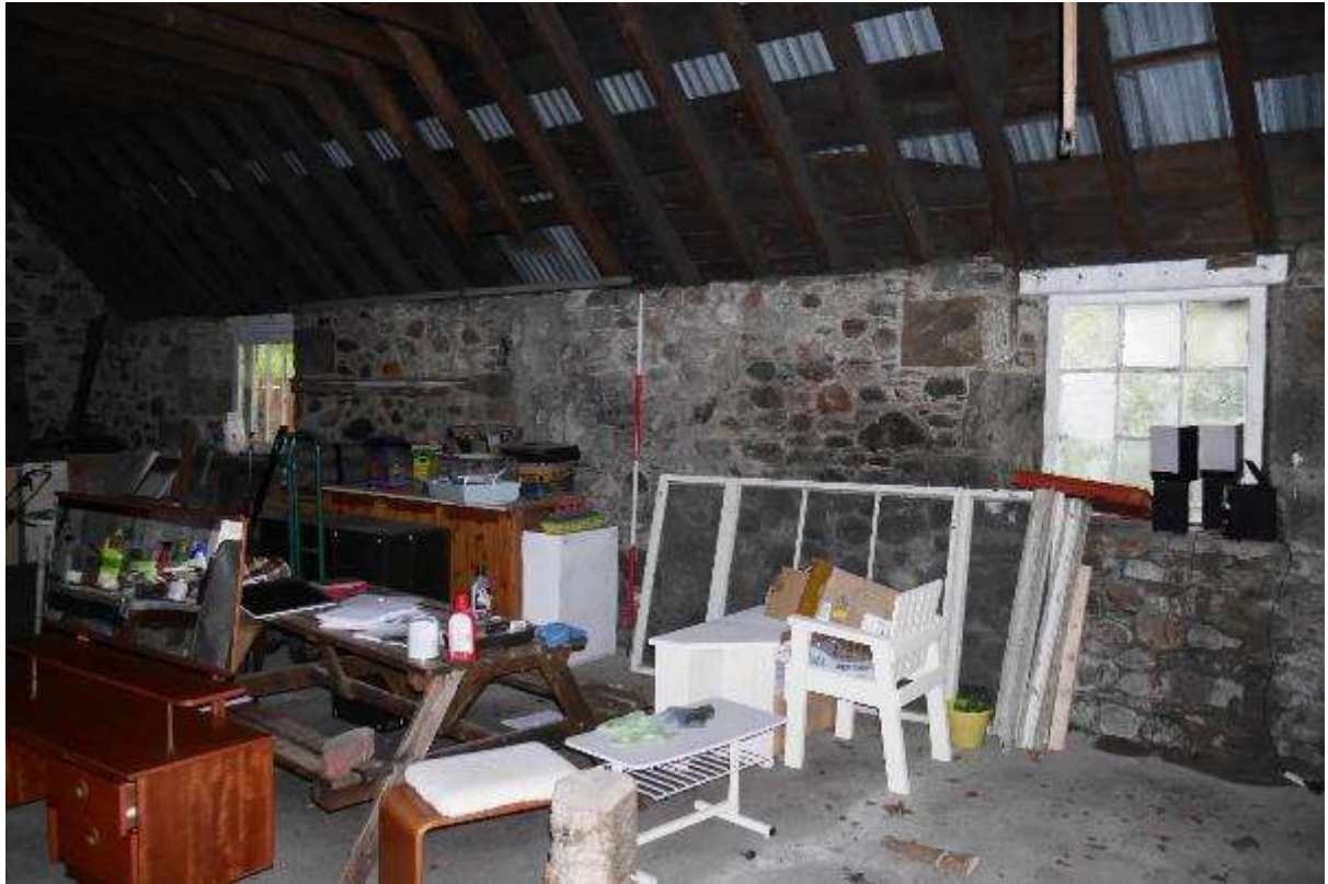
Illustration 12- Internal East facing elevation of Building 1.
