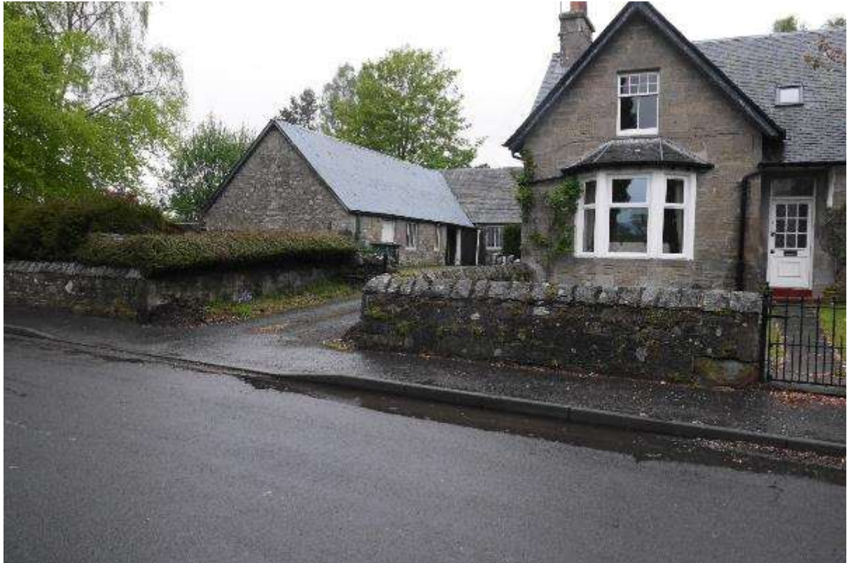
General view of Buildings surveyed adjacent to Dunsinane Cottage, Station Road, Murthly looking North West.
