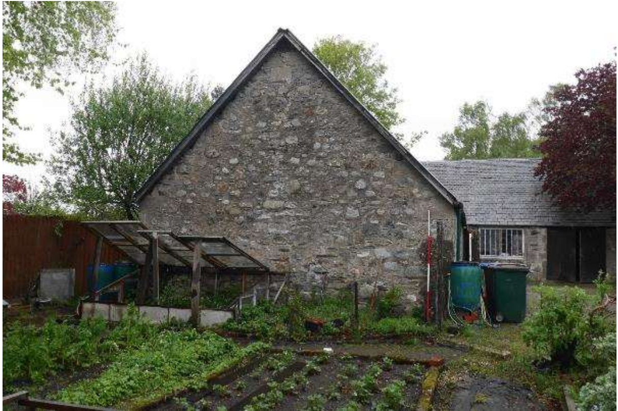
Illustration 9- Southern gable elevation of Building 1 looking North.
