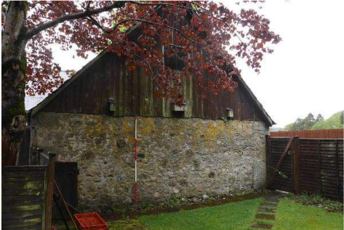
Illustration 16- East facing external elevation of Building 2 looking North West.
