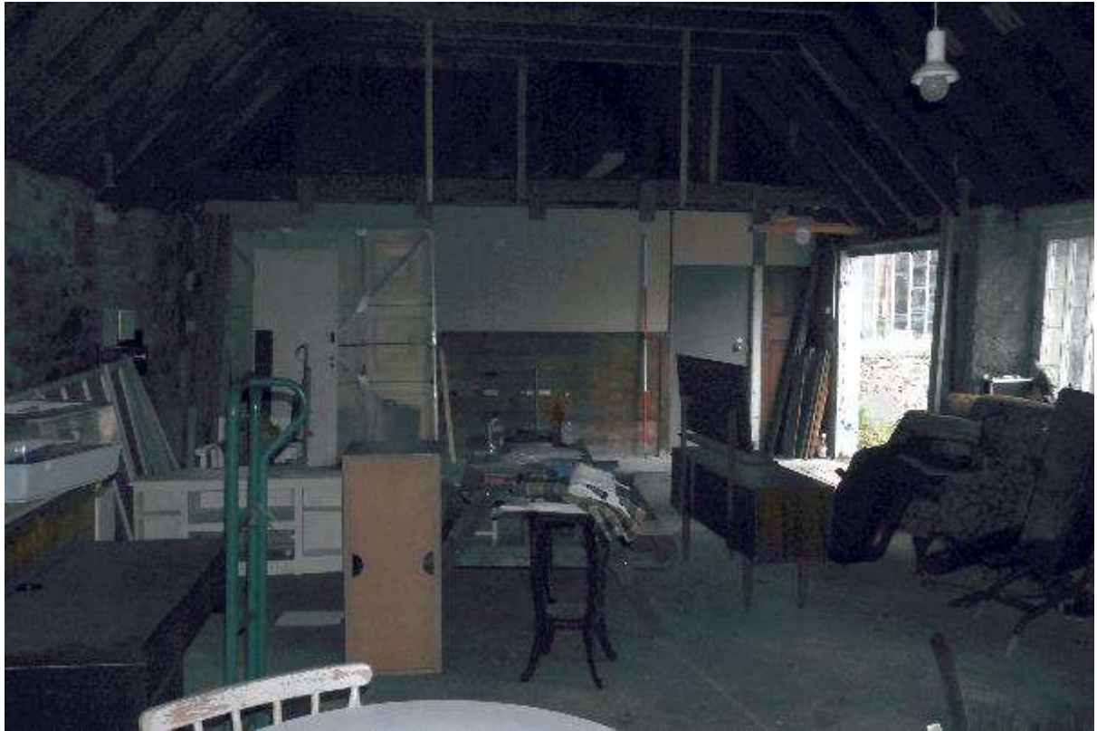
Illustration 13- Internal South facing wooden partition wall in Building 1.
