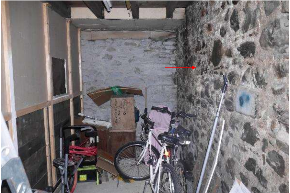
Illustration 14- South facing internal elevation of Building 1 (red arrow).
