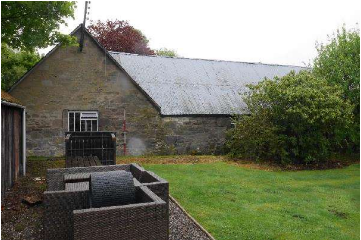
Illustration 20- External West facing elevation of Building 2, junction with Building 1 also visible.
