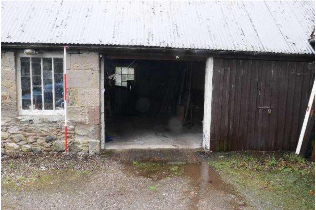
Illustration 8- Window and doorways at Northern end of Eastern elevation of Building 1.
