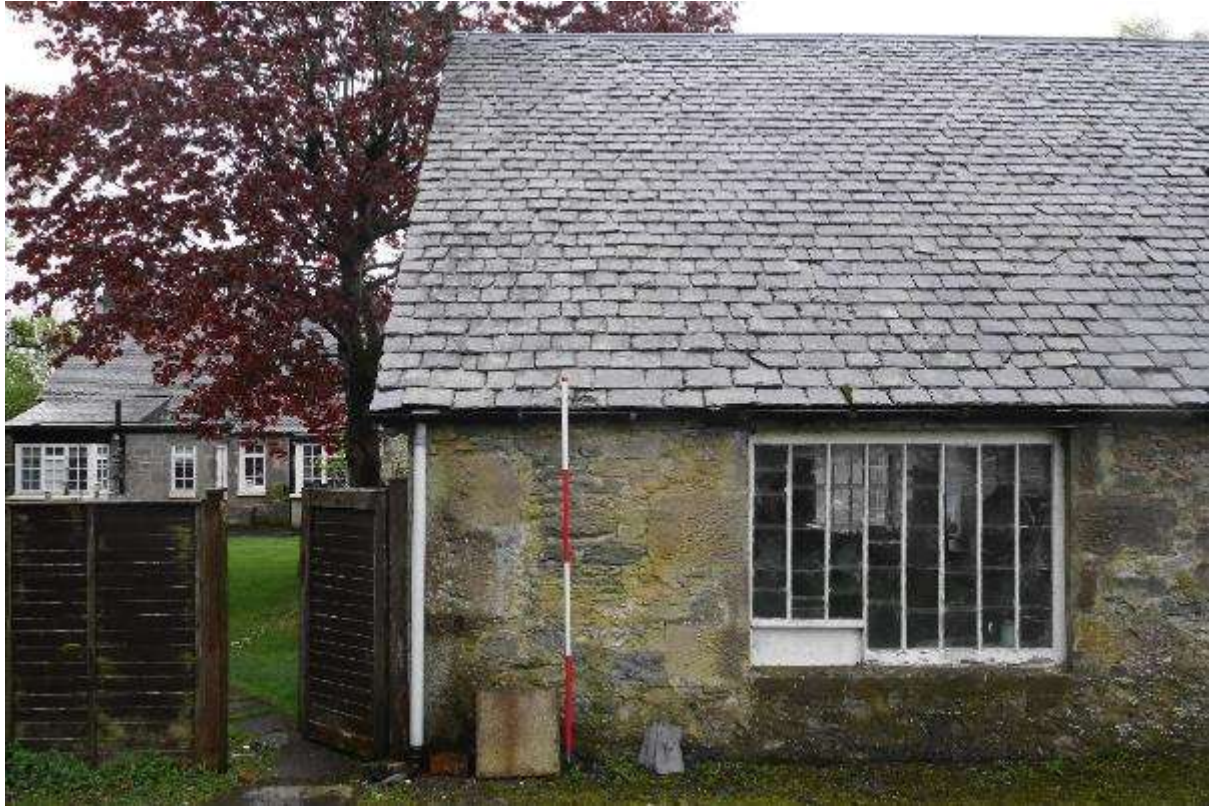
Illustration 18- Eastern end of Northern elevation of Building 2 looking South.
