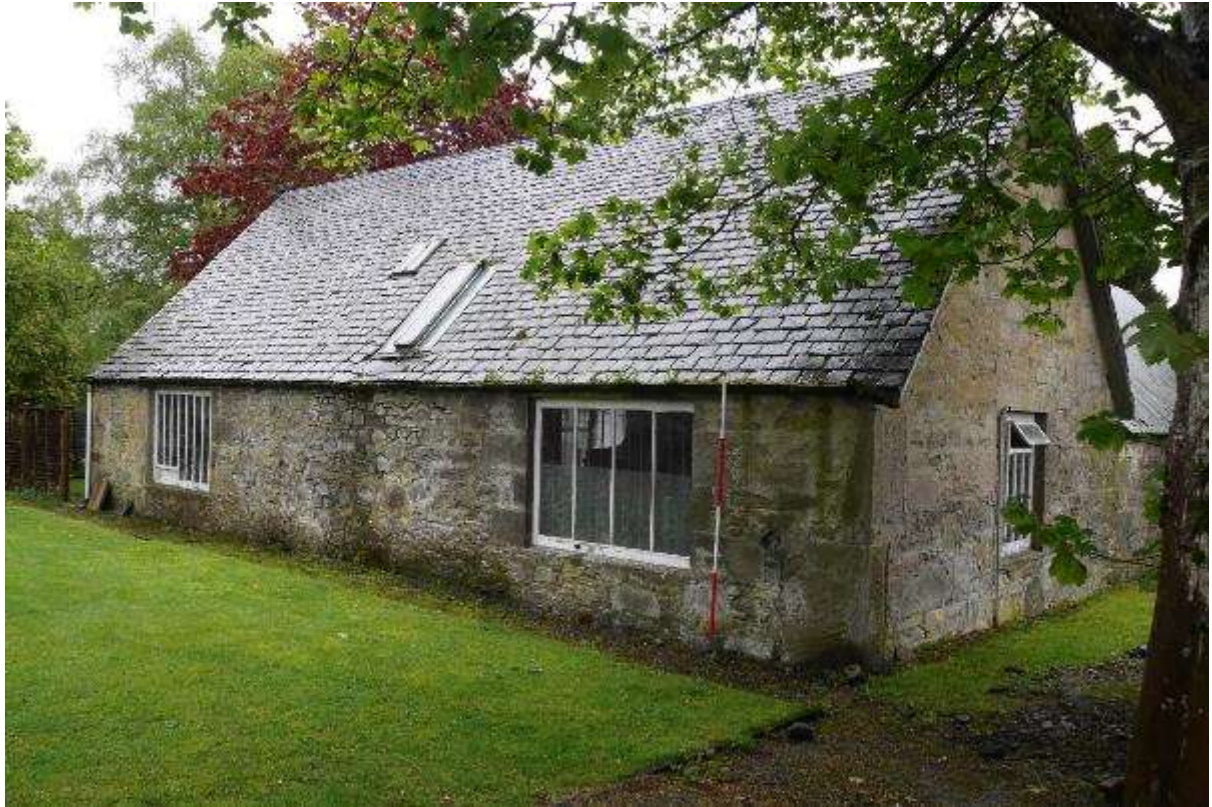
Illustration 17- North facing external elevation of Building 2 looking South East.
