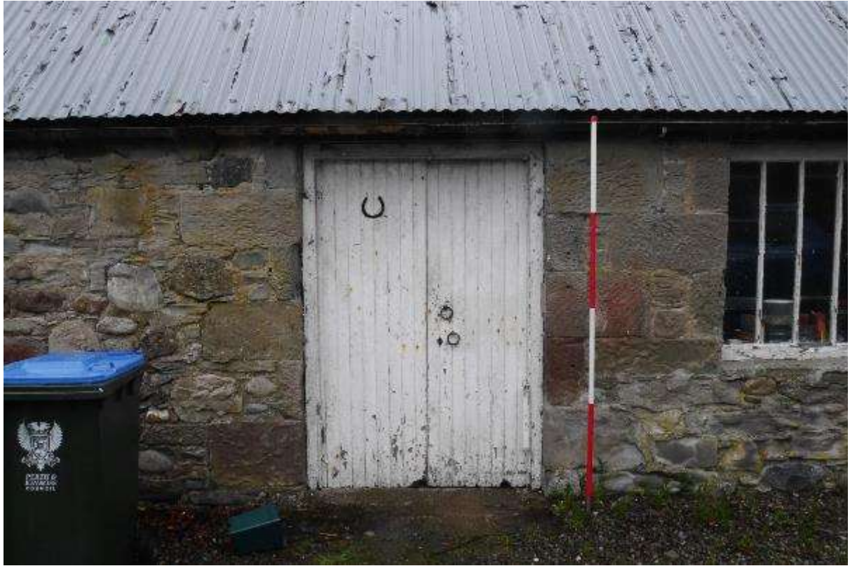
Illustration 6- Doorway at Southern end of Eastern elevation of Building 1.
