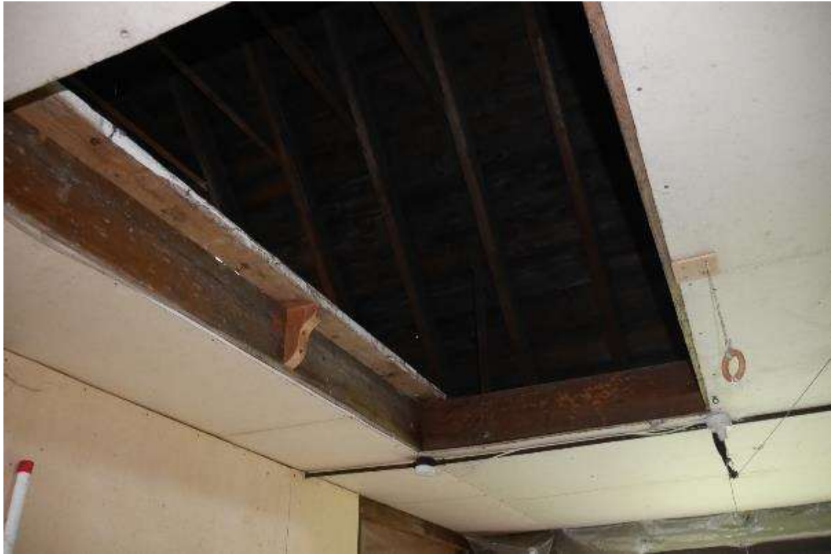
Illustration 26- Access to attic roof space in Building 2.
