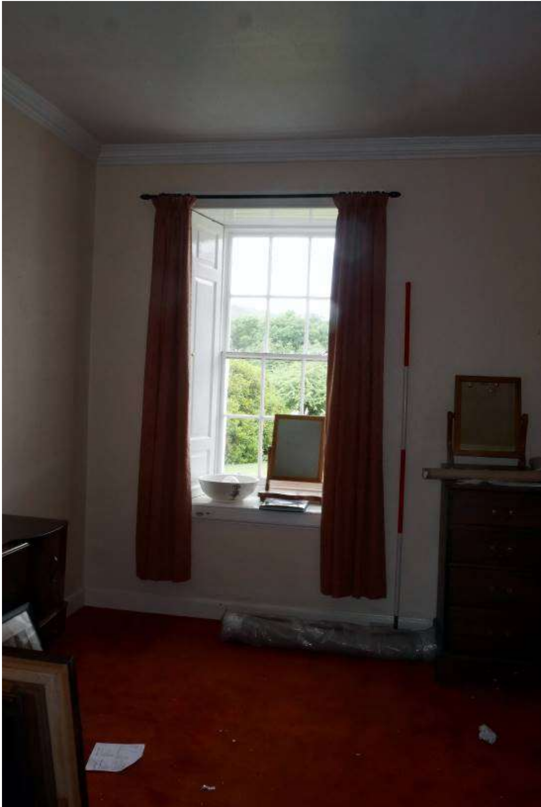
Illustration 48- Glazed shuttered window at Southern end of North Eastern internal elevation of Room (4).
