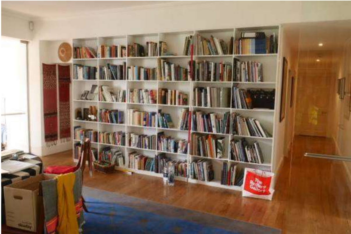
Illustration 72- South Eastern facing internal elevation of Room 10 showing bookcase and doorways. It is proposed to block the two doorways, split the bookcases left and right and form a new opening in the centre through to the new larger dining room. The corridor on the right will be incorporated into the dining room.
