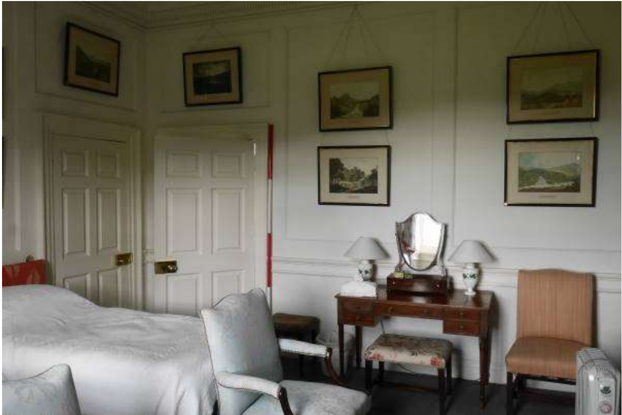
Illustration 102- Bedroom 21 South Western internal elevation showing door into First floor corridor (door to left is to be blocked).
