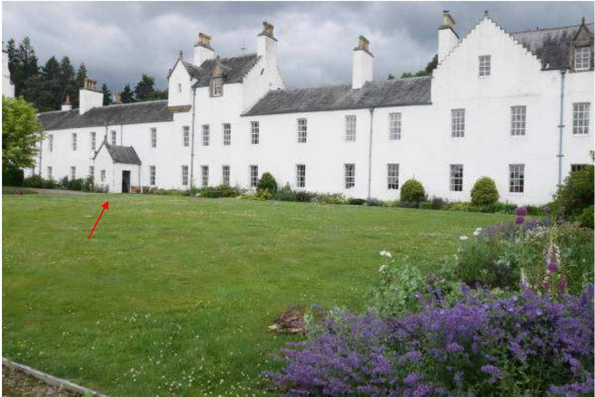
Illustration 32- South Wing looking North East. A small extension is proposed for the front of the porch extension (red arrow).
