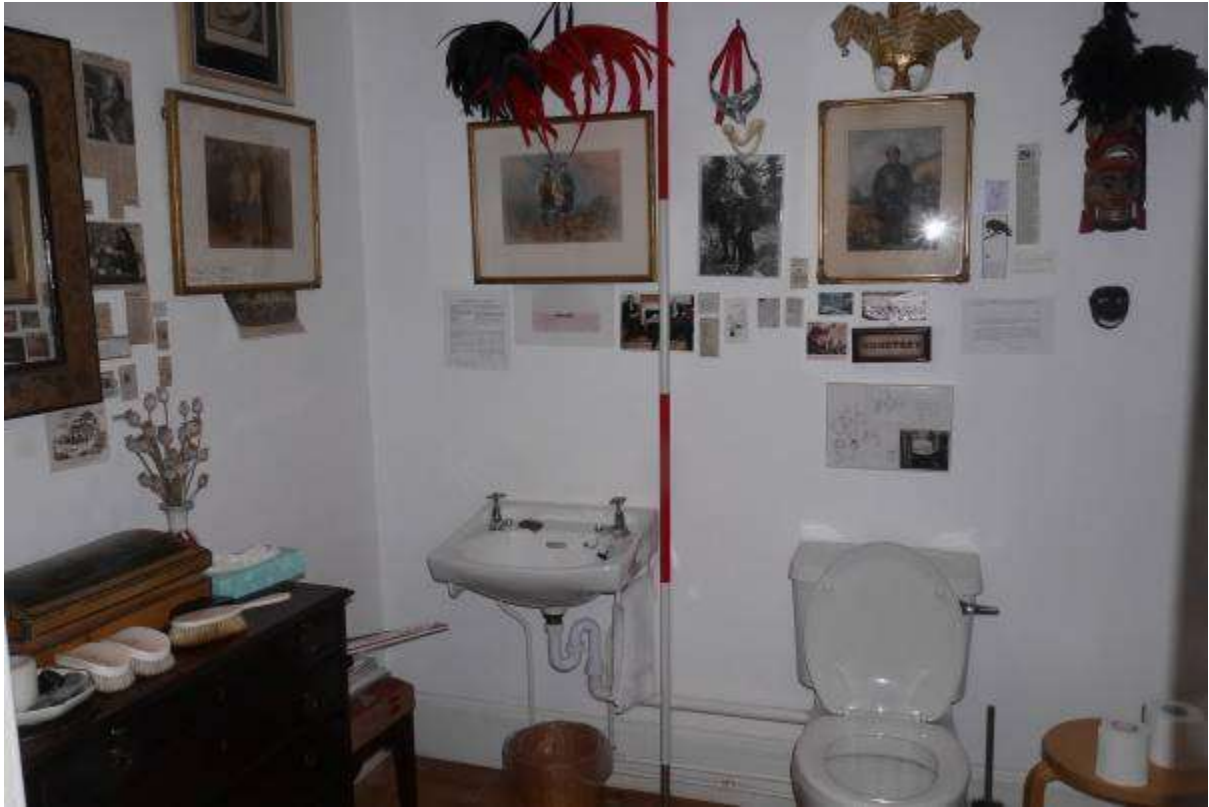
Illustration 78- South Eastern facing internal elevation of Room 12 (Lavatory). This room is to be incorporated into the main dining room once more, a new doorway to the hall will be formed at the junction of this wall and the wall on the left.
