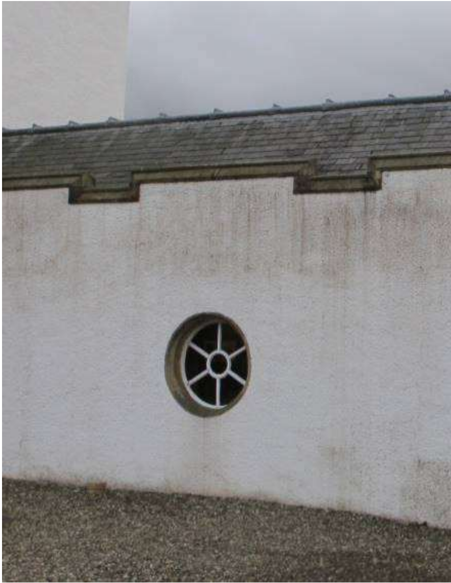
Illustration 10- Bulls Eye window on ground floor of Castle "Well Court" screen wall © JGA.
