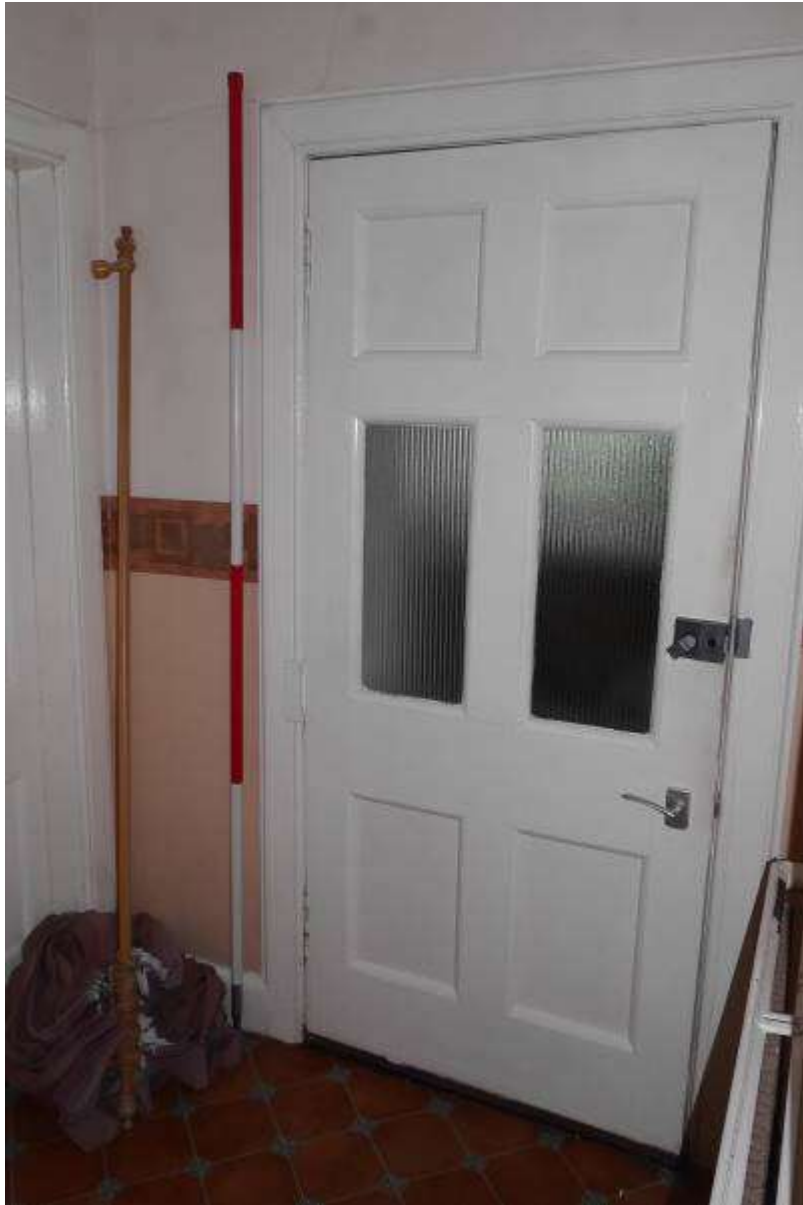
Illustration 38- Room 2 North Eastern facing internal elevation.
