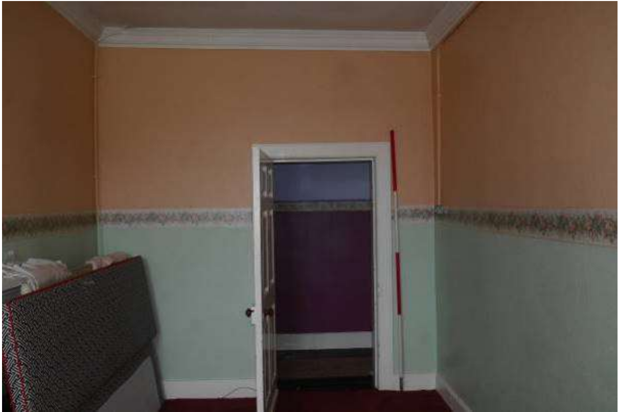
Illustration 59- Internal South Western facing elevation of Room 6 (Bedroom) showing door into South Corridor (4). It is proposed to make alterations to this elevation, the door and wall will be removed from door head level downwards.
