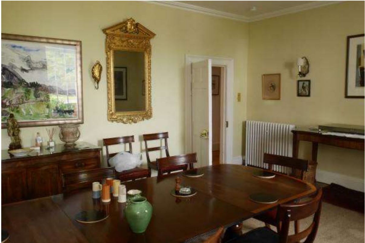
Illustration 82- South Western facing internal elevation of Room 13 (Dining Room) showing doorway into corridor. This entire wall and door are to be removed and the corridor incorporated back into the room (it was originally one larger space with a lower floor, the main Kitchen).
