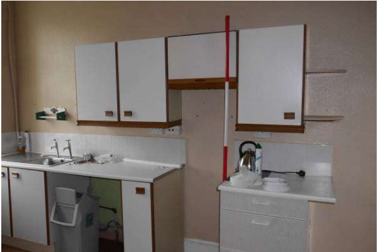
Illustration 54- Internal South Eastern facing elevation of Room 5 (Kitchen). It is proposed to remove the furniture.
