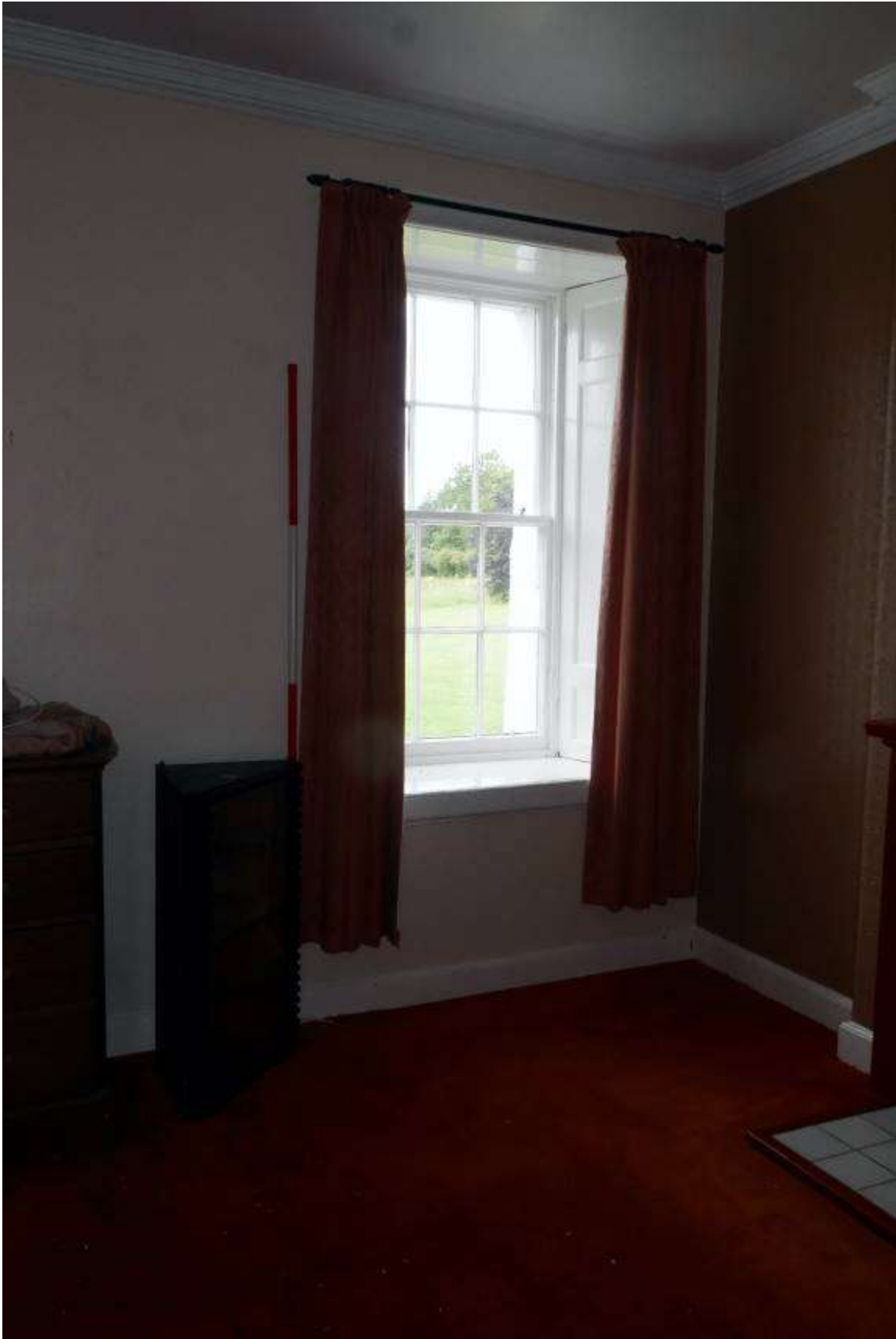
Illustration 49- Glazed shuttered window at Northern end of North Eastern facing internal elevation of Room 4. It is proposed to make alterations to this elevation.
