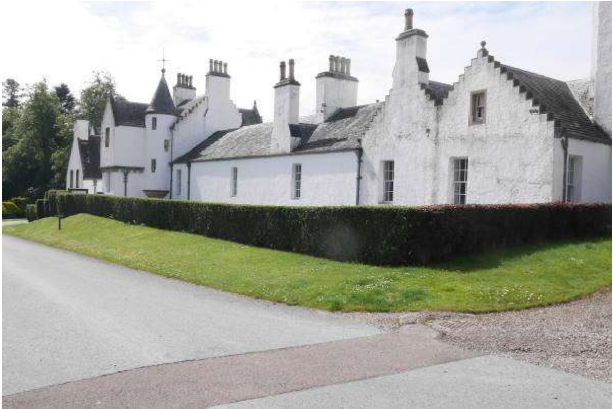
Illustration 31- South Wing looking South West.
