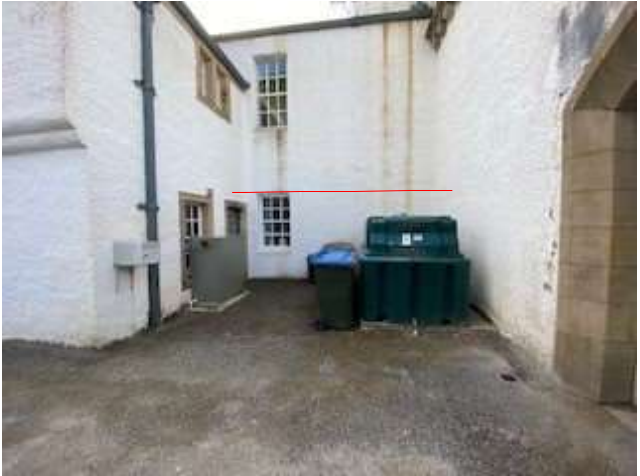
Illustration 122- General view of line of new ground floor corridor (red line). See Illustrations 123 and 125 for detailed views of either end.
