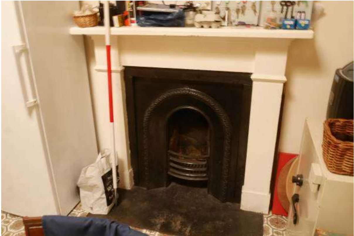
Illustration 88- Detail of fireplace in North eastern facing internal elevation of Room 15 (Pantry).
