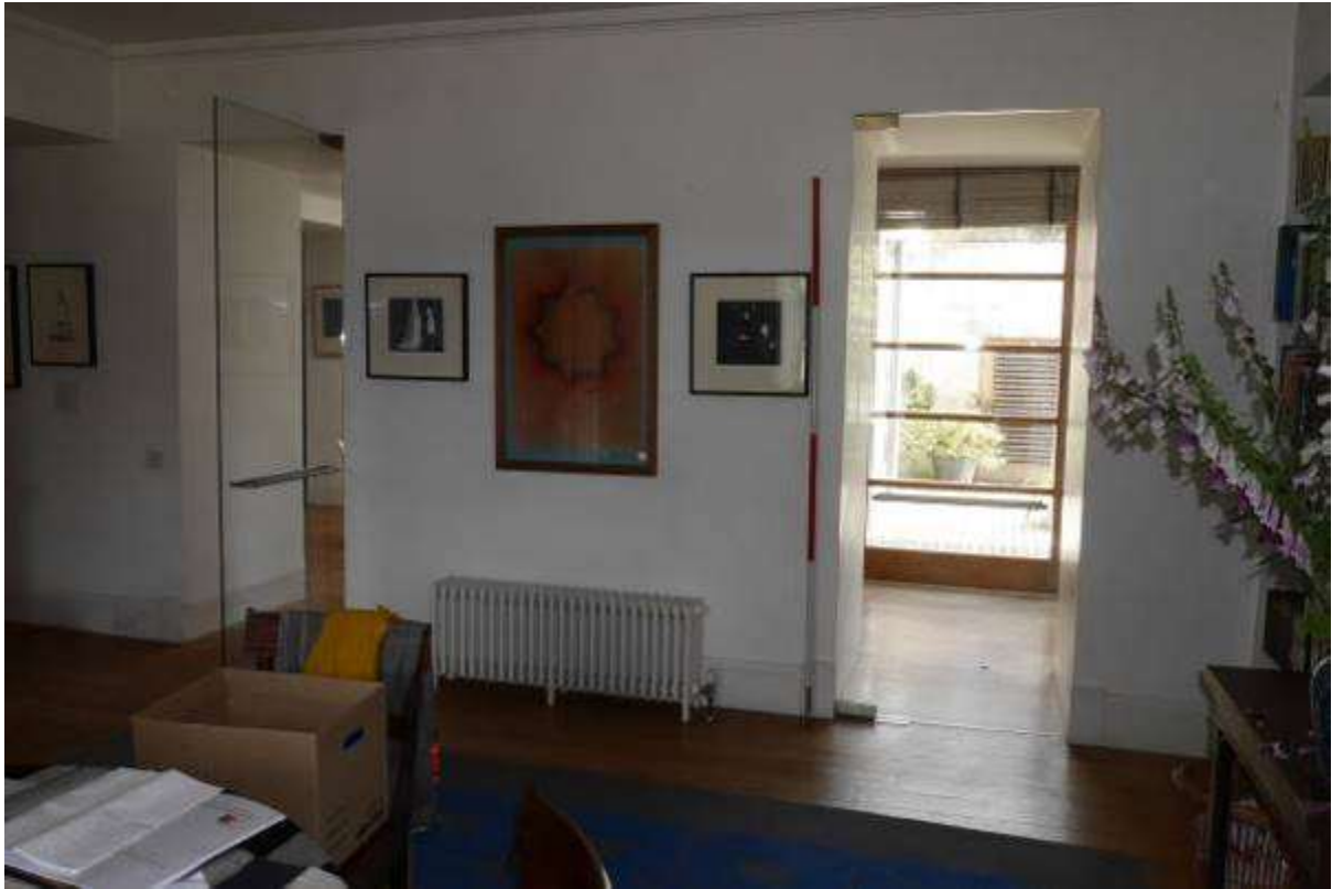
Illustration 75- South Western facing internal elevation of Room 10 showing Doorway (9) and doorway into Kitchen (14).
