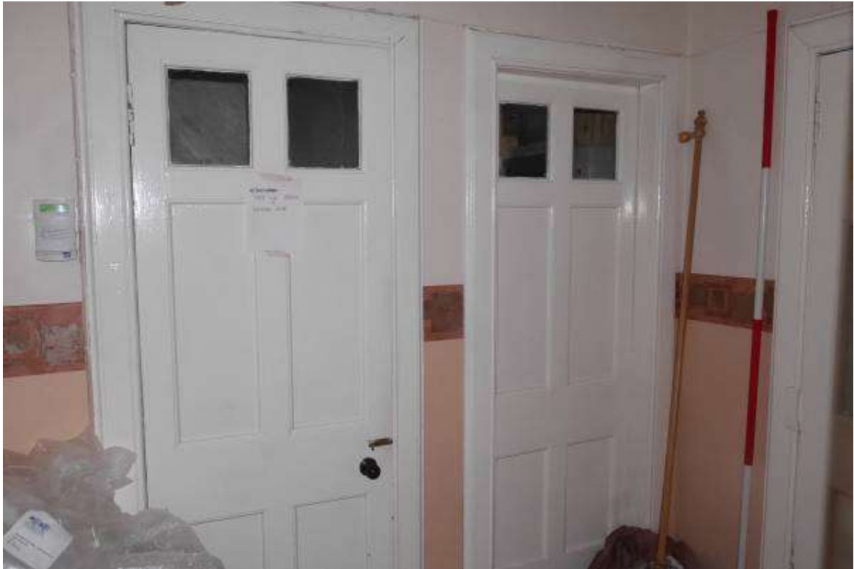
Illustration 41- North Western facing internal elevation. It is proposed to remove this dividing wall to make space for the new stair.
