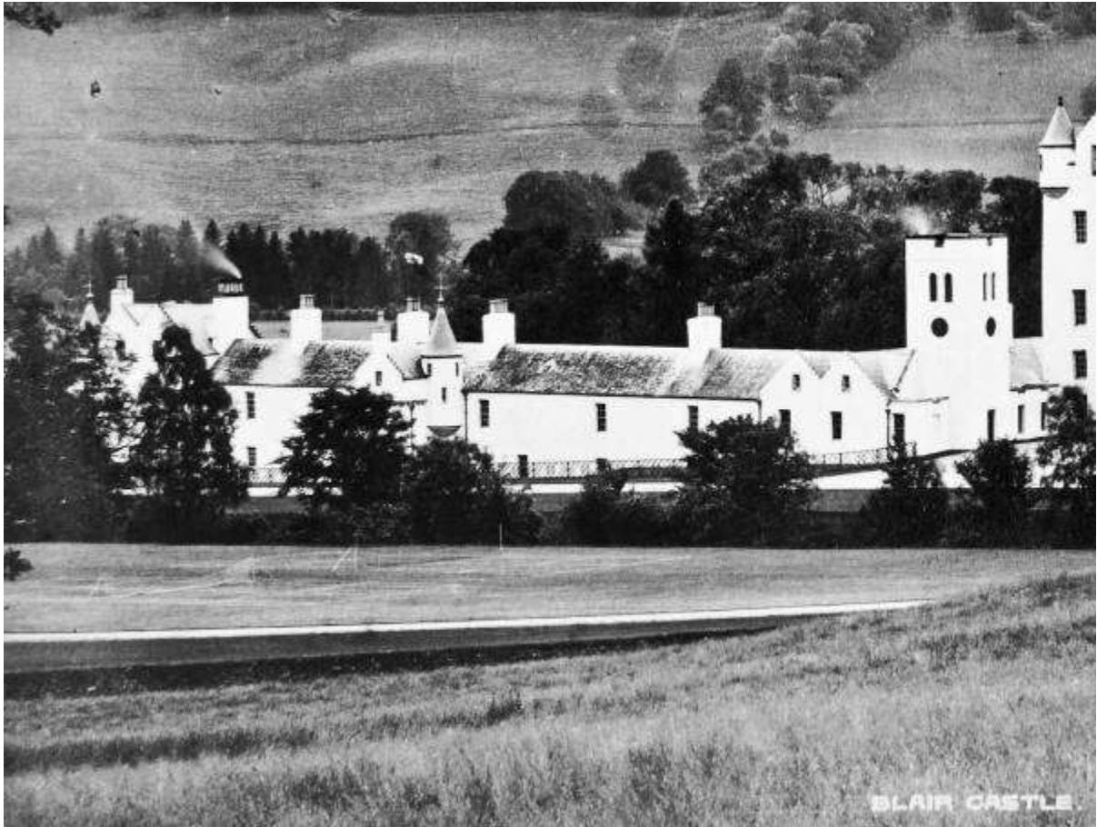
Illustration- 12 Blair Castle 1885 George Washington Wilson, (cropped) view of South Wing East side. This view includes the extended stair tower in the centre of the wing's west side, but not an extra floor over the whole wing width. The chimneys are the same height as the originals and there is no gabled "but & ben" between them. Courtesy: BCA.
