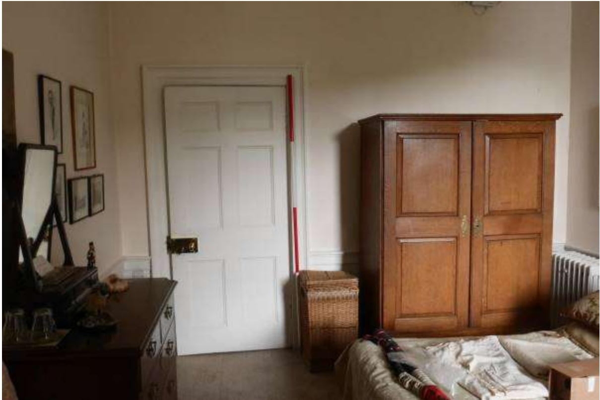
Illustration 115- Bedroom 25 South Western internal elevation, it is proposed to block the doorway.
