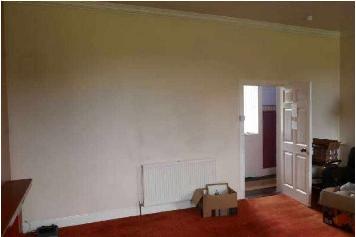
Illustration 51- Internal South Western facing internal elevation of Room 4.
