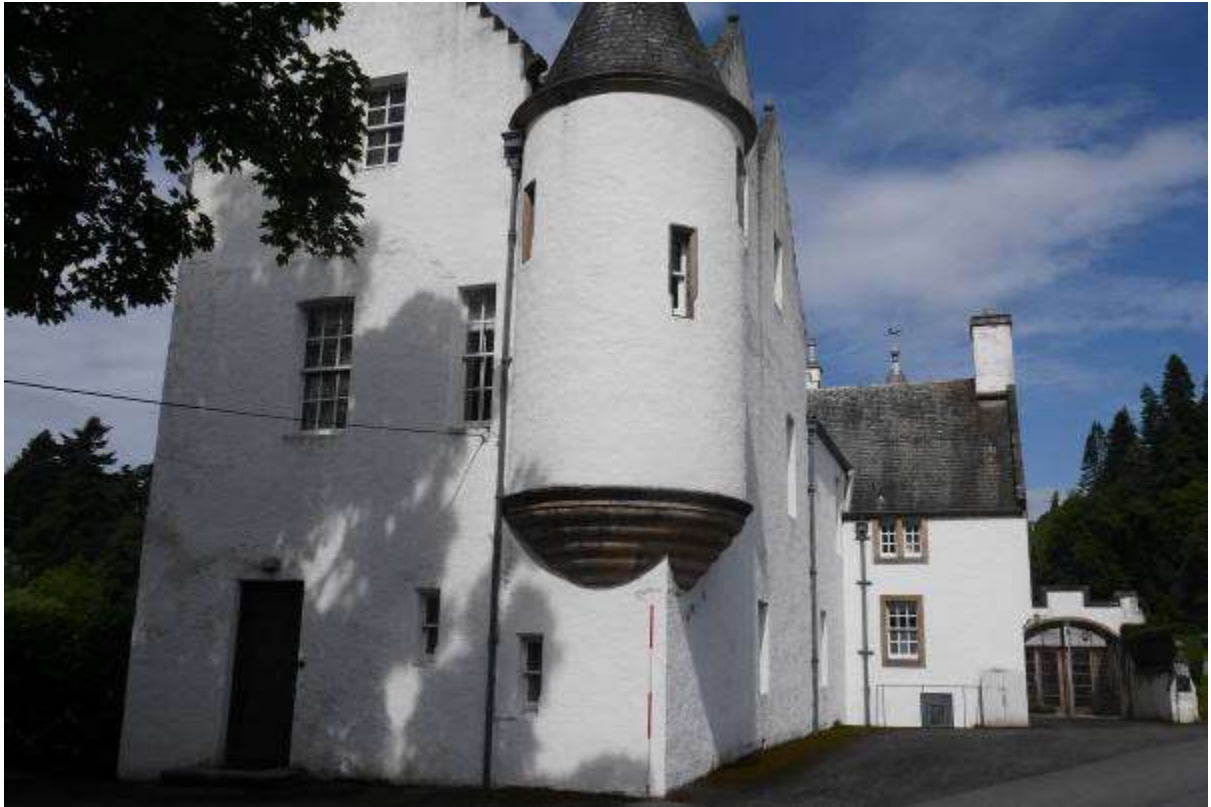
Illustration 30- South Wing looking North.
