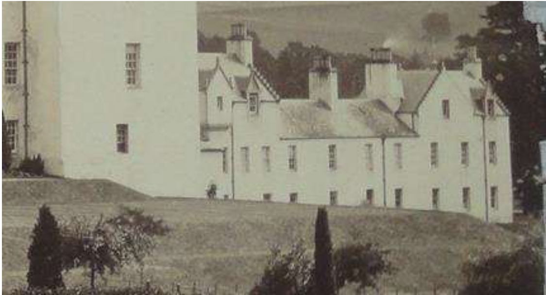
Illustration 13- Blair Castle 1893 cropped view of South Wing West side taken from North side of the Castle. Walker's "but & ben" addition is built, and the windows have been added on the ground floor BCA.
