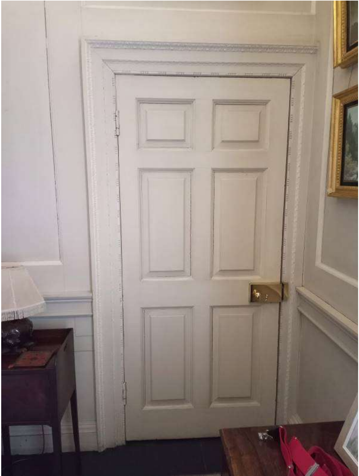
Illustration 107- Doorway 23 in Bedroom F10. This doorway is to be blocked.
