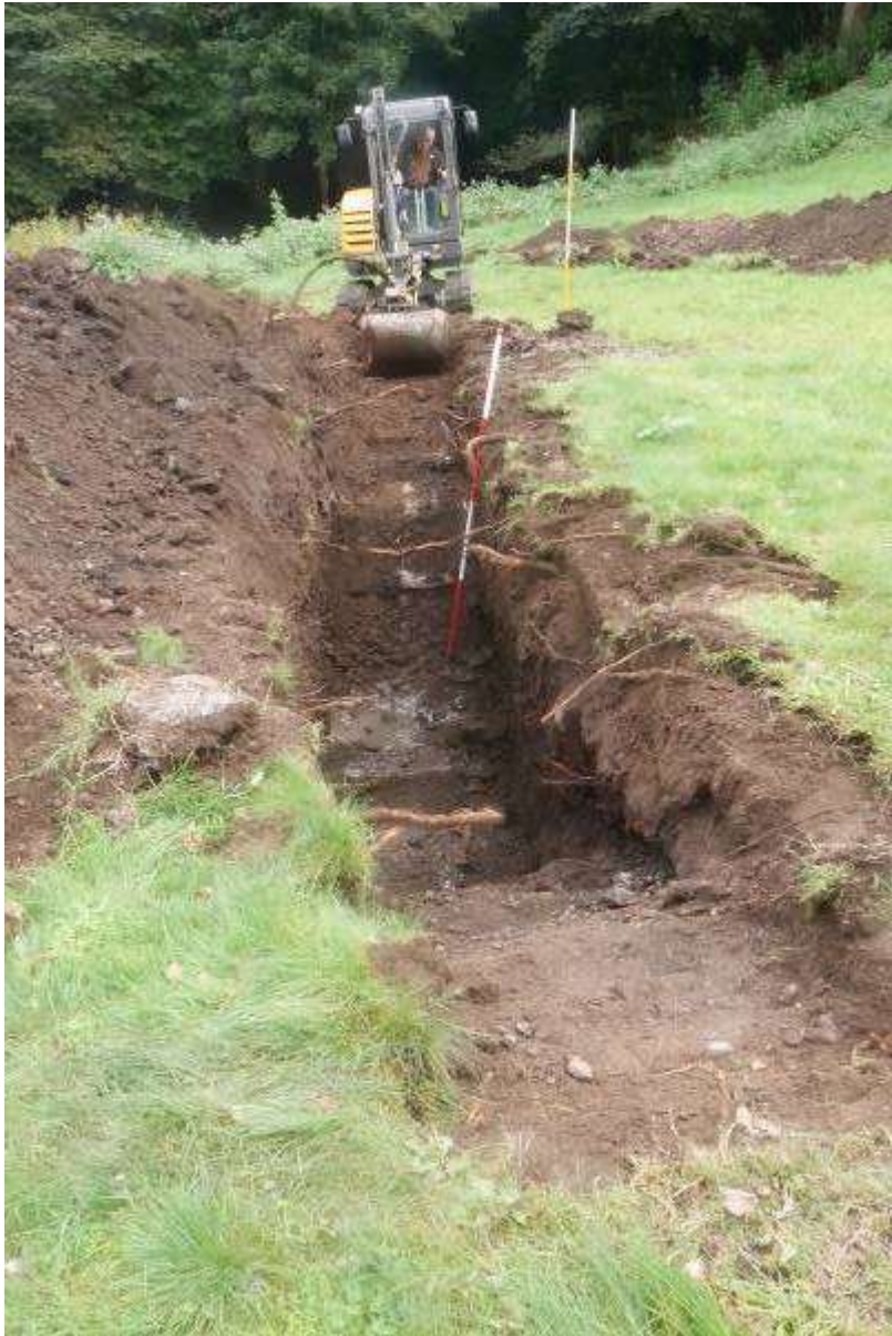
Illustration 13- Trench C under excavation looking South East, ranging rod is in deep modern soakaway.
