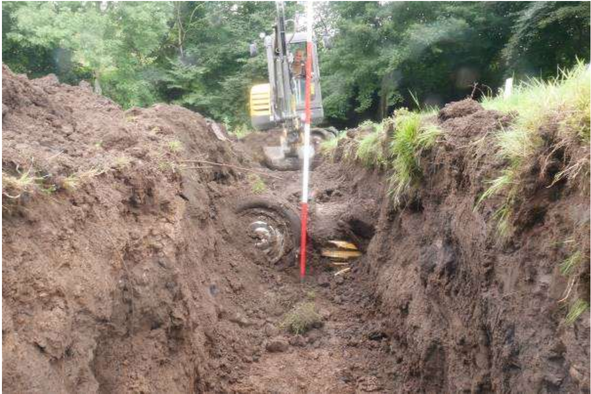
Illustration 10- Dumped Wolseley car becoming visible in Trench B.
