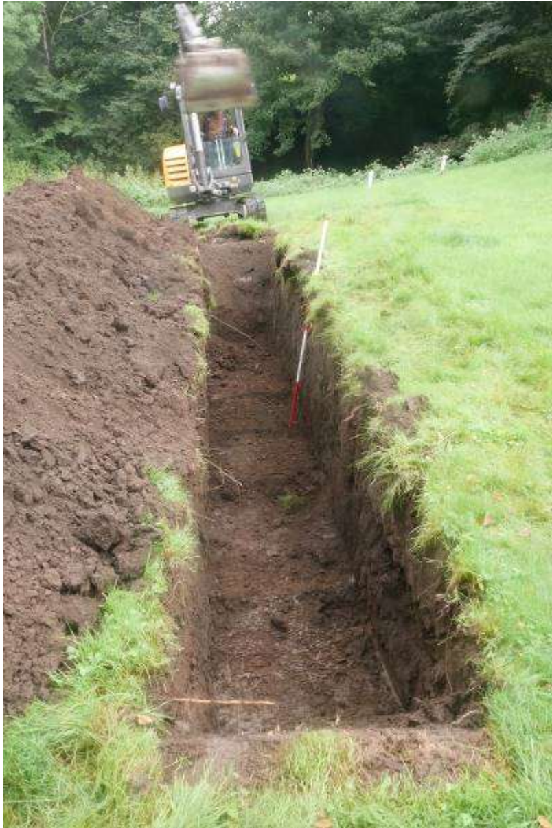
Illustration 8- Trench B under excavation looking North East.
