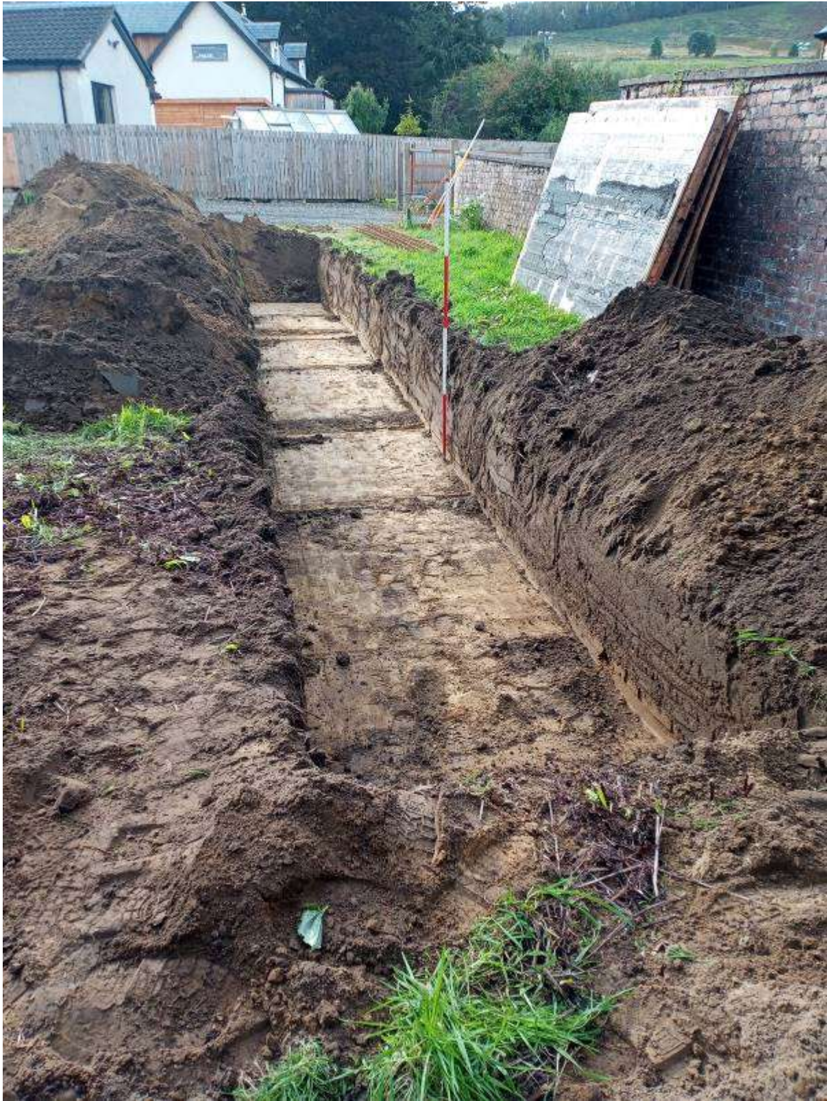
Illustration 10- Trench B completely excavated looking South showing moderate light-yellow sand 201 below dark down sandy clay 200.
