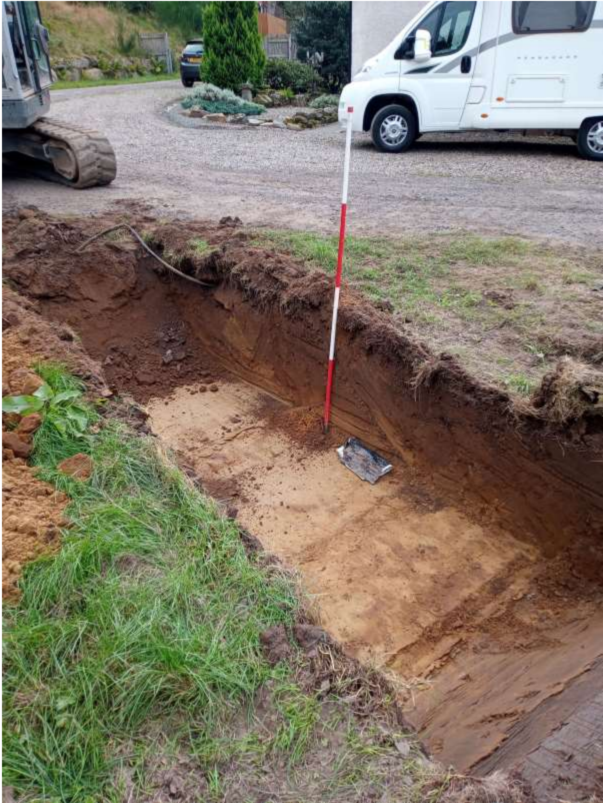
Illustration 13- Trench C completely excavated looking South showing dark brown sandy clay 300 overlying moderate natural light-yellow sand 301.
