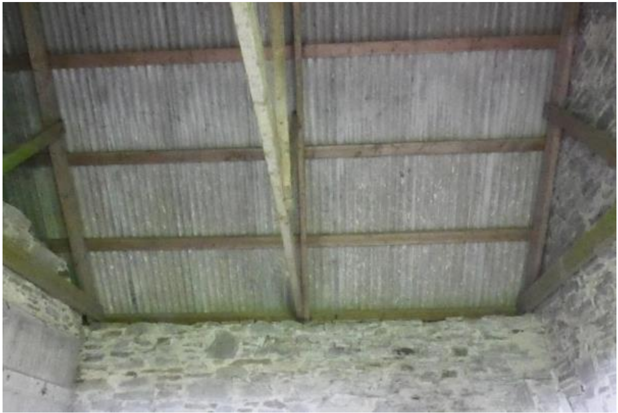
Illustration 19 – Internal view of corrugated iron roof of Building A.
