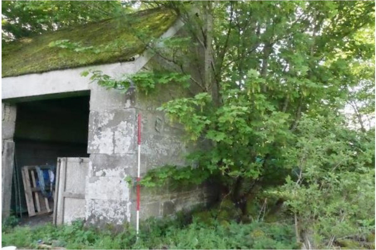
Illustration 14- North Western facing external elevation (gable) of Building A.
