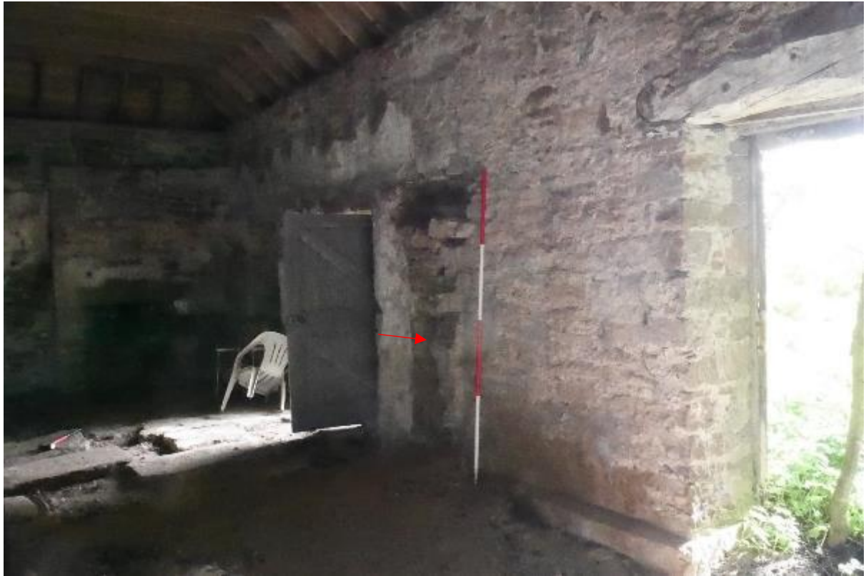
Illustration 46 – General view of internal North Western facing elevation of Building B, red arrow former wall line of earlier building as in opposing elevation (Illus 42).
