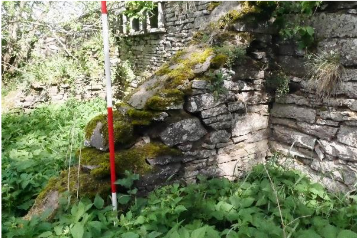
Illustration 53- Detail view of one of the buttresses built against the South Western facing elevation of Boundary wall C.
