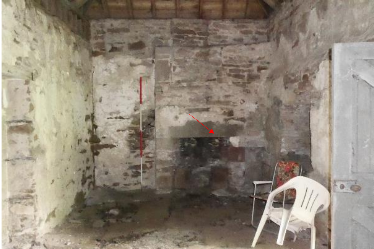
Illustration 44 – General view of internal South Western facing elevation of Building B, fireplace and cupboard at red arrow.
