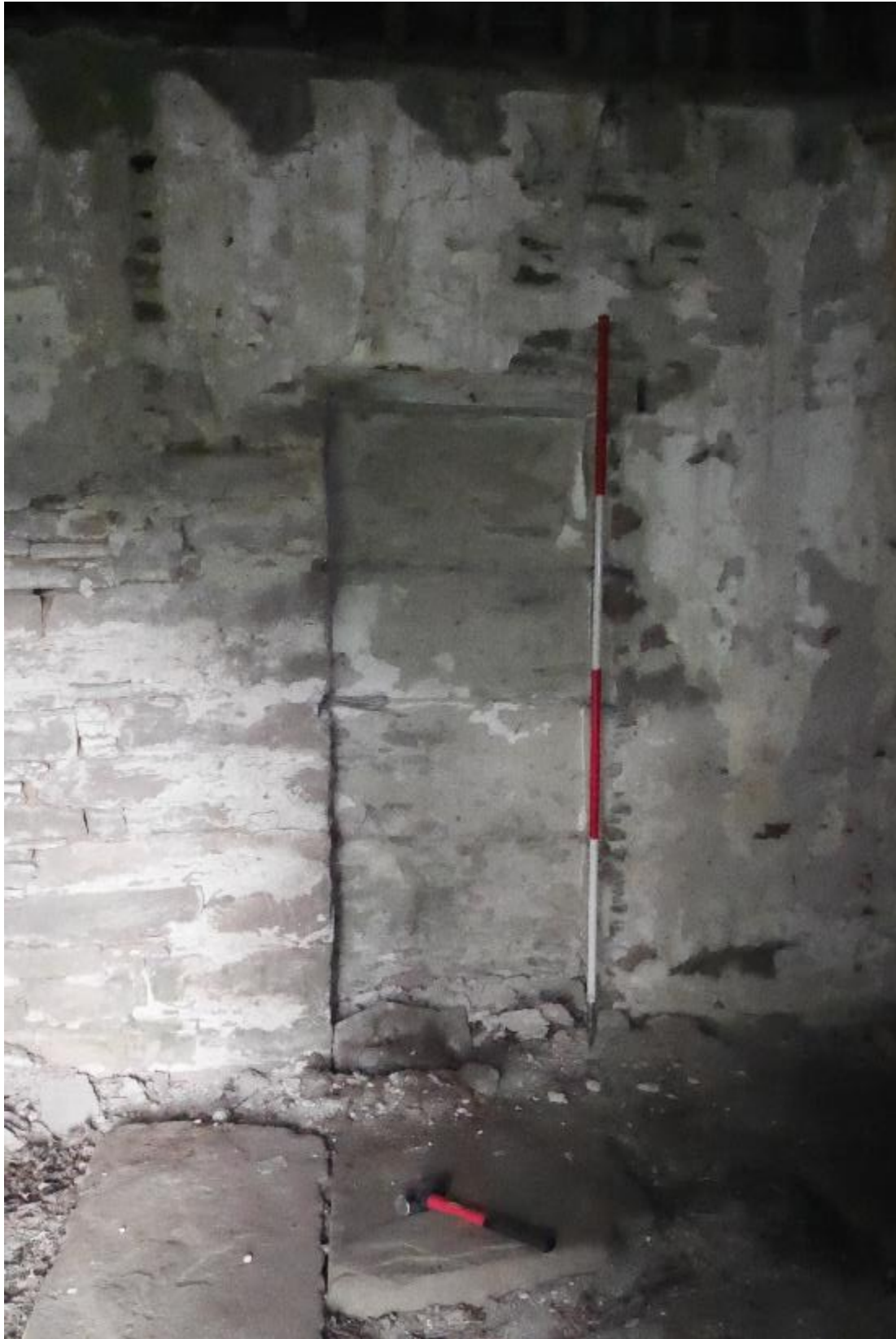
Illustration 41 – Blocked doorway in internal South Eastern facing elevation of Building B.
