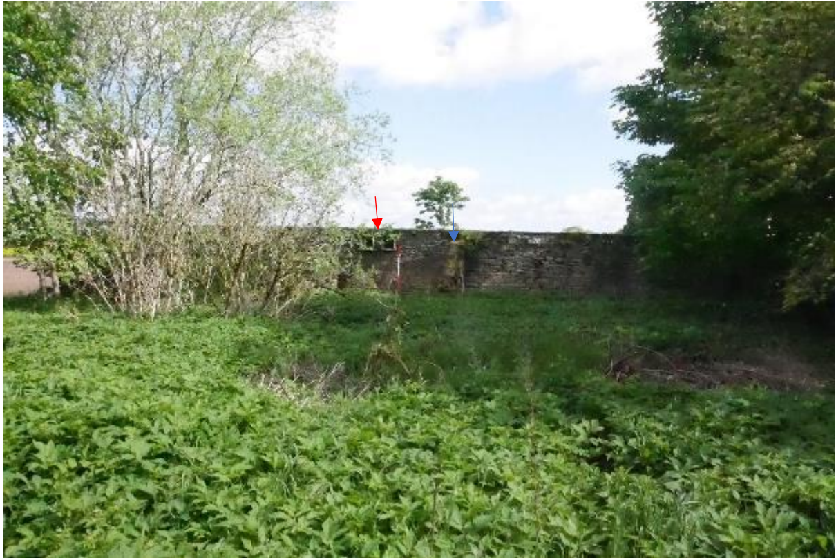
Illustration 50- General view of Boundary wall C looking North, red arrow shows location of bird boxes (see Illus 51), and blue arrow shows one of four buttresses built against wall face (see Illus 51 and 53).
