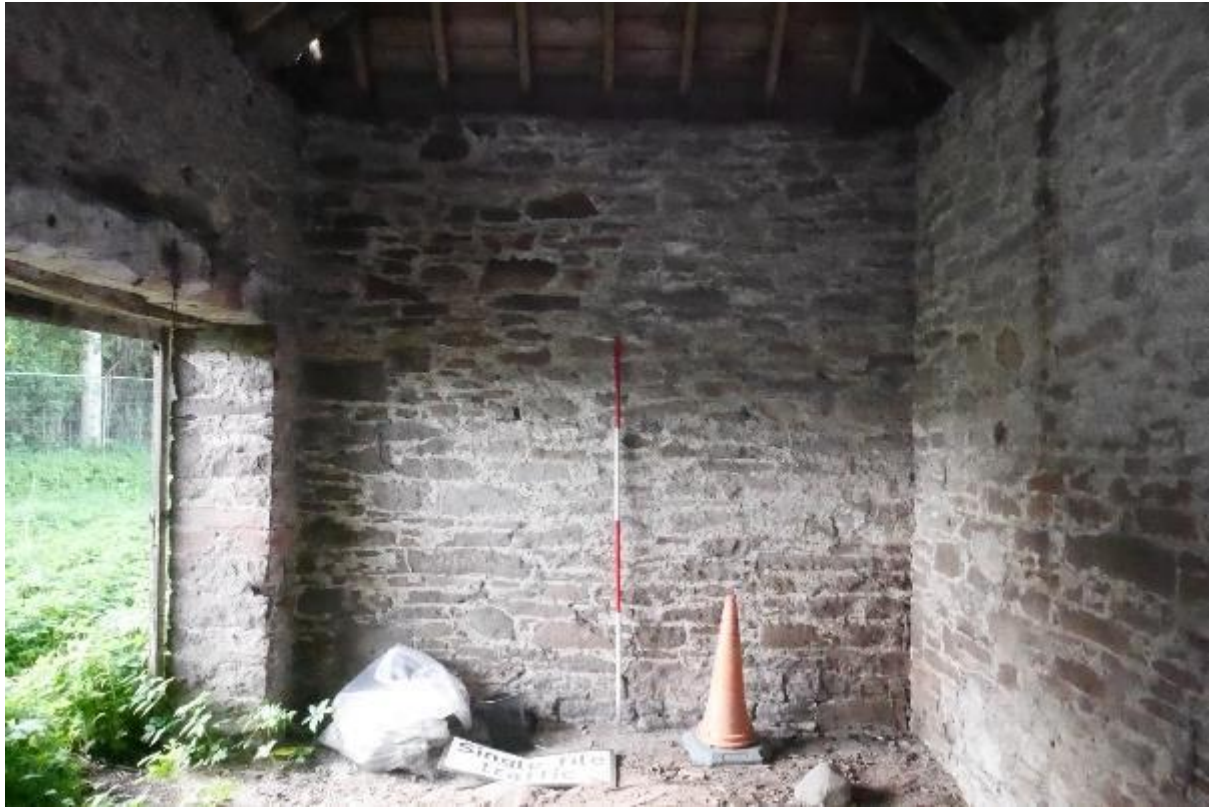
Illustration 49 – General view of internal North Eastern facing elevation of Building B.
