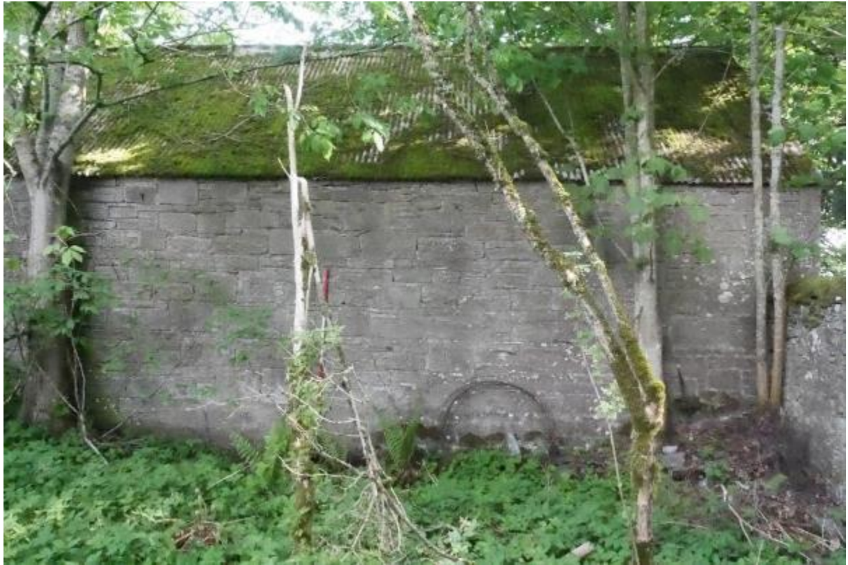
Illustration 15- South Western facing external elevation of Building A.
